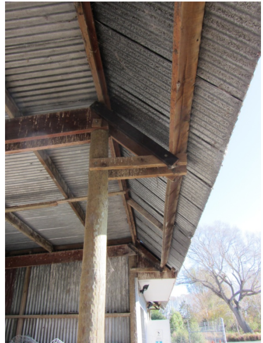
Photo 4: Structure along The Eastern Face
