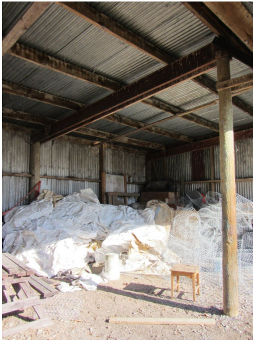
Photo 3: Internal View of Structure
