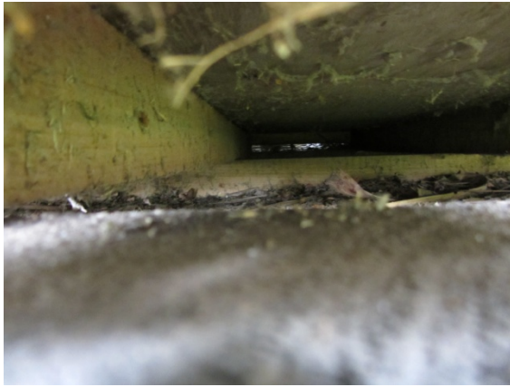
Photo 5: Underside of the building showing the timber bearers 2 of 2
