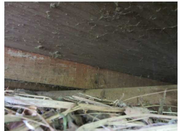
Photo 4: Underside of the building showing the timber bearers 1 of 2
