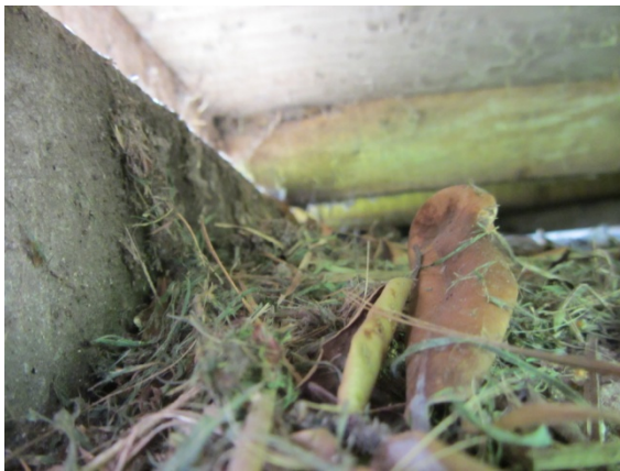
Photo 3: Underside of the building
