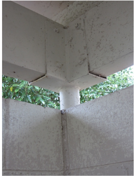
Photo 6: Interior view of steel connection
