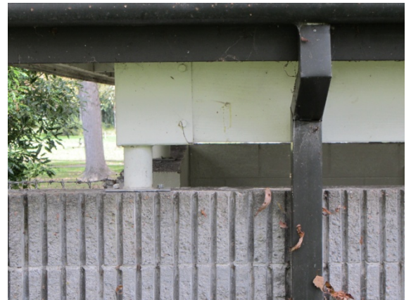
Photo 4: Exterior view of south west steel connection
