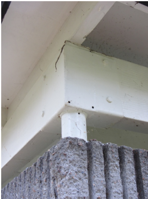
Photo 7: exterior view of connection
