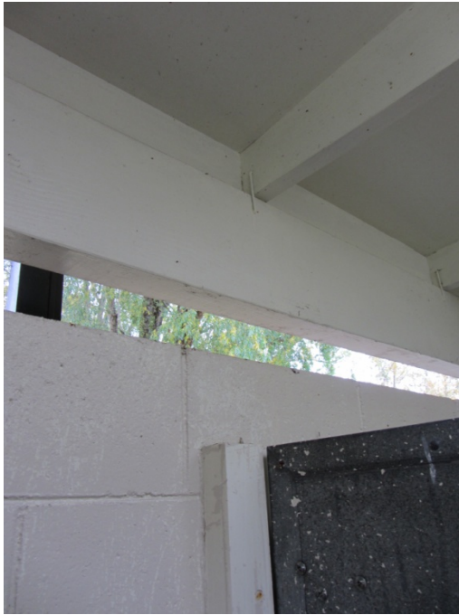
Photo 5: Interior view of timber roof frame
