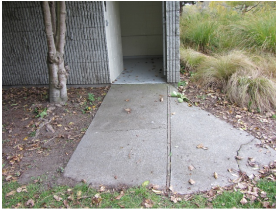
Photo 13: Pavement leading to womens toilet
