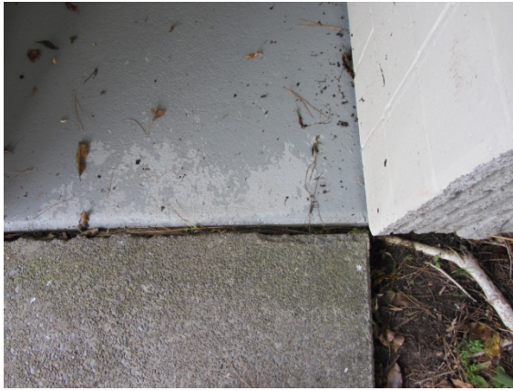
Photo 21: Separation between pavement and entrance to mens toilet
