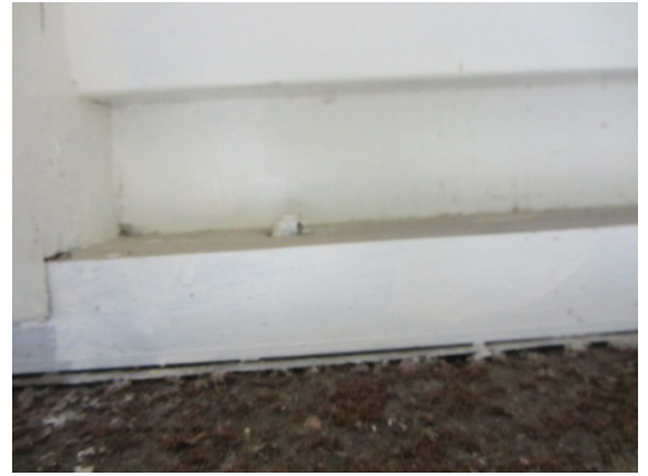
Photo 10: Bolt connection between timber and masonry
