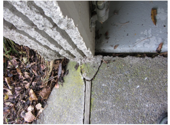
Photo 22: Cracking in the pavement at the mens toilet entrance
