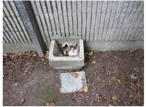
Photo 18: Sump at the back of the toilet block (west side)
