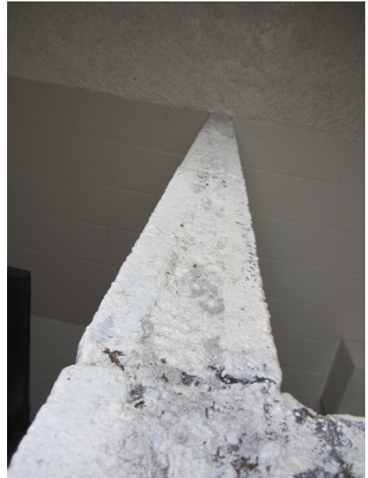
Photo 8: top of the wall showing infilled masonry blocks
