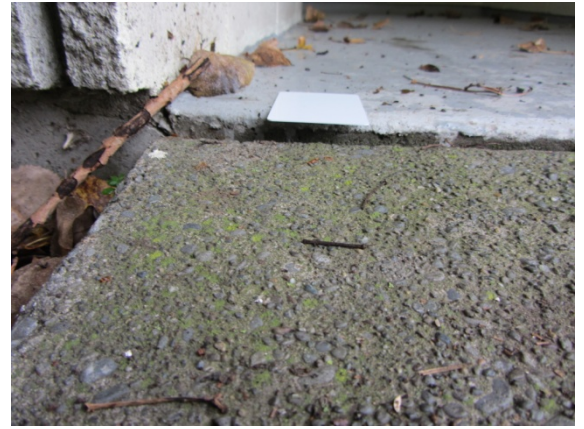
Photo 14: Separation between pavement and toilet entrance
