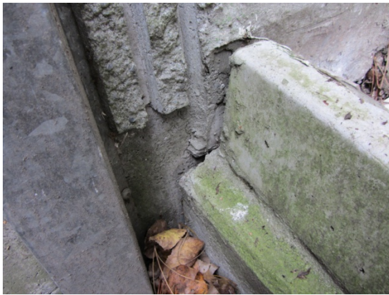
Photo 19: Separation between sump and toilet structure
