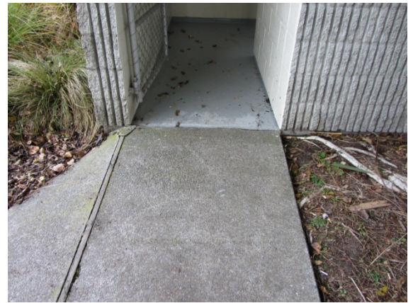
Photo 20: Pavement leading to the mens toilet
