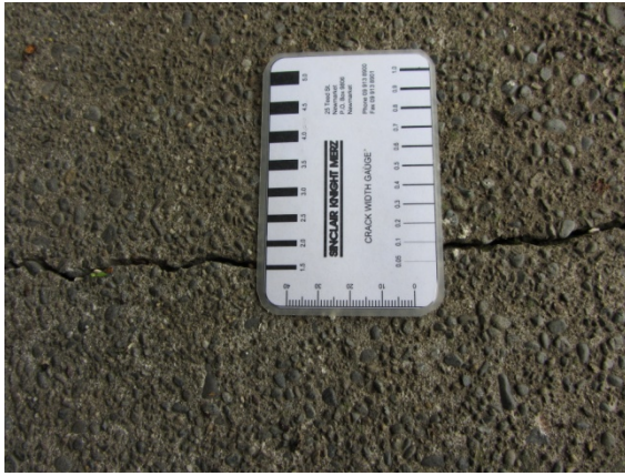
Photo 17: Close up view of crack from photo 16 showing 1.5mm wide crack
