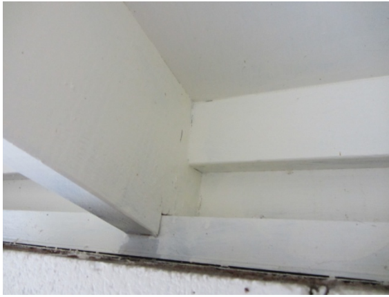
Photo 9: Rafter connection
