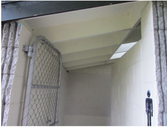
Photo 5: Entrance to mens toilets
