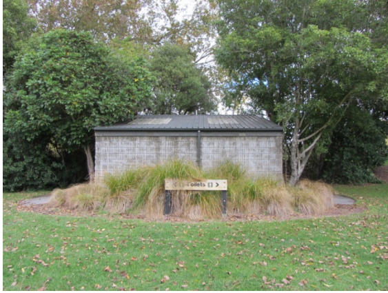
Photo 1: East elevation, with womens toilet on the left and mens toilet in the right
