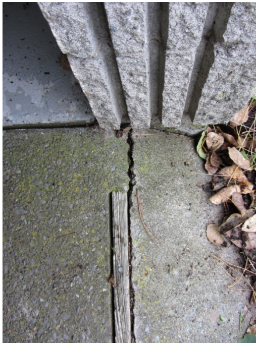
Photo 15: Cracking in the pavement
