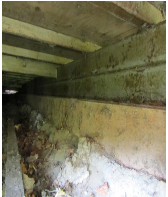
Photo 8: Underside of Building – Photo 4
