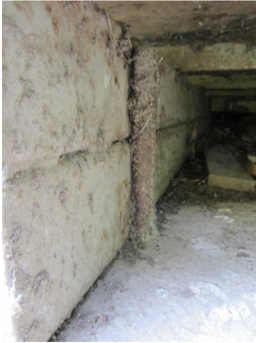
Photo 5: Underside of Building – Photo 1
