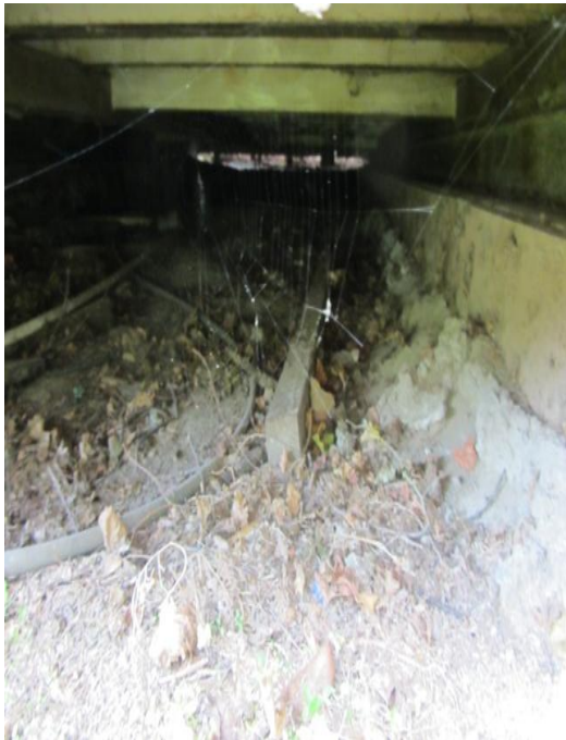
Photo 7: Underside of Building – Photo 3
