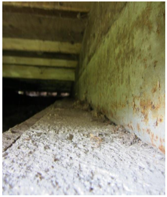
Photo 6: Underside of Building – Photo 2
