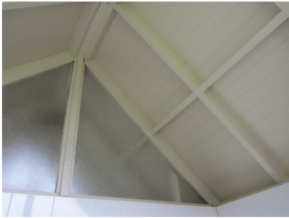
Photo 5: Interior view of roof (2 of 2)
