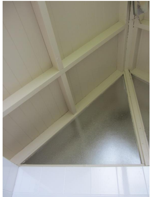
Photo 4: Interior view of roof (1 of 2)
