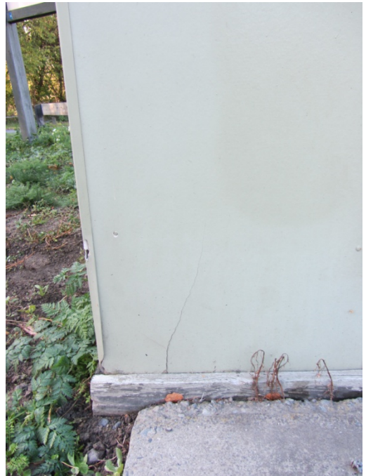
Photo 8: Cracking to Cladding Panel in NE Corner
