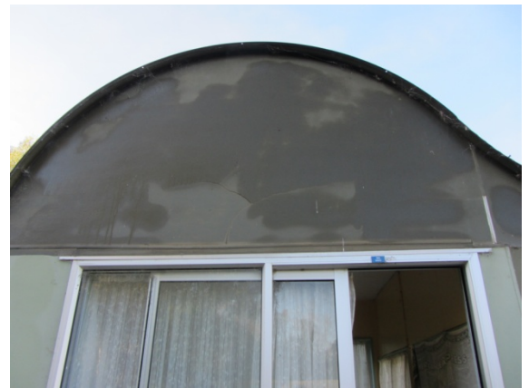
Photo 4: Damage to Cladding above North Door
