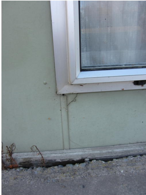
Photo 9: Hairline Cracking to Cladding Panel under North Door
