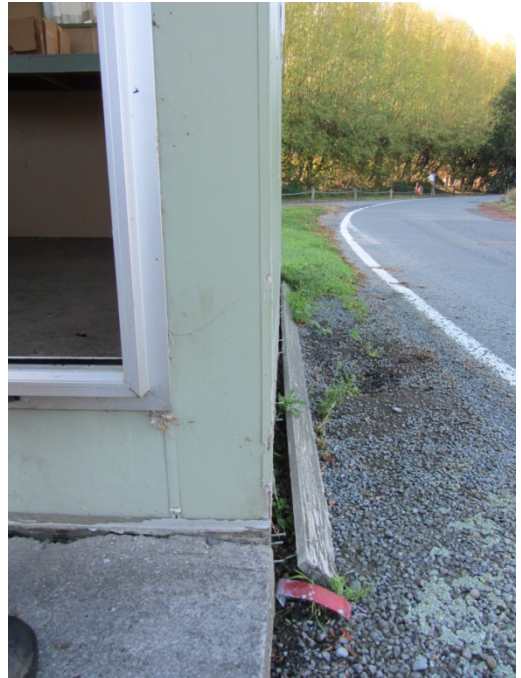
Photo 10: Hairline Cracking to Cladding Panel in NW Corner
