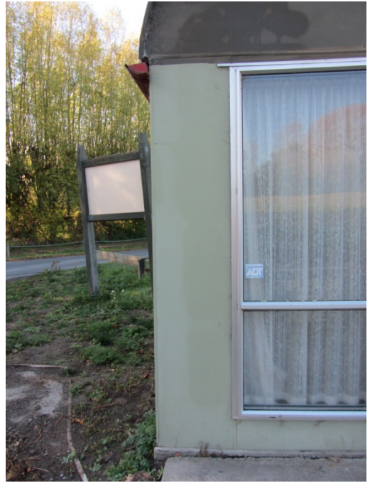
Photo 6: Hairline Cracking to Cladding on the North Wall
