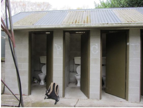
Photo 1: North elevation 1 of 2
