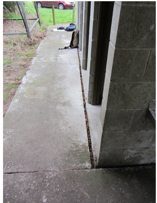
Photo 12: Pavement in front of the toilet block showing the separation away from the structure.
