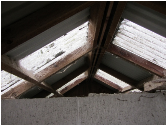
Photo 7: Interior view along the apex of the roof
