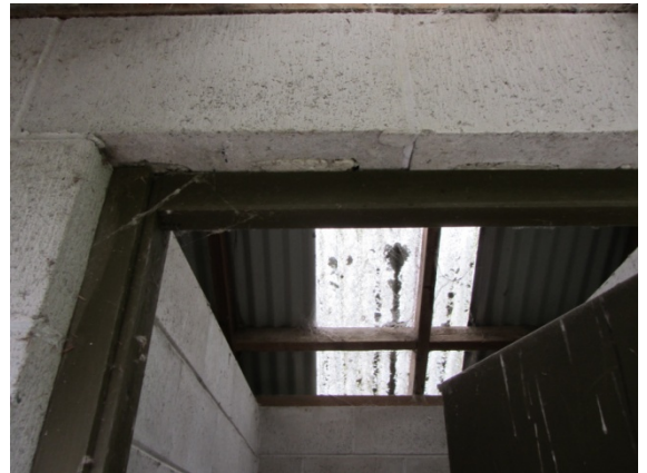
Photo 8: Bond Beam above doorway
