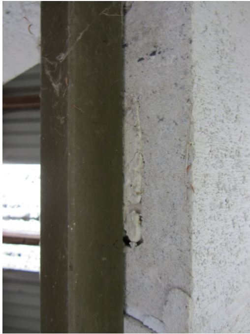
Photo 9: Side of the door way
