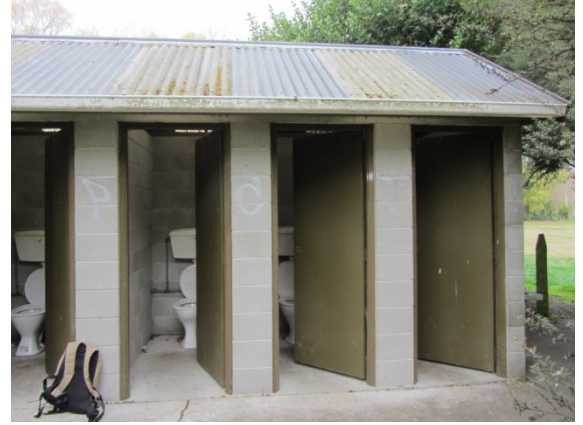
Photo 2: North elevation 2 of 2
