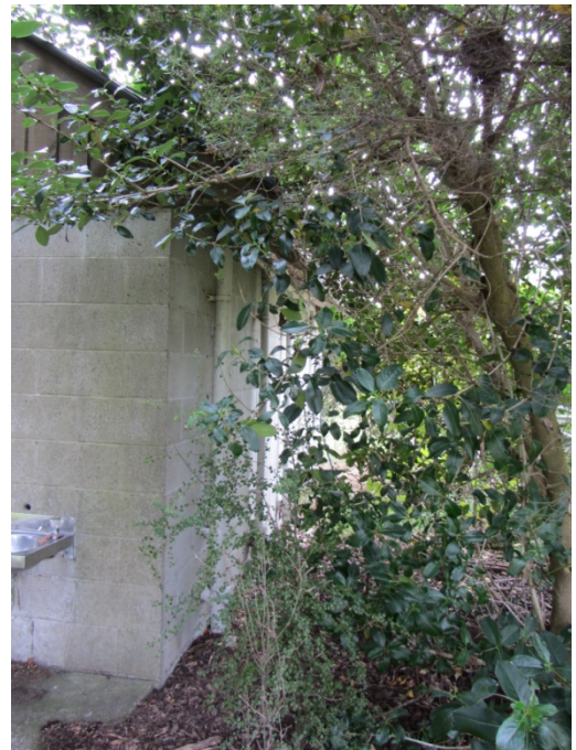
Photo 4: View towards south elevation
