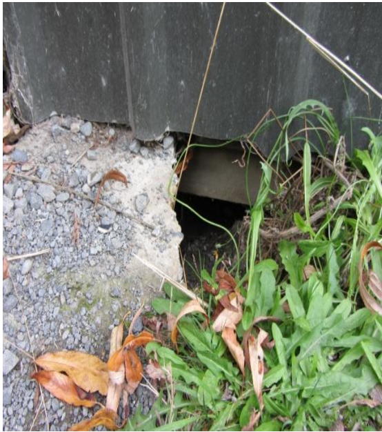
Photo 5: View of timber framed foundation
