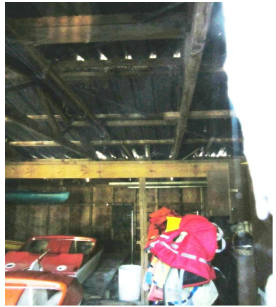
Photo 6: Interior view showing roof truss and steel bracing
