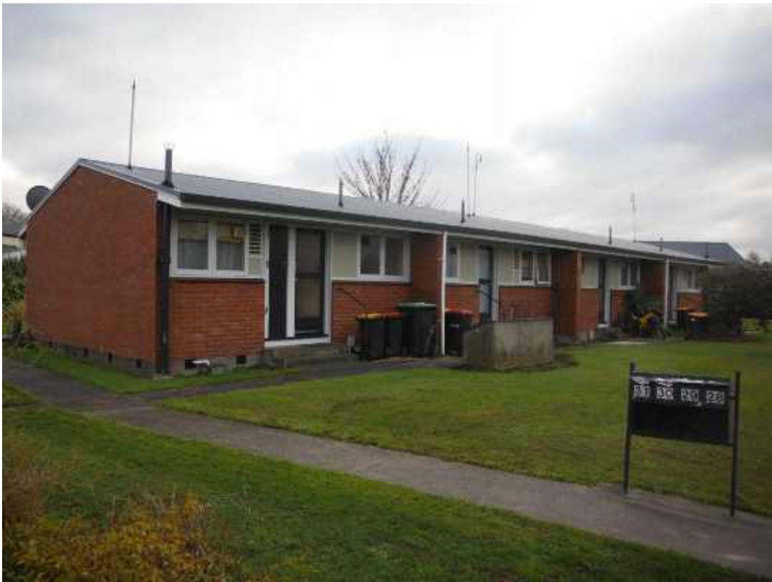
Photograph 2: Rear Elevation of Units 28 -31, Gowerton Place.
