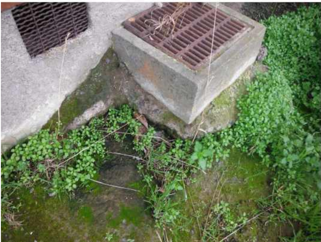
Photograph 8: View of exposed concrete observed around drain where the ground may have settled (up to 60 mm) at the southern corner of Unit 11.
