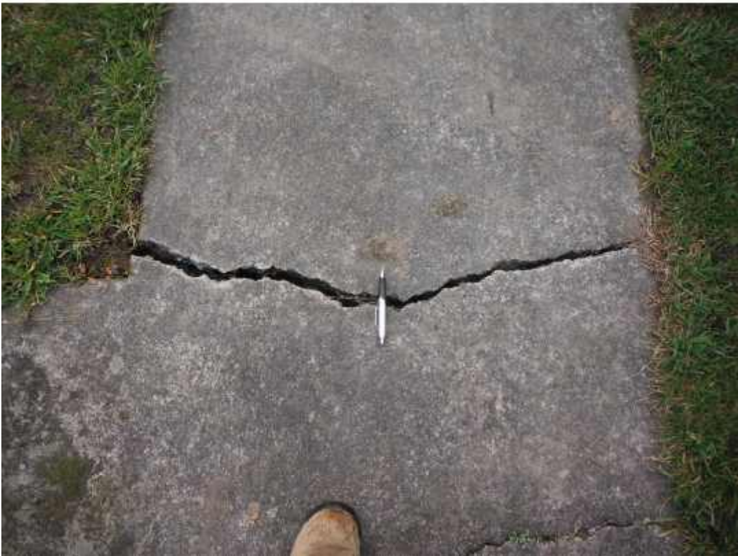
Photograph 10: View of crack (approximately 40 mm wide) across entire width of footpath slab indicating differential settlement.
