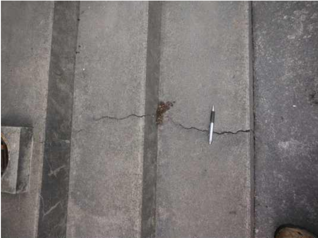
Photograph 7: View of crack (approximately 3 mm wide and 750 mm long) observed in the front porch slab of Units 11 and 12.
