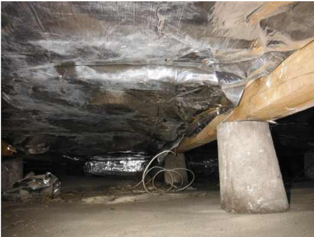
Photograph 11: View of liquefaction observed beneath floor in Unit 20.
