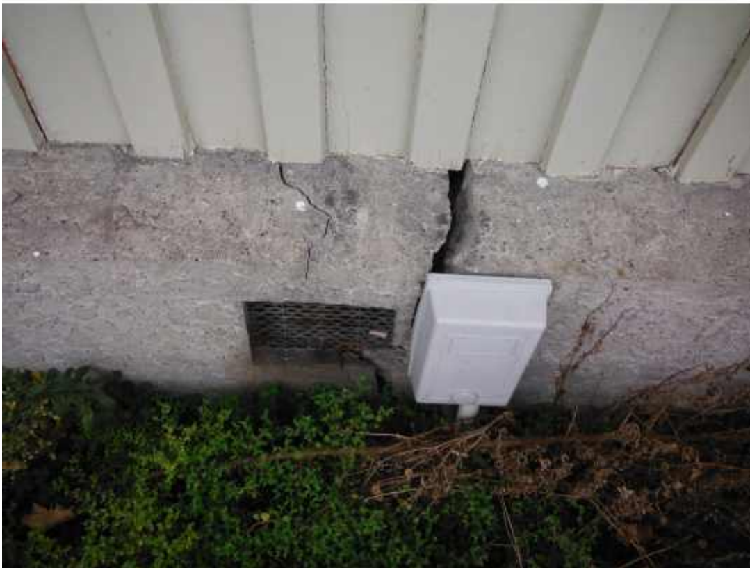
Photograph 4: Large crack (approximately 30 mm wide) observed in footing, north-western side of Unit 21.
