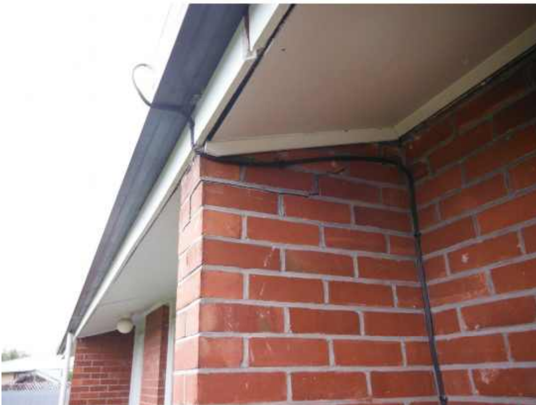
Photograph 6: View of cracking in the party walls (approximately 4 mm wide and 500 mm long) between Units 21 and 22.
