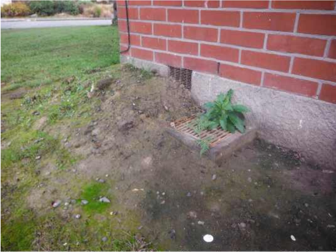
Photograph 9: View of ejected liquefied material (approximately 200 mm high) observed in the flower bed at southern corner of Unit 16.
