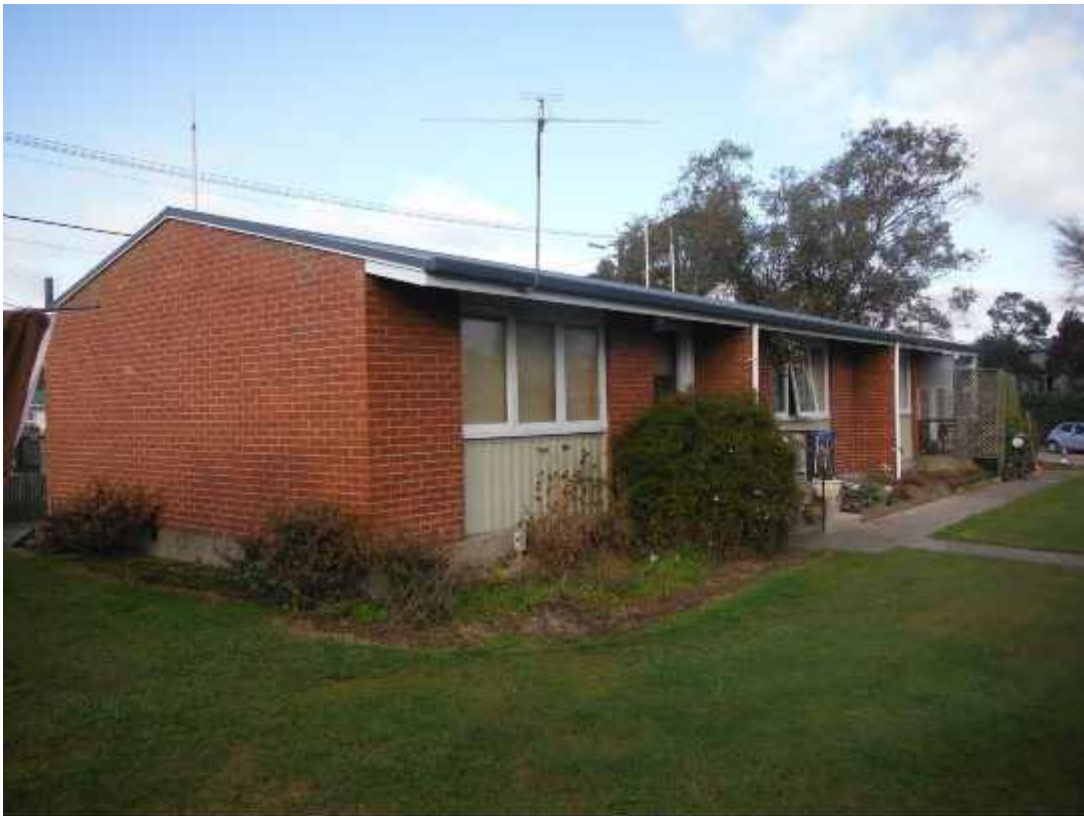
Photograph 1: Front Elevation of Units 1 -3, Gowerton Place.
