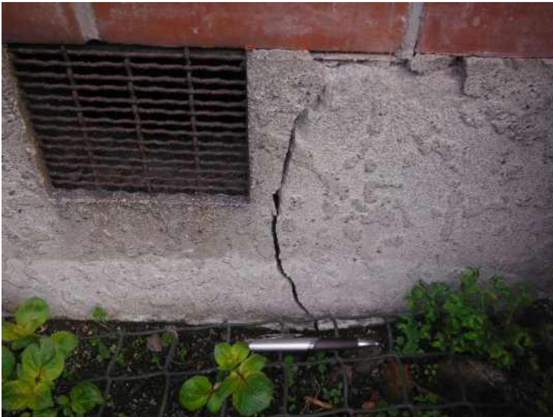
Photograph 3: Observed crack (approximately 4 mm wide) in footing, south-eastern side of Unit 18.
