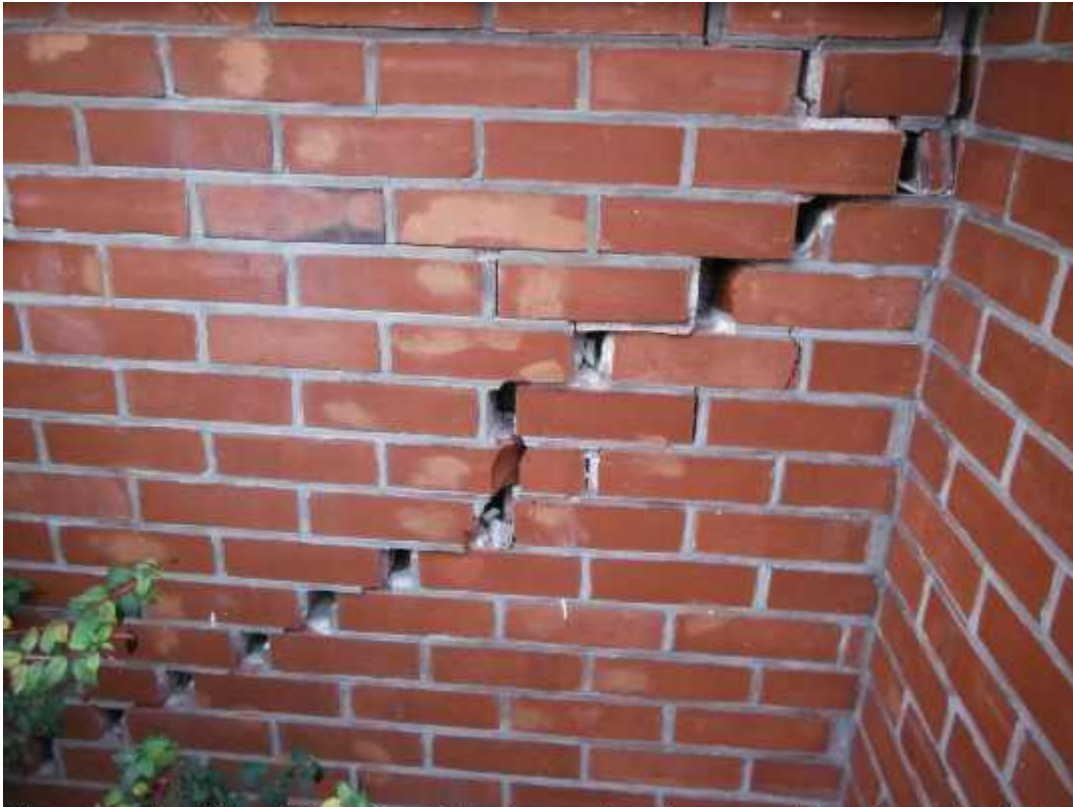
Photograph 5: View of stepped cracking (approximately 40 mm wide and 2 m long) observed in the brick veneer in the southeast corner of Unit 22.
