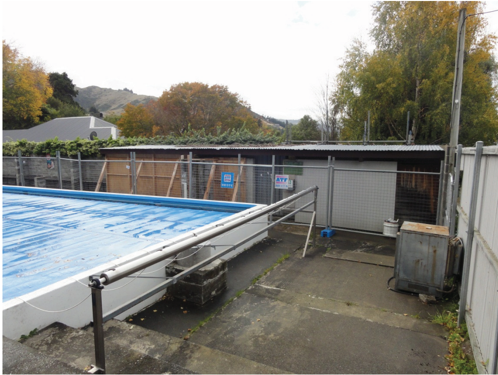
Photo 3 Extensive propping of building. Paving slabs around pool tilted.
