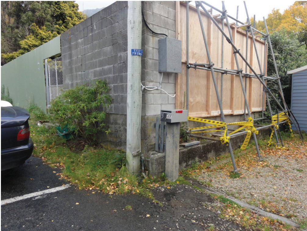
Photo 4. Blockwork on SE corner of building at back of storeroom propped.
