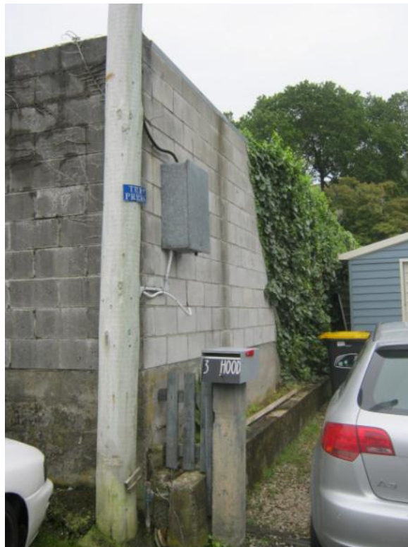
Photo 4: Plant Room back wall (prior to propping)
