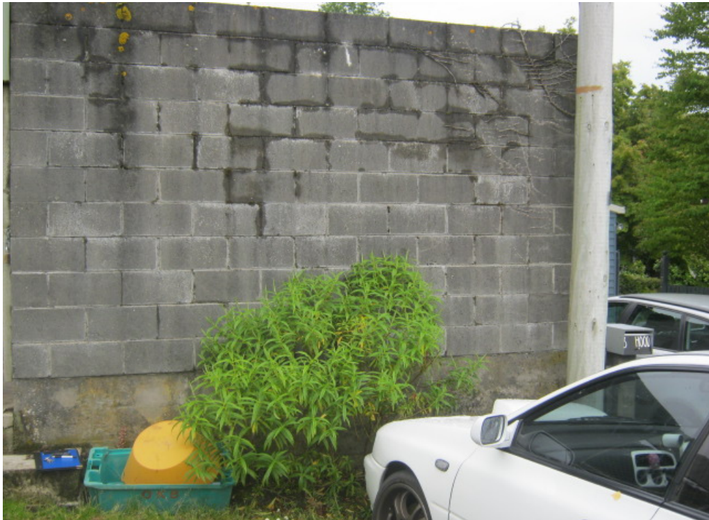
Photo 3: Plant Room side wall (prior to propping)
