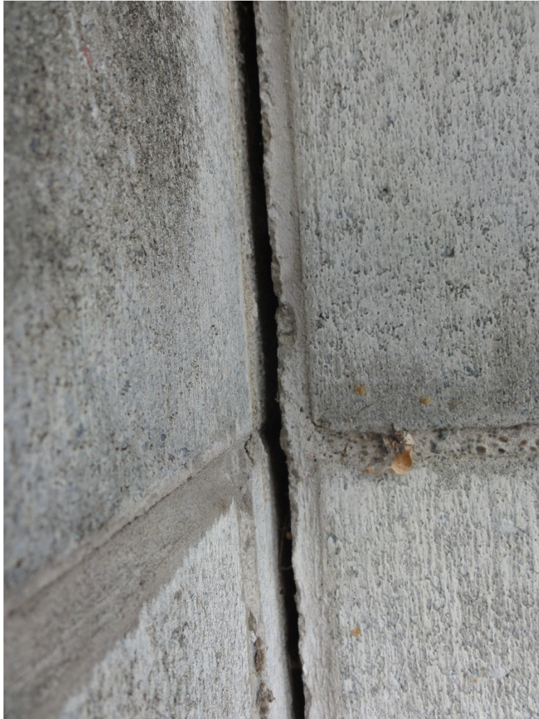
Photo 9: Separation of pier and block boundary wall.
