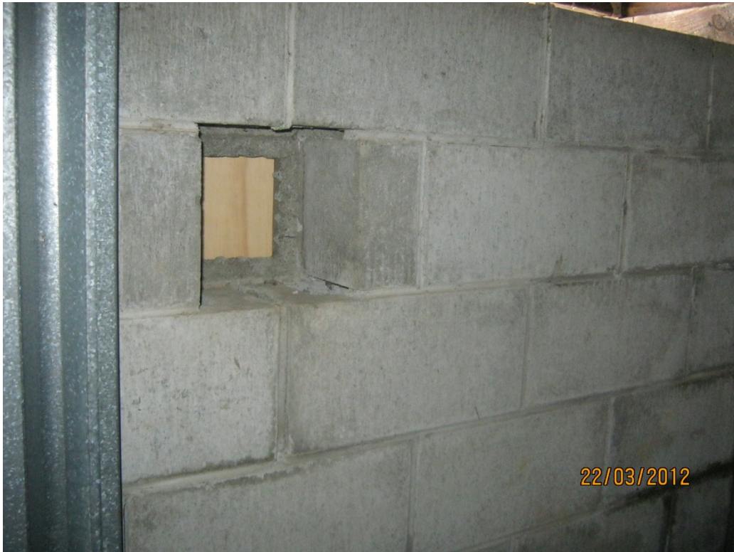
Photo 10: Plant Room – opening in block wall
