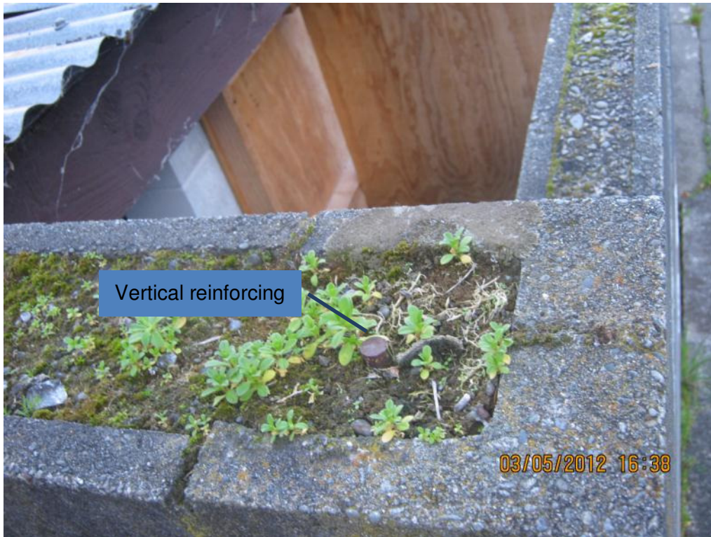
Photo 7: Mens Changing Rooms - front corner bond beam and vertical rebar
