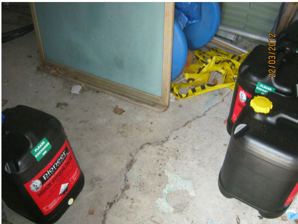
Photo 11: Plant Room – crack in floor (non-seismic damage)
