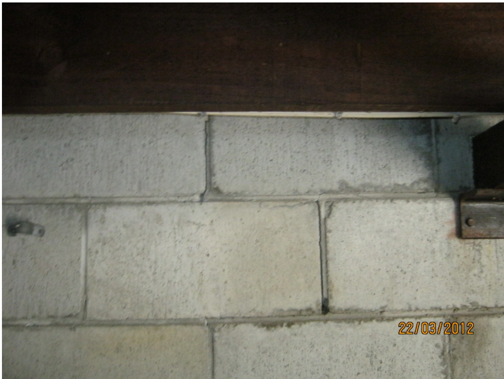
Photo 13: Pool Plant Room block wall opening crack
