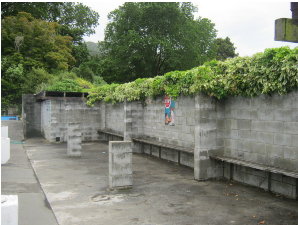
Photo 8: Freestanding boundary wall and Mens Changing Rooms (prior to propping)
