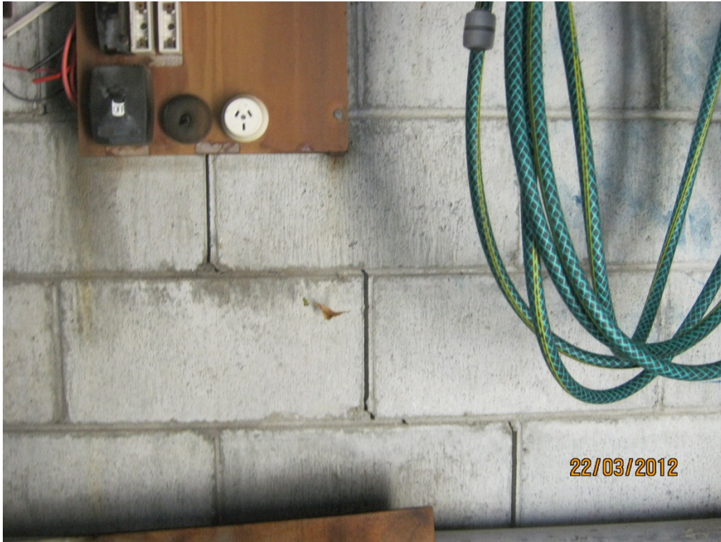
Photo 12: Pool Plant Room - block wall opening crack
