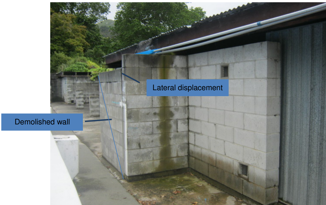
Photo 15: Similar photo as photo 14 – prior to wall demolition and propping
