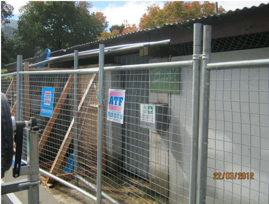
Photo 14: Pool Plant Room block wall propping
