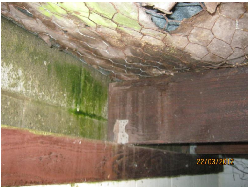
Photo 6: Mens Changing Rooms timber roof purlins and wall plate
