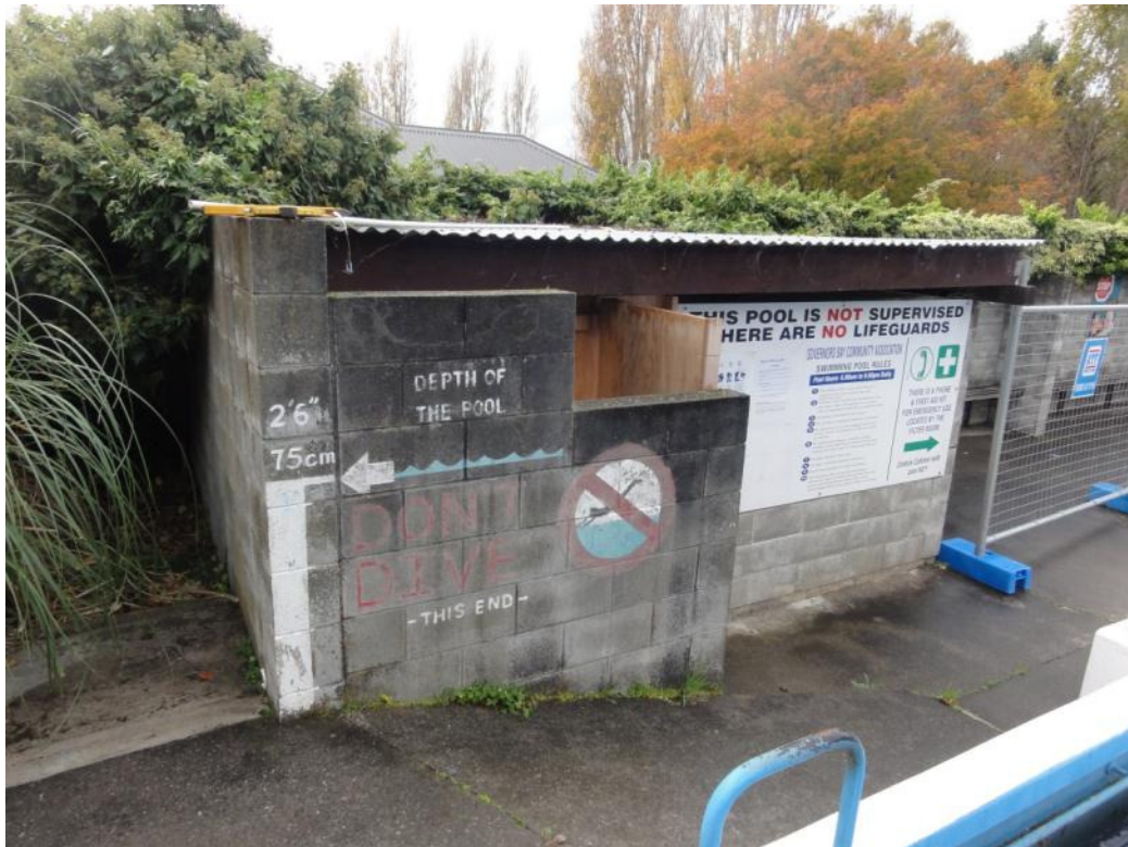
Photo 2: Mens Changing Rooms general photo
