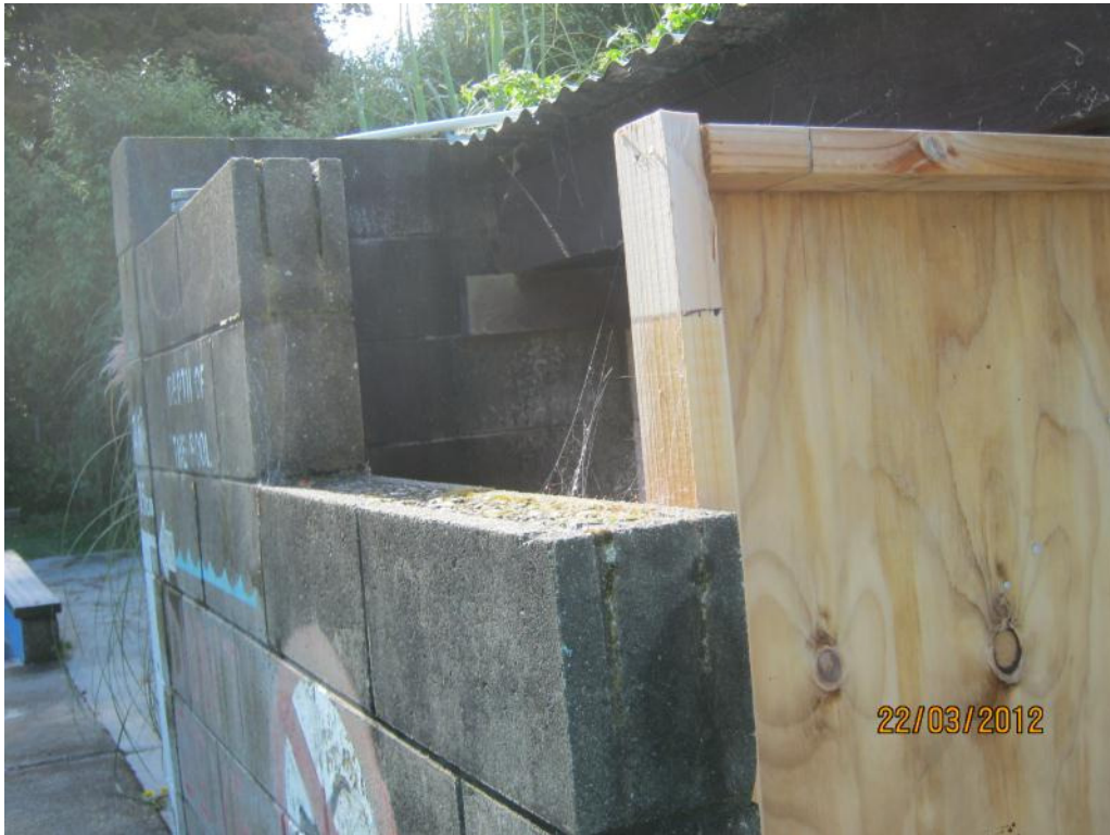
Photo 5: Mens Changing Rooms front corner
