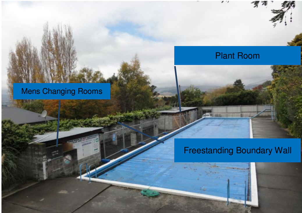
Photo 1: General photo of the structures
