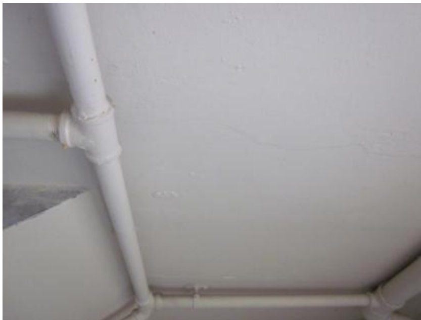
Photograph 10 Minor cracks at 1 st floor slab near the staircase.
