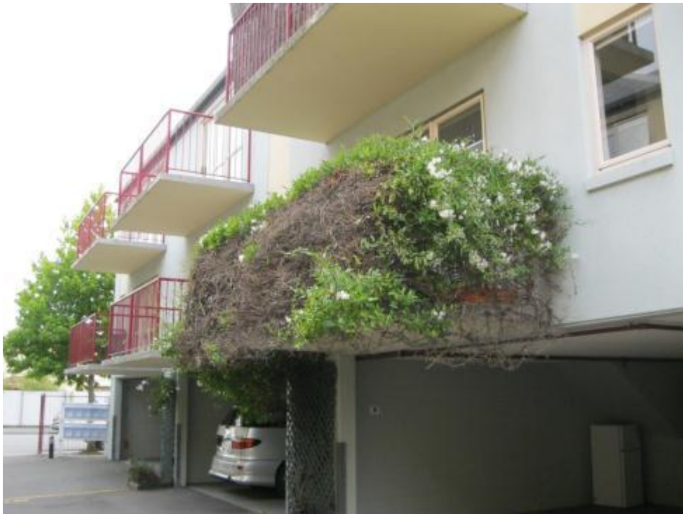
Photograph 2 Gloucester Courts Block B – Front View
