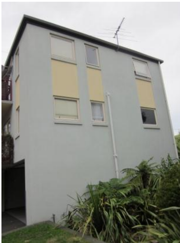
Photograph 4 Gloucester Courts Block B – Side View
