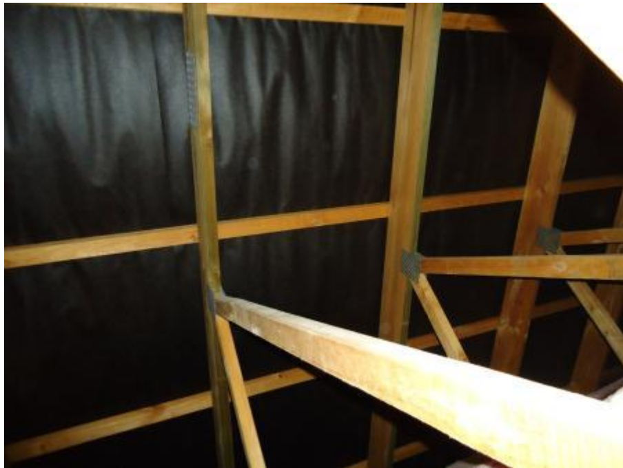
Photograph 14 View of Lightweight metal roof cladding of Gloucester Courts Block A – indicative of building style that may have been used for Gloucester Courts Blocks B and C.
