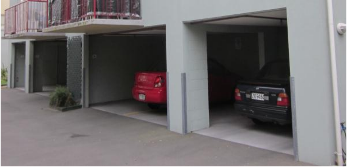
Photograph 13 View of parking space at ground floor (Block C).
