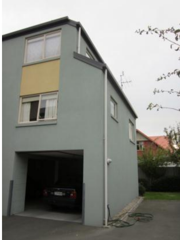
Photograph 7 Gloucester Courts Block C – Side View
