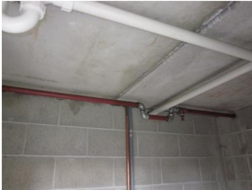
Photograph 11 View of concrete masonry walls and precast floor slab.
