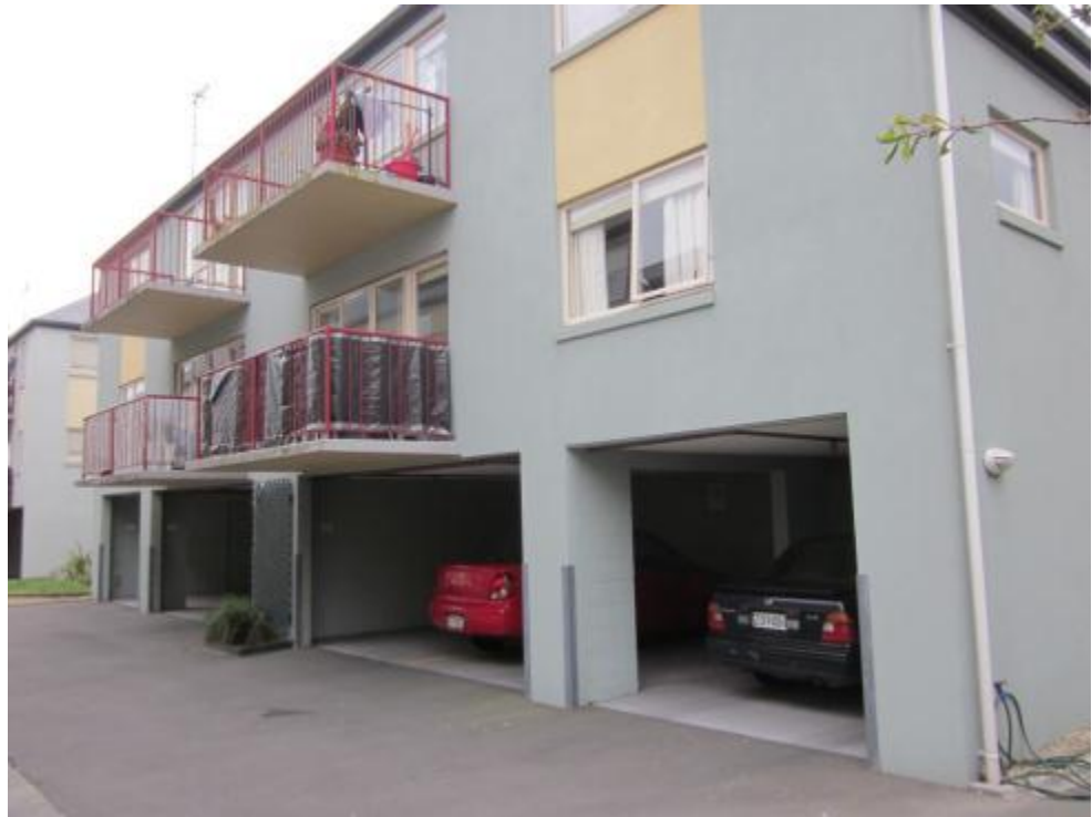
Photograph 5 Gloucester Courts Block C – Front View
