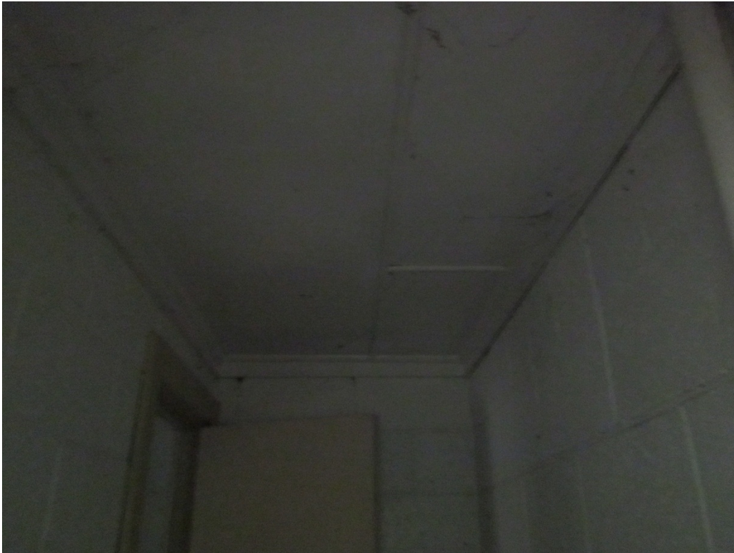
Photo 5: Internal view through window opening
