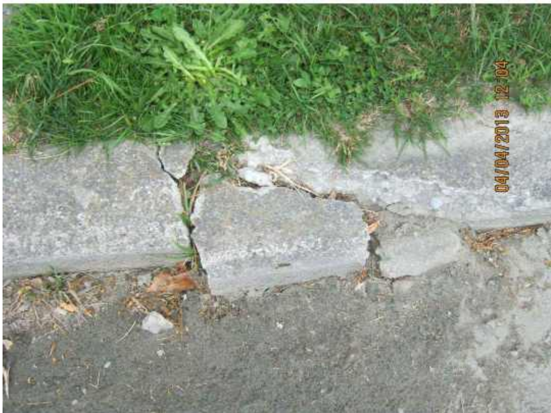
Photograph 4: View of large cracks and broken sections of kerbing, north of Units 1-6 .
