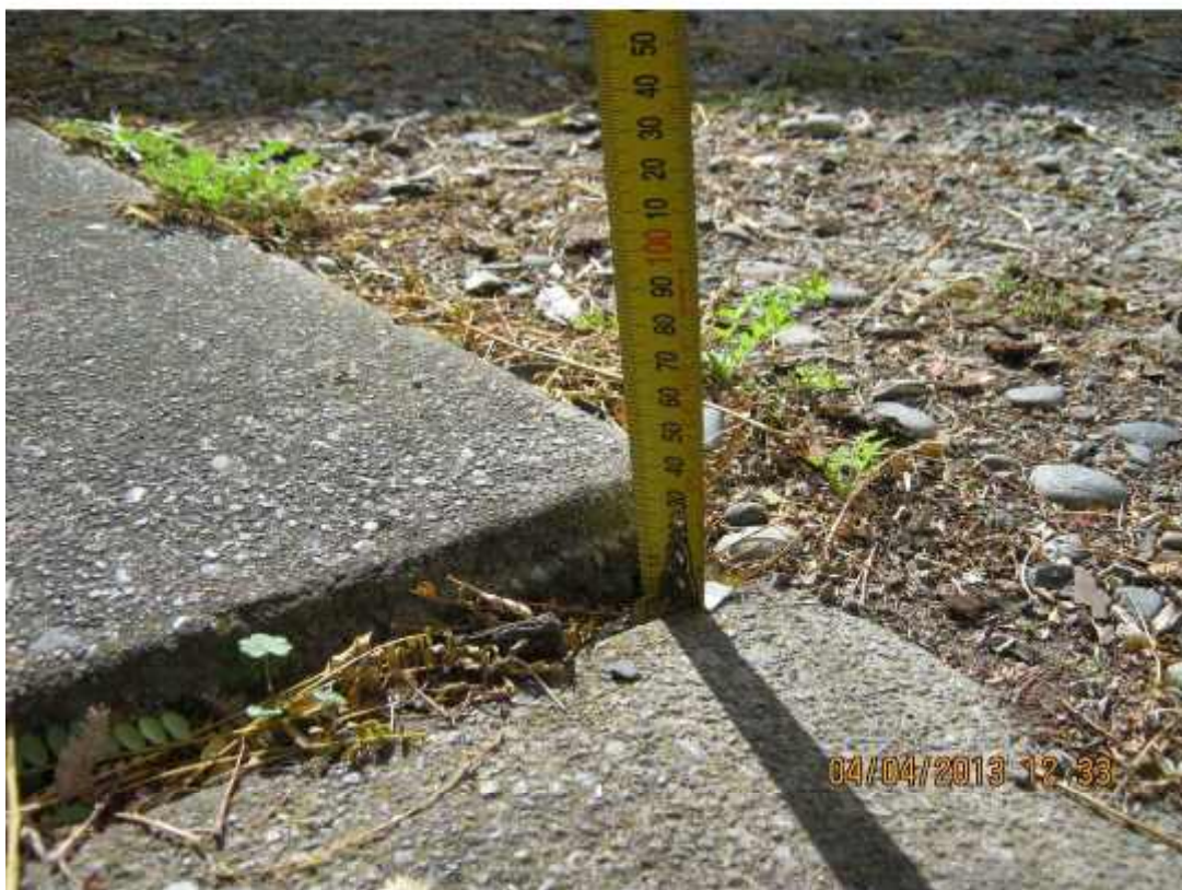
Photograph 12: View of surface evidence of up to 40mm of differential settlement observed in the footpaths in the western half of the complex.
