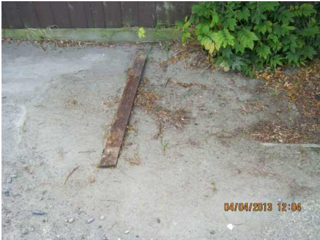
Photograph 3: Observed sand boil in driveway, north of Units 1-6.
