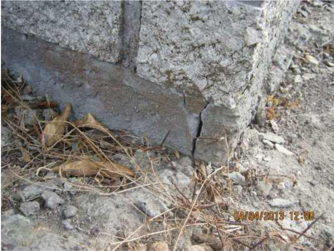
Photograph 5: View of cracking (5mm wide) observed in the footing in the southeast corner of Unit 1.
