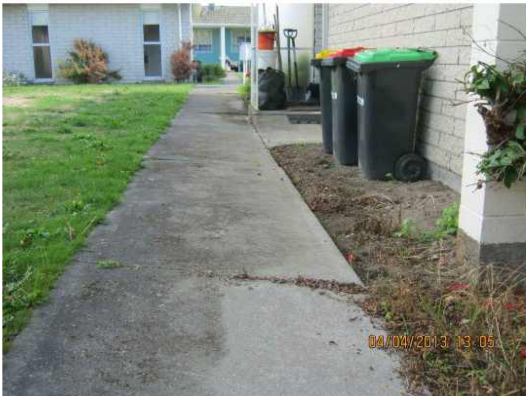
Photograph 14: View of footpath slab (approximately 10m long) along the southern side of Units 9 and 10 that appeared to have undergone differential settlement (up to 40mm) as a result of liquefaction and now slopes in a northerly direction towards the structure.
