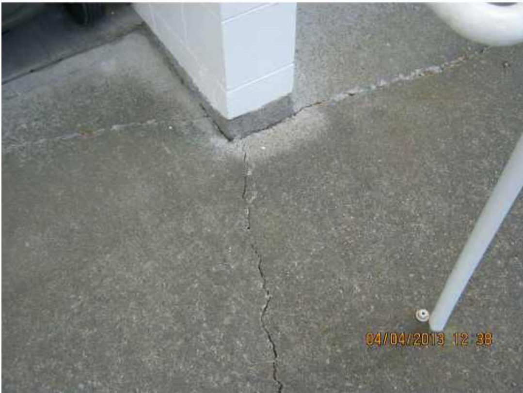
Photograph 6: View of large cracks up to 5mm wide and 1.5m long, observed in the front porch slabs of most units.
