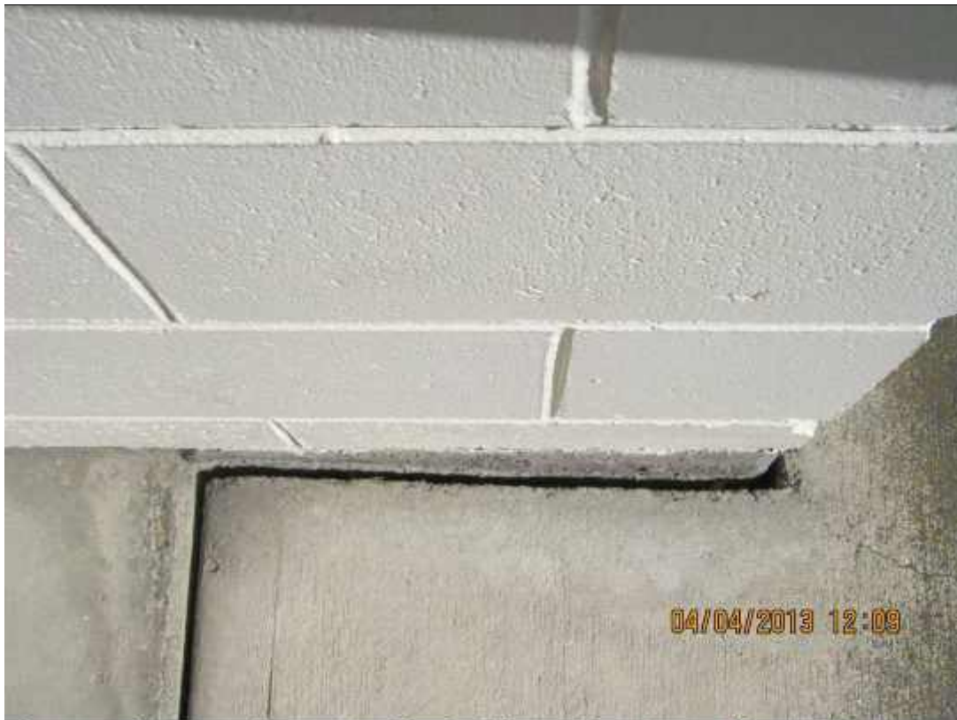
Photograph 7: View of separation of porch slab away from Party wall footing (by approximately 20mm) observed along the northern side of Unit 32.
