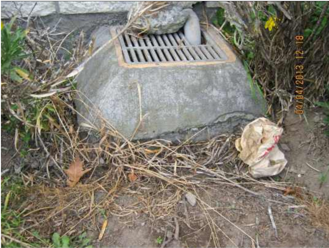
Photograph 9: View of exposed concrete observed around drain where the ground may have settled, at the northeastern corner of Unit 34.
