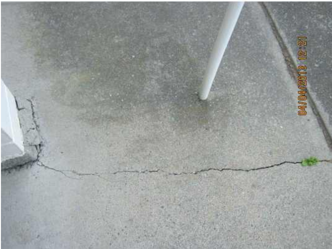
Photograph 10: View of cracking of porch slab (5mm wide x 1m long) and spalling of Party wall footing concrete observed on the northern side of Units 35 and 36.
