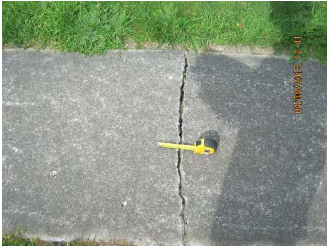
Photograph 13: View of large crack across entire width of footpath slab, east of Units 21 and 22, indicating differential settlement.
