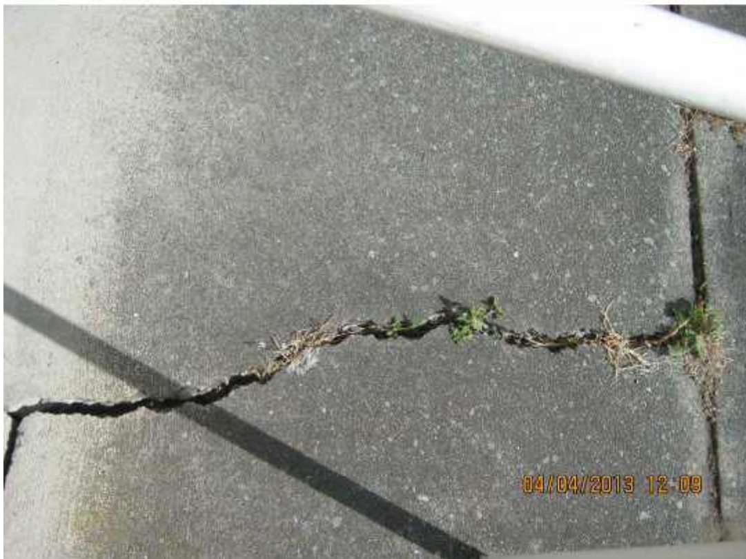
Photograph 8: View of crack in slab (approximately 1m long and 20mm wide) observed along the northern side of Unit 32.
