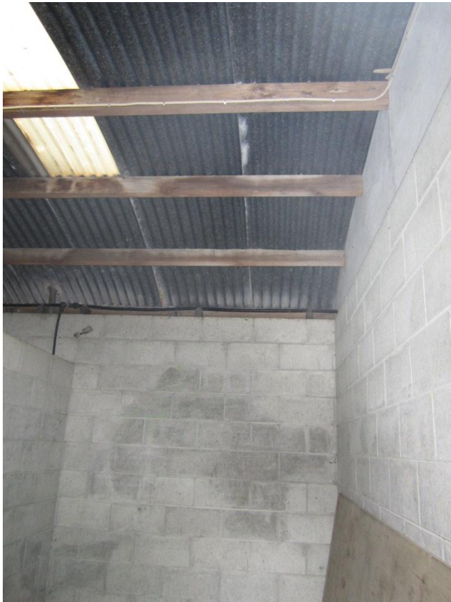
Photograph 4 Timber roof rafters
