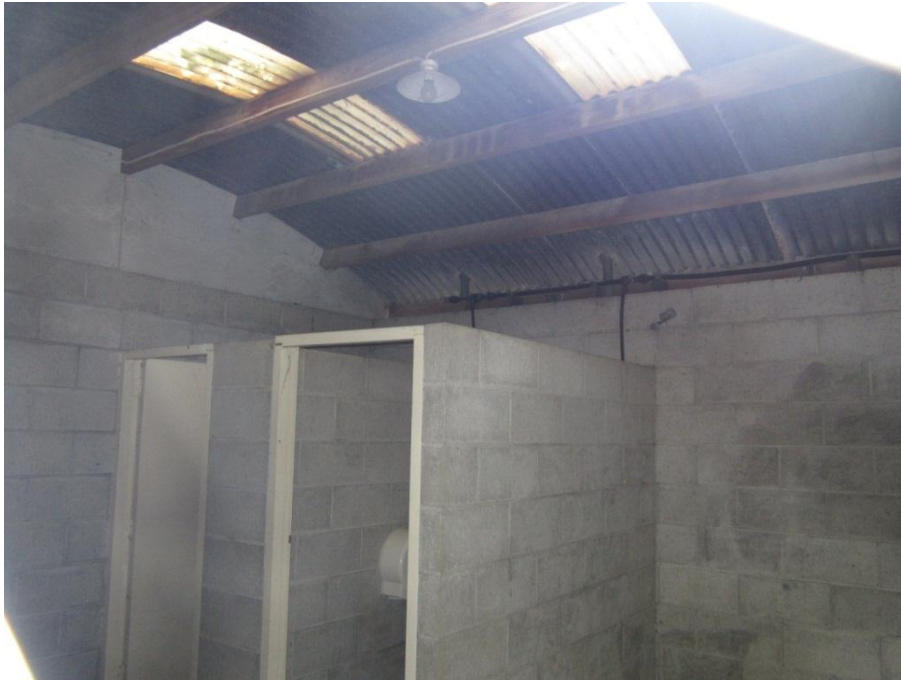
Photograph 3 90mm thick internal walls
