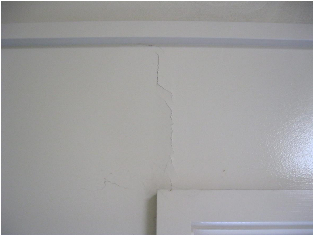
Photograph 7 Flaking of paint work.
