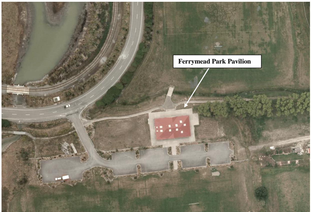
Figure 3 Post February 2011 Earthquake Aerial Photography 2
