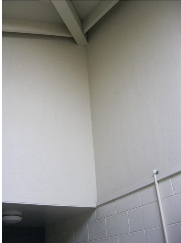
Photograph 9 Timber and masonry interior wall.
