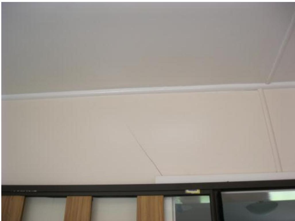
**Photograph 6 Cracking to plasterboard linings.**
