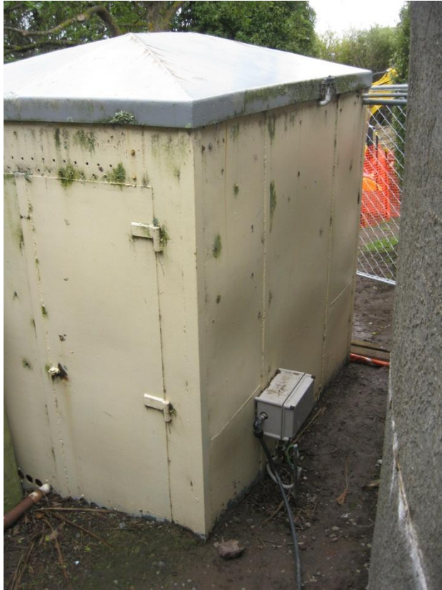
Photograph 4 Hipped steel-plate roof
