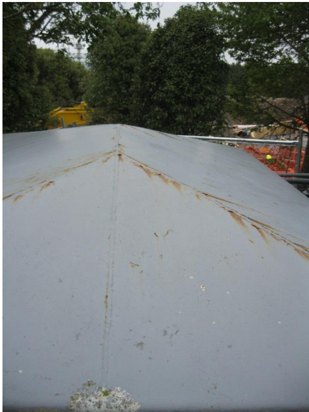
Photograph 4 Hipped steel-plate roof
