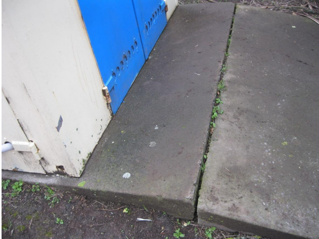
Photograph 5 Concrete slab on grade
