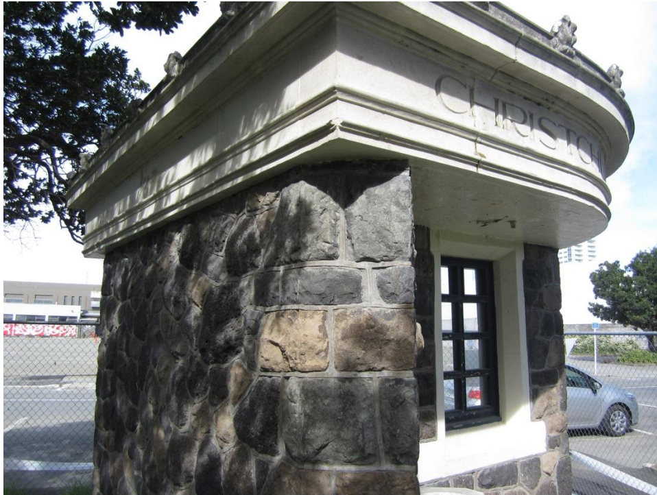
Photograph 5 Stone masonry walls
