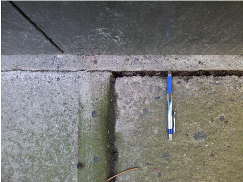
■ Figure 8 Minor gap between the building and external ground slab
