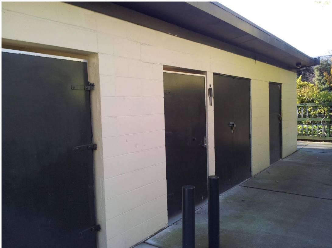
■ Figure 7 Front view of the building (southern elevation)
