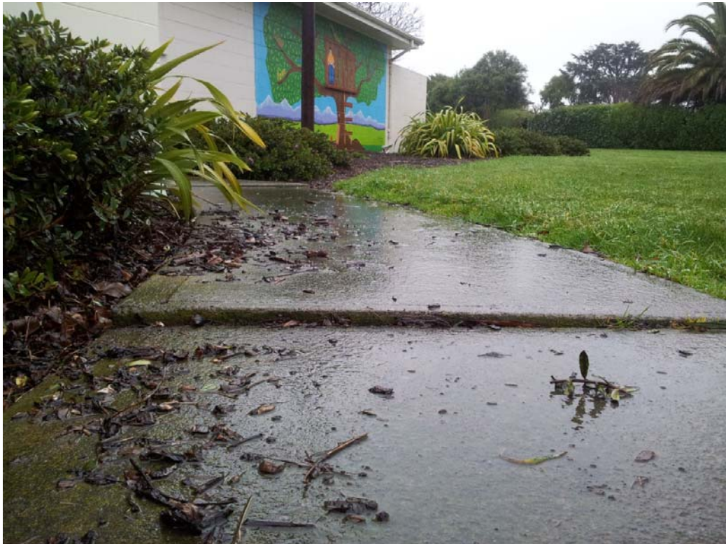
■ Figure 6 Observed settlement of pavement slabs
