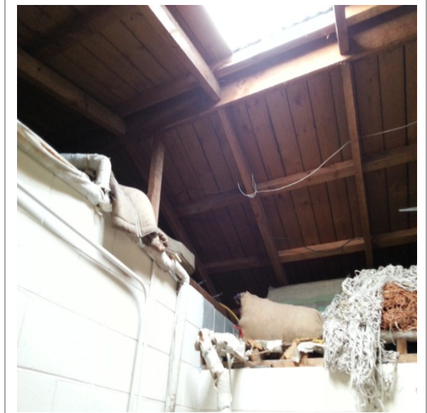
Photo 12: Timber framed roof truss (1)
