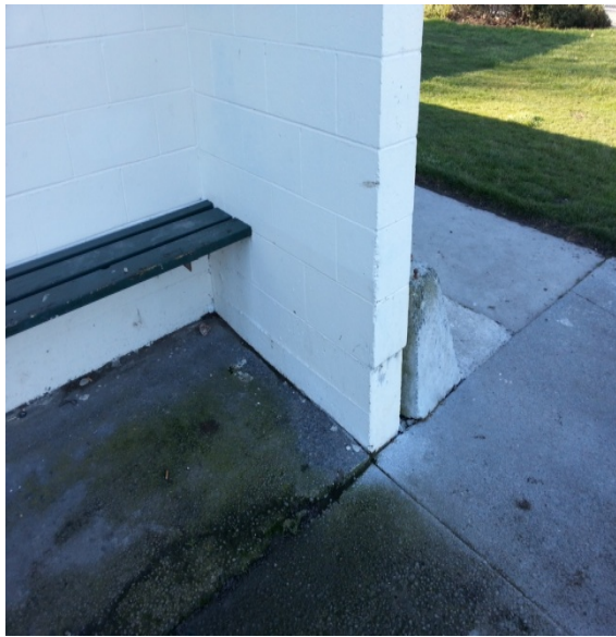
Photo 17: View of concrete foundation beneath masonry
