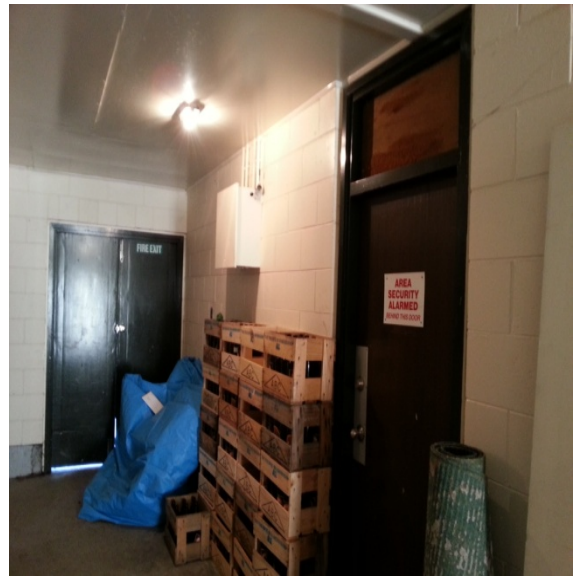
Photo 14: Hallway of changing rooms (2)
