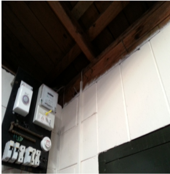
Photo 13: Timber framed roof truss (2)
