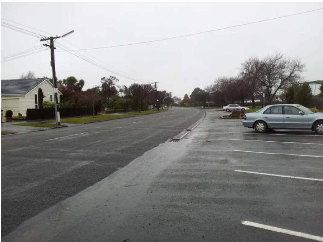
■ Figure 7 No apparent damage to the section of Condell Avenue near the site
