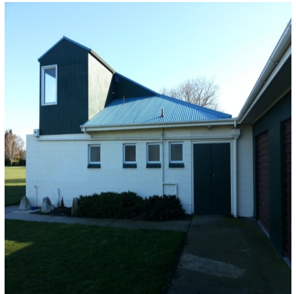
Photo 16: East elevation doorway into changing rooms on the right
