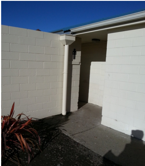
Photo 7: Entrance to men's toilet
