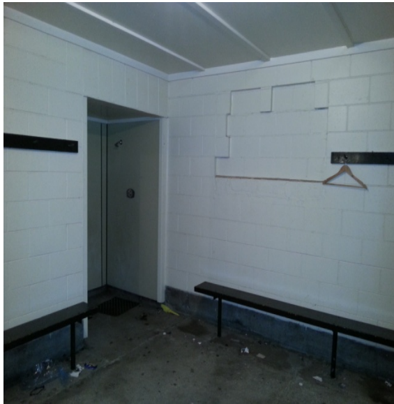
Photo 15: Cricket changing rooms (3)
