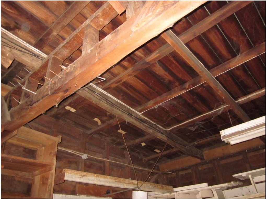
Photograph 7: Timber framed roof with timber gurder truss
