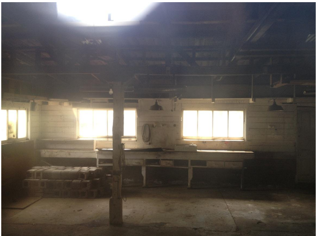
Photograph 4: Interior timber panelling/ Timber column with concrete plinth
