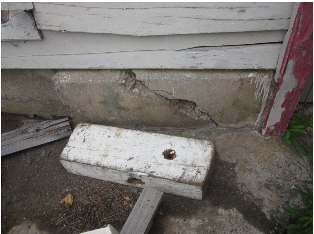
Photograph 6: Existing cracking to the perimeter strip footing may have opened up further in recent seismic activity
