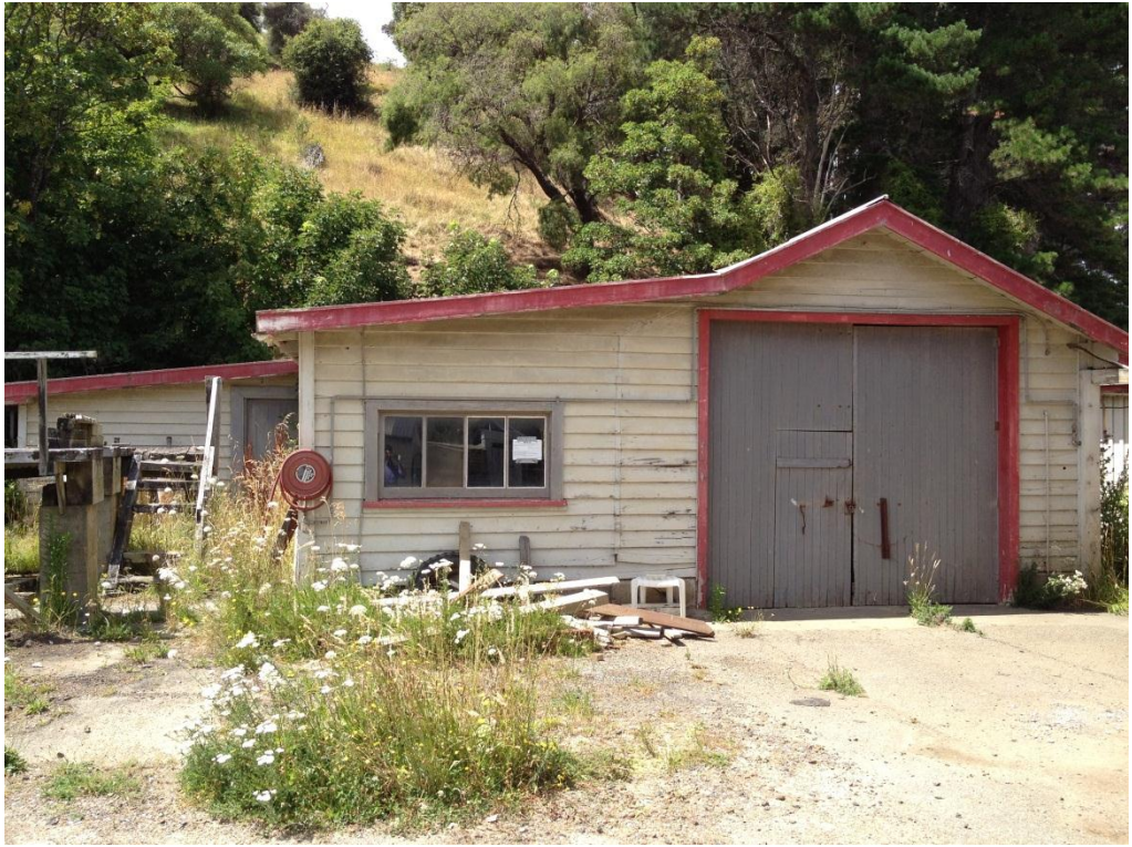
Photograph 1: West (front) Elevation
