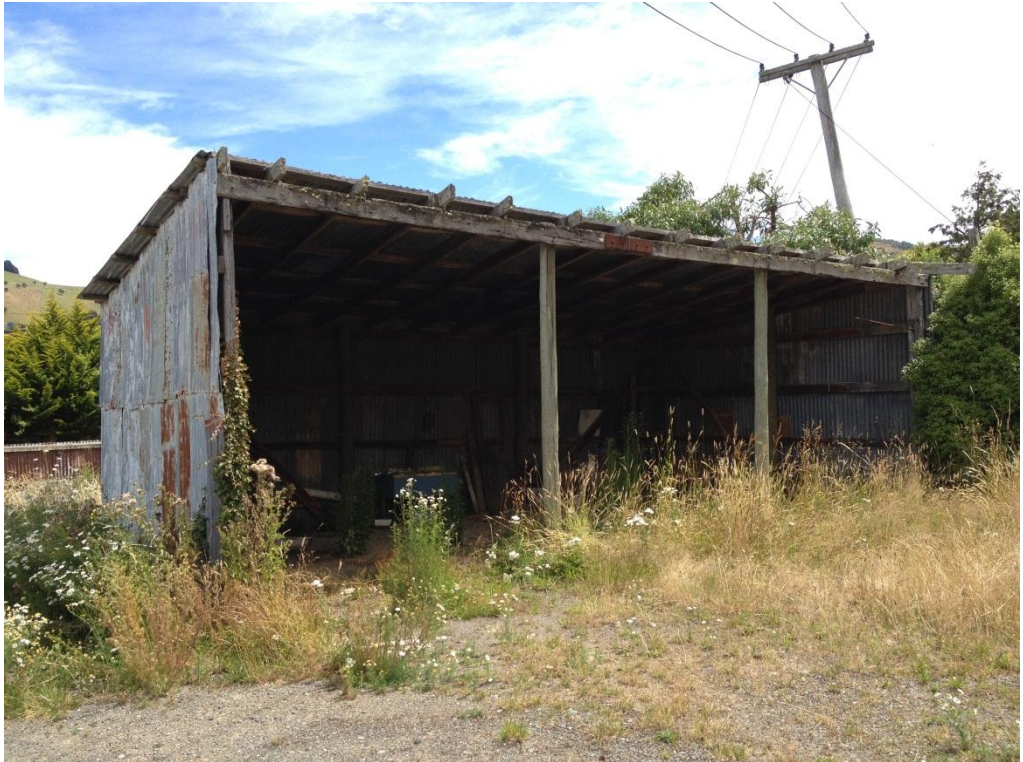
Photograph 1: East (front) Elevation
