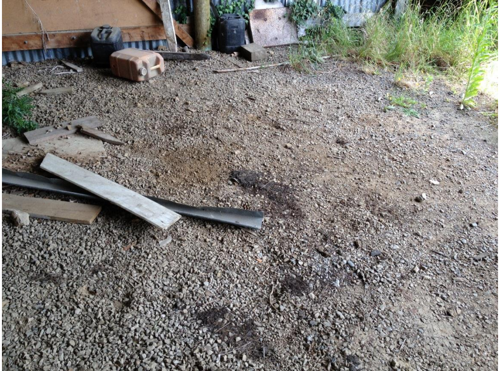
Photograph 5: Loose gravel ground material
