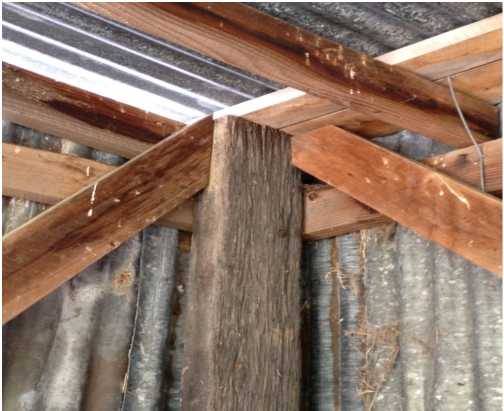
Photograph 6: Diagonal bracing to column connection
