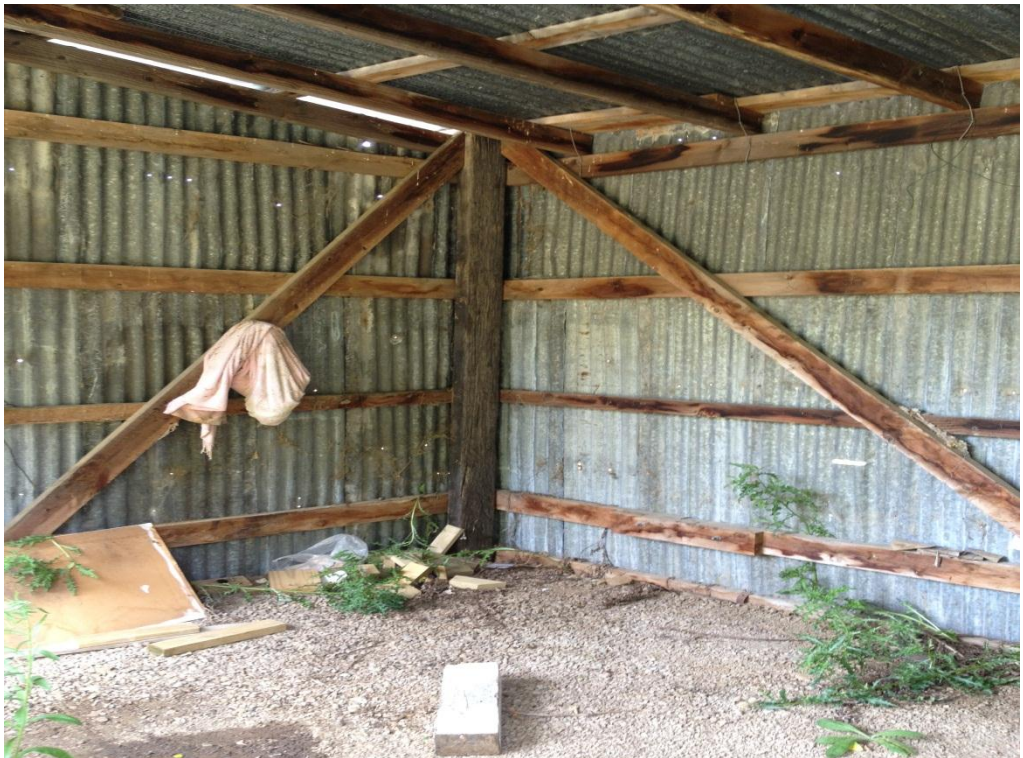
Photograph 3: Tension/Compression bracing
