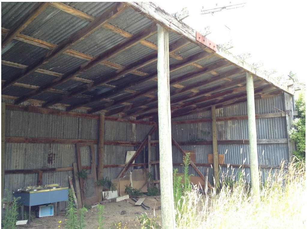
Photograph 4: Pitched timber framed roof structure
