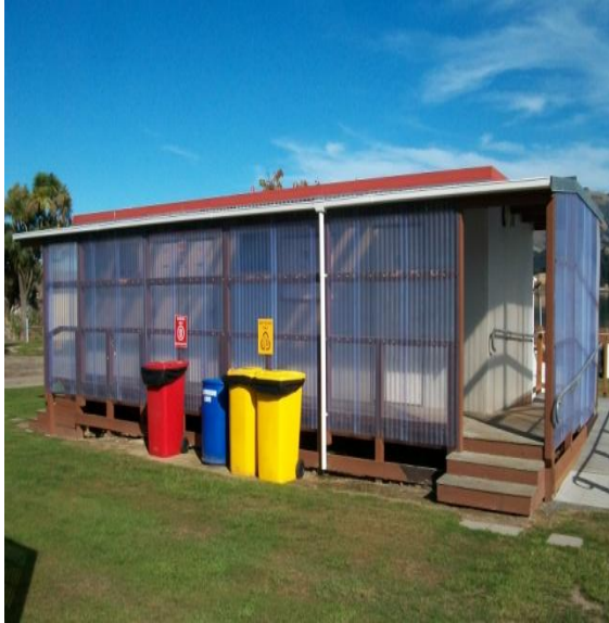
Photo 1: The east elevation of the toilet block
