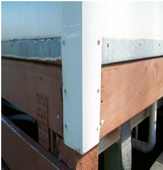
Photo 7: Typical corner angle showing popped nails where it is fixed to the supporting timber framing
