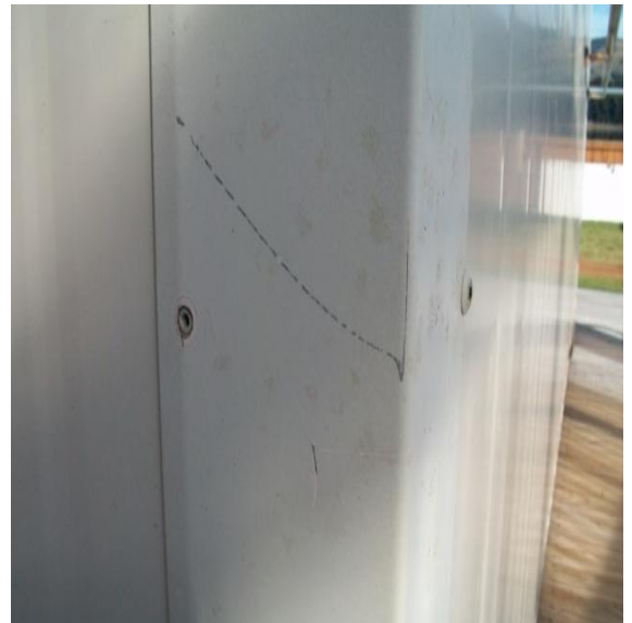
Photo 4: Detail of sheared rivets in the north east corner of the building
