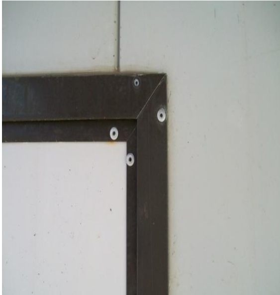
Photo 5: Example of sheared rivets on the door trim
