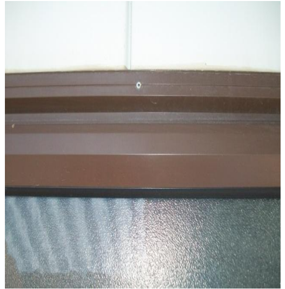
Photo 6: Example of sheared rivets on the window framing
