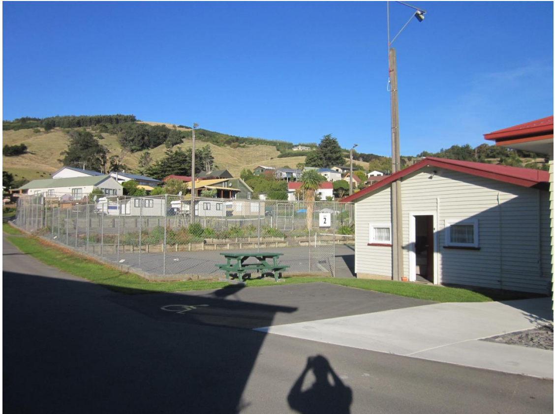
■ Figure 5 Overview of the Community Hall
