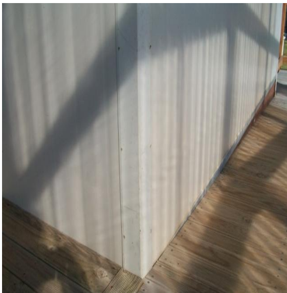
Photo 3: The north east corner of the structure where rivets have sheared
