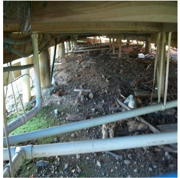
Photo 2: The sub floor structure showing the short timber poles
