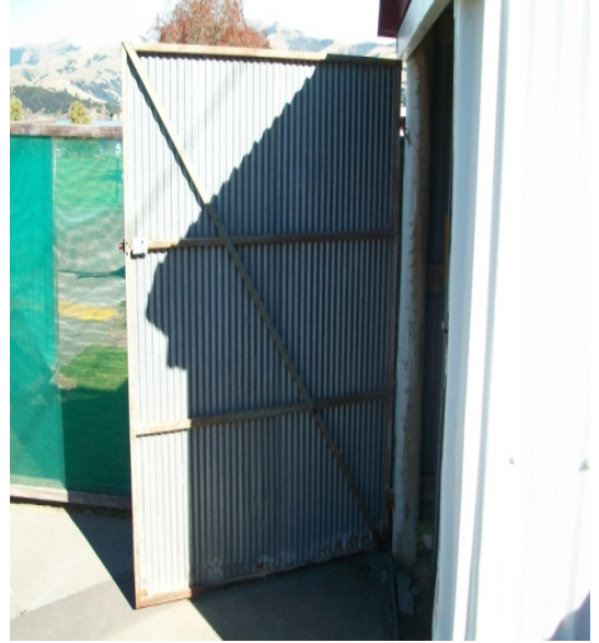
Photo 2: The steel framed door in the south side of the shed
