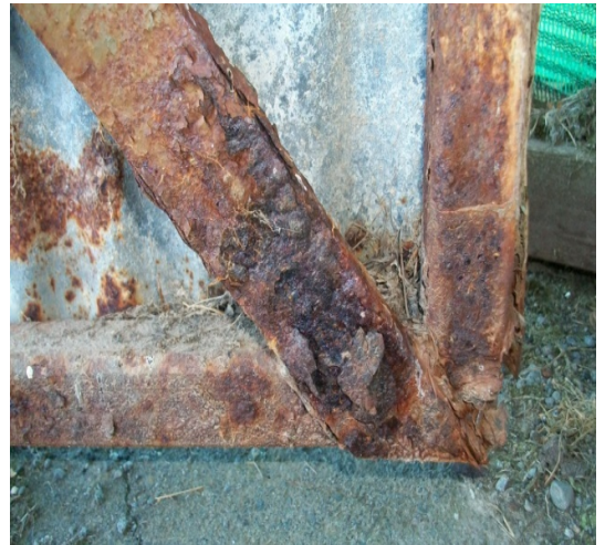
Photo 4: Example of corrosion present on the steel framing of the shed door
