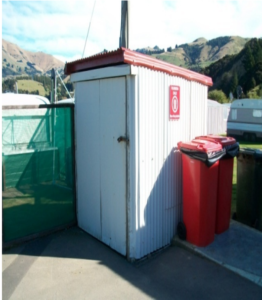
Photo 1: The south and east elevations of the mower shed
