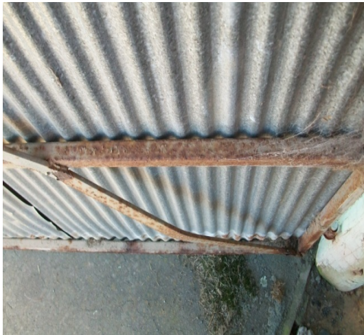
Photo 3: Detail of the shed door bracing showing the buckled flat bar
