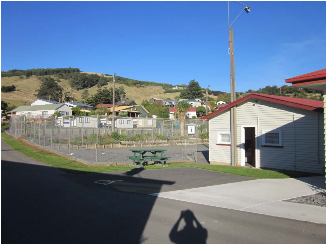
■ Figure 5 Overview of the Community Hall
