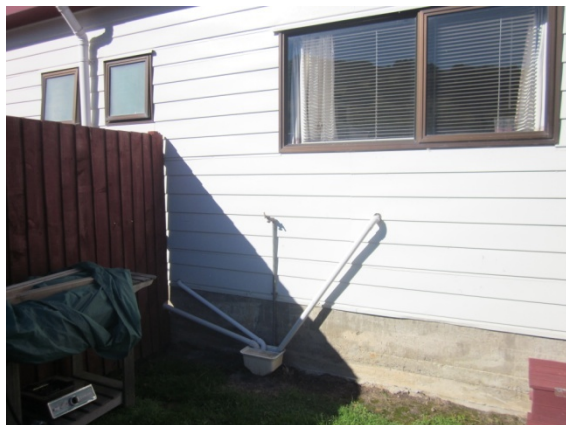
Photo 1: The north face of the building showing the external drain, adjacent to which, cracking in the foundation was observed
