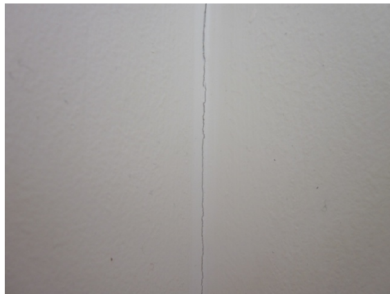
Photo 4: Typical separation found between internal wall lining at the junction between the perimeter walls
