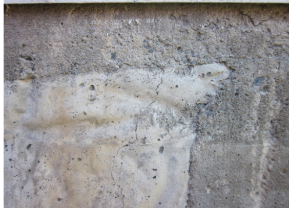
Photo 2: Details of hairline cracking in the north face of the foundation
