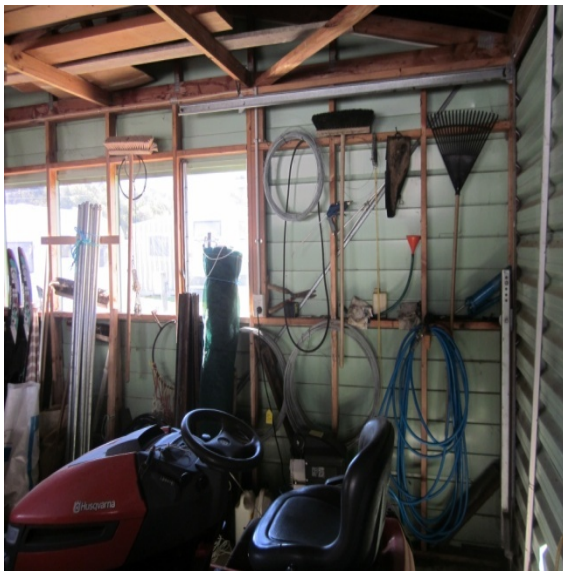
Photo 3: Elevation on an internal wall of the garage showing timber framing and steel strap bracing
