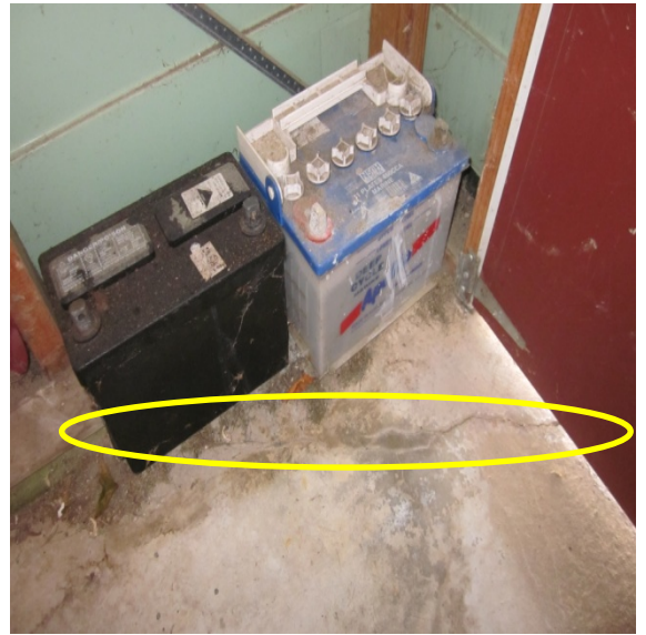
Photo 6: The crack in the south west corner of the foundation slab
