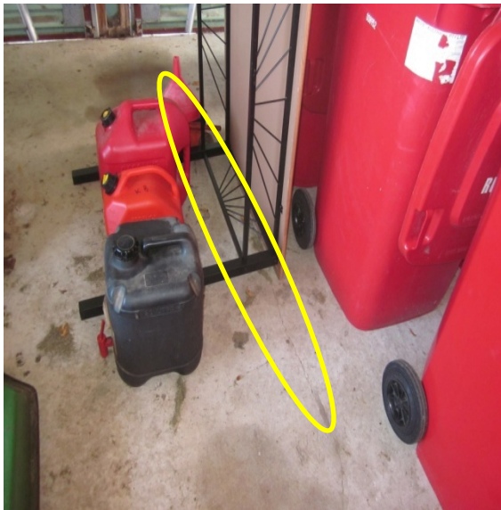
Photo 7: The crack through the centre of the foundation slab
