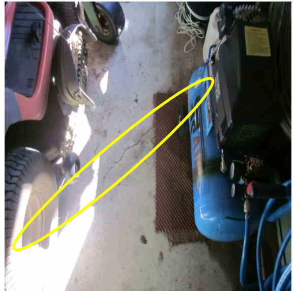
Photo 8: The crack in the south east corner of the slab
