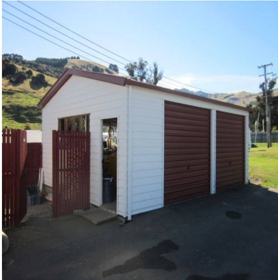
Photo 1: The west and south elevations on the garage
