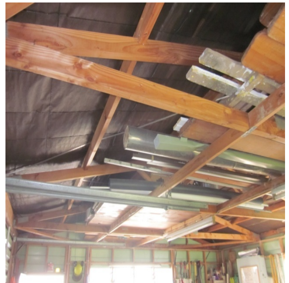
Photo 4: The roof framing of the garage showing the timber A-frame trusses, timber purlins and steel strap bracing
