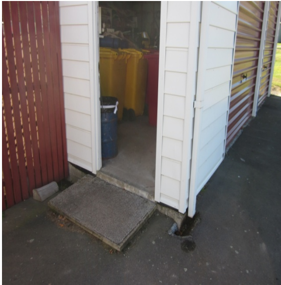
Photo 5: The door at the south end of the west wall where one of the cracks in the foundation are located
