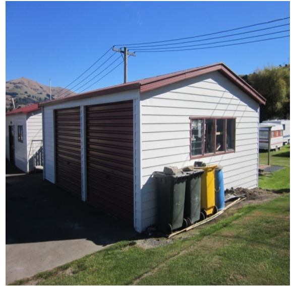
Photo 2: The south and east elevations of the garage
