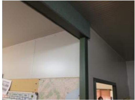
Photo 3 – Internal Steel Beam and Post
