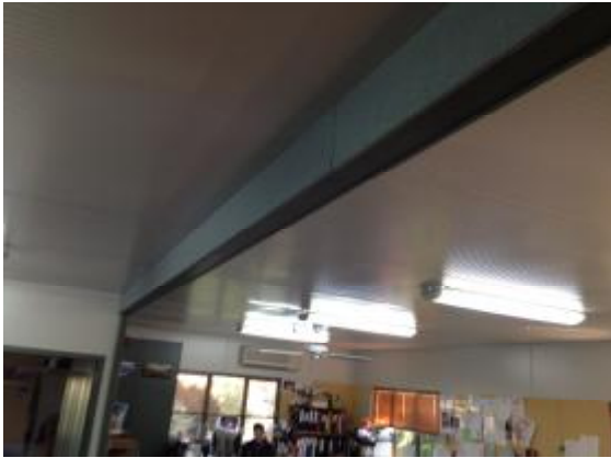
Photo 2 – Internal Steel Beam and Post
