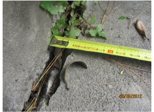
Photo 6: Cracking up to 40mm wide through steps
