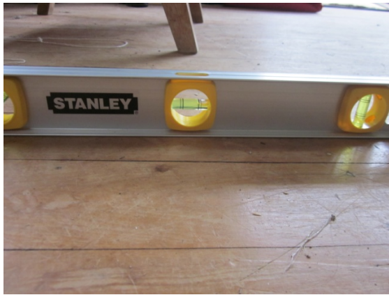
Photo 17: significant slope towards the end wall in the west of the scouts den
