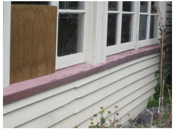
Photo 10: Rotting of the timber window framing
