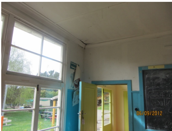
Photo 15: Roof lining damage in the NE corner of the scouts den
