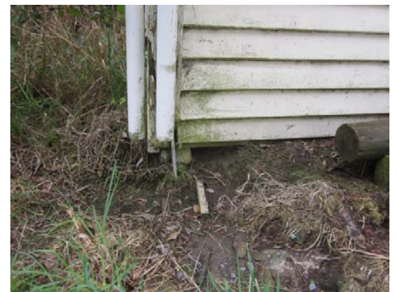
Photo 20: Settled west end of the building.
