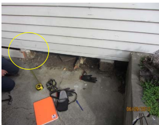
Photo 21: Pile broken approx 50mm below ground level
