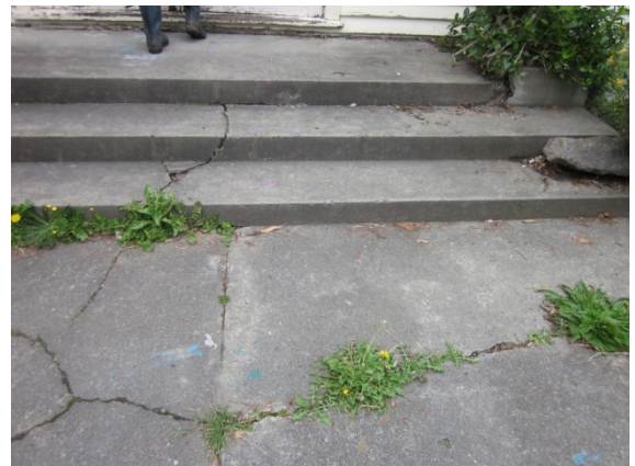
Photo 4: Cracking to the concrete steps and concrete slabs around the entry to the building
