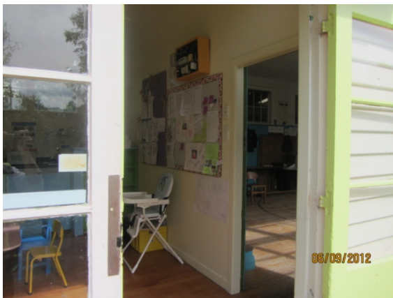
Photo 11: Wall dividing renovated playcentre left of shot and the original scouts den right of shot.
