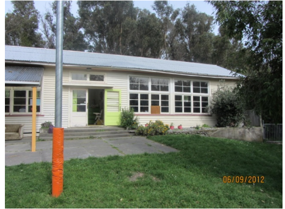
Photo 2: West end of the building - Scouts Den
