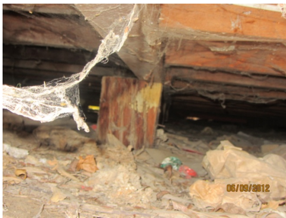
Photo 19: Bearer off centre of pile along the north side of the building
