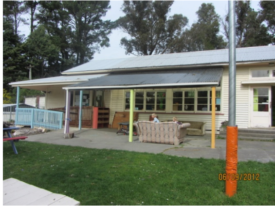
Photo 1: Eastern end of the building - Playcentre
