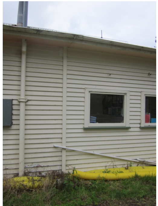
Photo 8: Light timber framed walls with weatherboard cladding.
