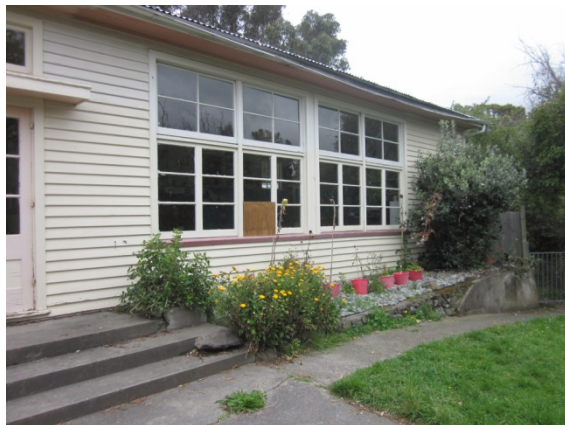
Photo 3: View looking west along the north face of the original and unrenovated 1920s building section
