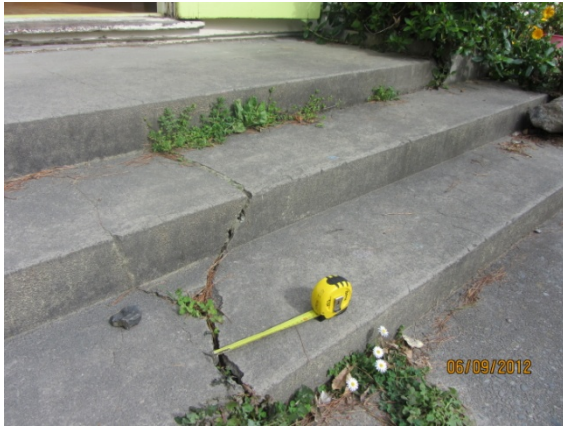
Photo 5: Cracking to the bulk concrete steps
