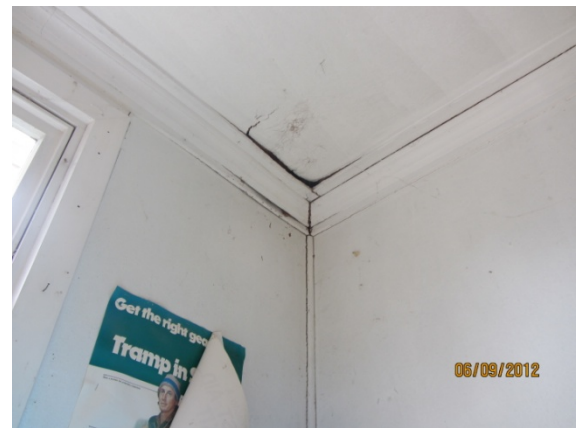
Photo 16: Close up of damage pictured photo 15
