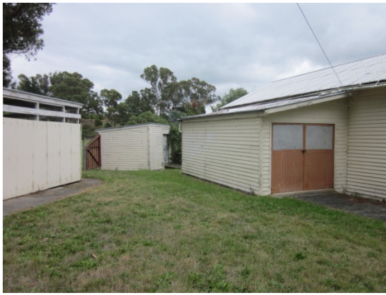
Photo 9: The buildings weather boards are becoming rotten, especially to the east.
