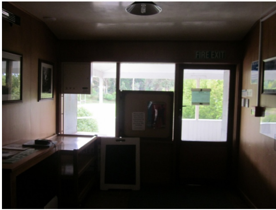
Photo 19: Typical plasterboard damage to the hall entrance
