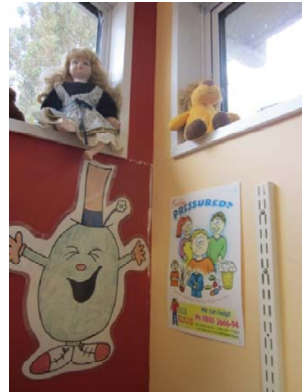
Photo 26: Plasterboard separation in the Library
