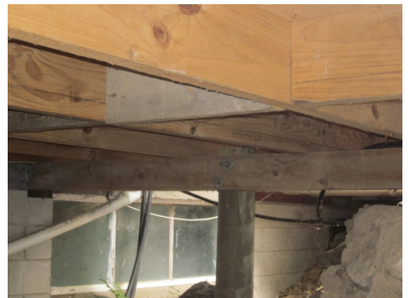
Photo 28: Storage rooms on south side of back stage area timber floor on joists on bearers supported by timber piles
