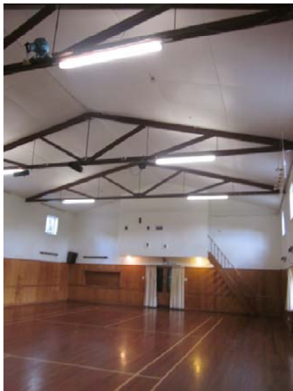
Photo 7: Community Hall with timber trusses apex approx 7m
