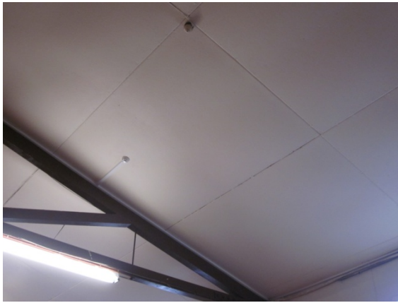
Photo 9: Timber roof cladding
