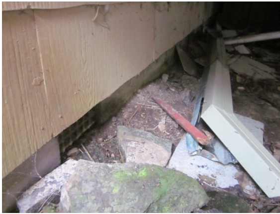
Photo 29: Ventilation points around concrete perimeter ring beam for internal ventilation
