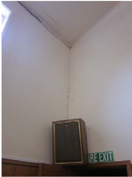
Photo 15: Typical plasterboard damage to the hall
