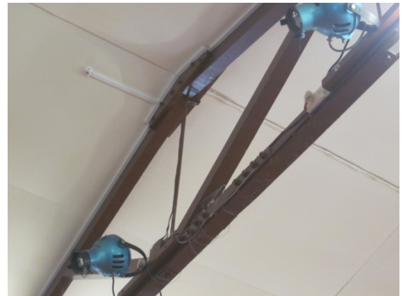
Photo 8: Composite truss made up of steel rods and timber with timber/ timber connections created with steel gussets
