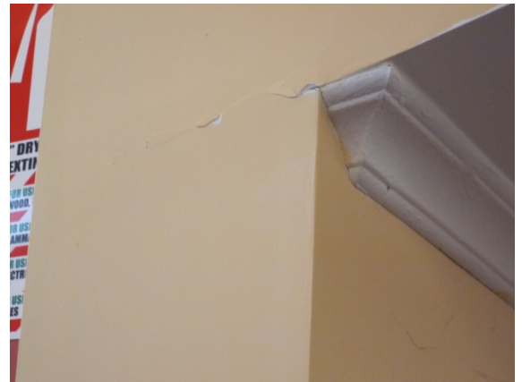
Photo 22: Plasterboard separation in the Library
