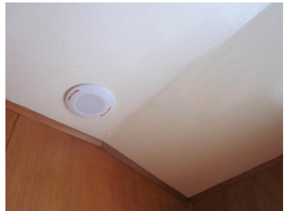
Photo 18: Typical plasterboard damage to the hall entrance
