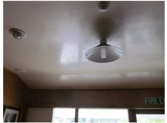
Photo 20: Typical plasterboard damage to the hall entrance
