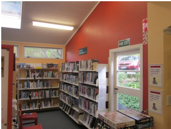
Photo 21: Plasterboard separation in the Library
