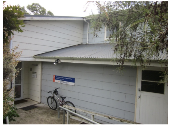
Photo 6: View of the library entrance past pre-existing structure
