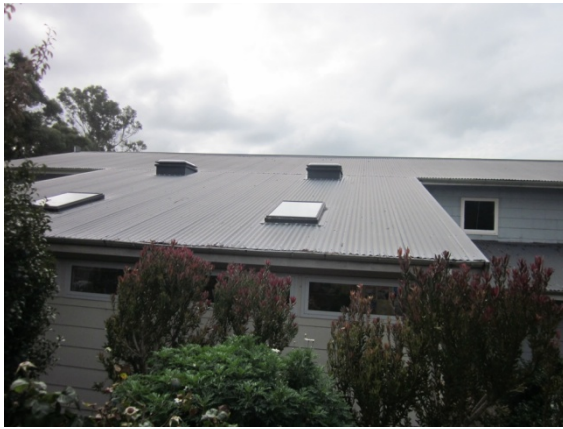
Photo 5: View looking North at the library addition
