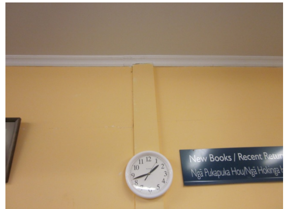
Photo 24: Plasterboard separation in the Library
