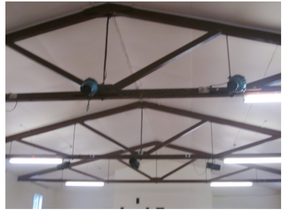
Photo 10: Timber trusses – no apparent damage
