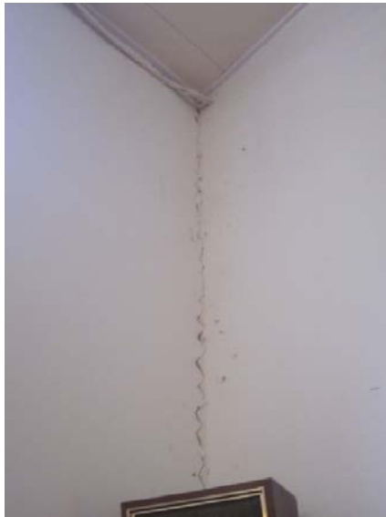
Photo 17: Typical plasterboard damage to the hall
