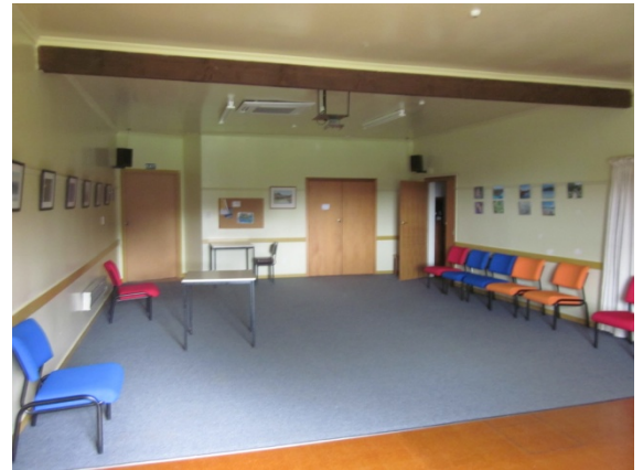
Photo 12: Roof supported by a timber beam
