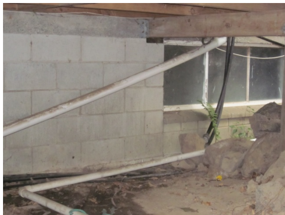
Photo 27: Back stage area supported by masonry block around the perimeter
