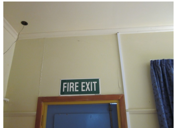
Photo 14: Typical separation between internal wall linings
