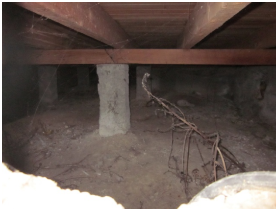
Photo 31: Floor and foundation system under the hall and foyer. Timber flooring on joists on bearers supported by concrete piles. View south
