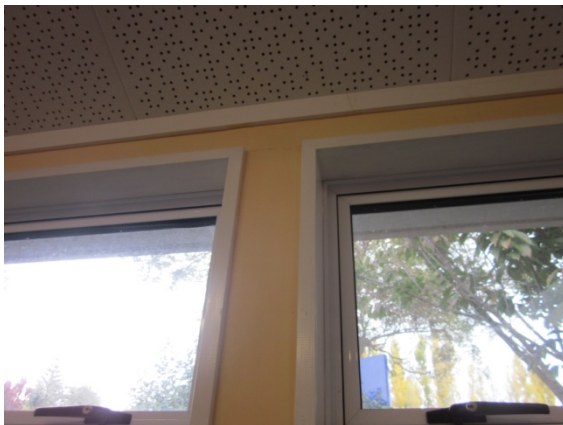
Photo 23: Plasterboard separation in the Library
