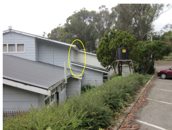
Photo 4: View East along the south side of the building. Library sharing the south wall
