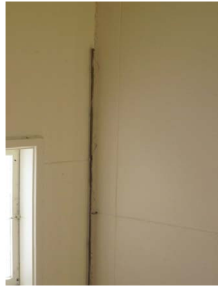
Photo 16: Typical plasterboard damage to the hall
