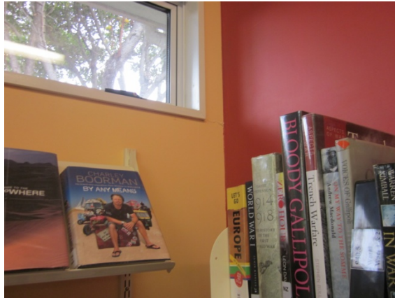
Photo 25: Plasterboard separation in the Library
