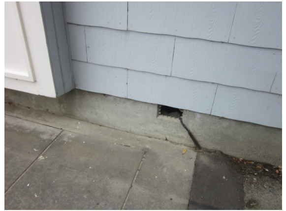
Photo 30: Ventilation point on buildings NW used to take photos 31 and 32
