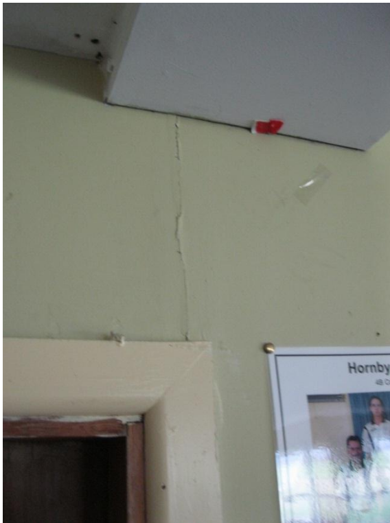
Photograph 8 Example of typical plasterboard cracking above windows and doors of clubrooms
