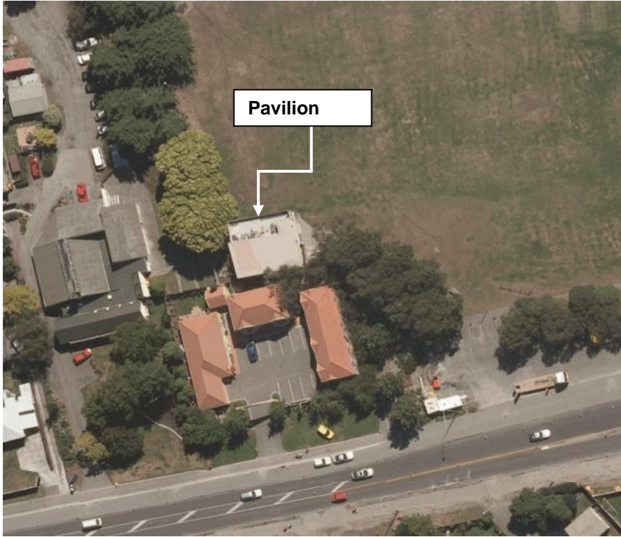
Figure 3 Post February 2011 Earthquake Aerial Photography 2
