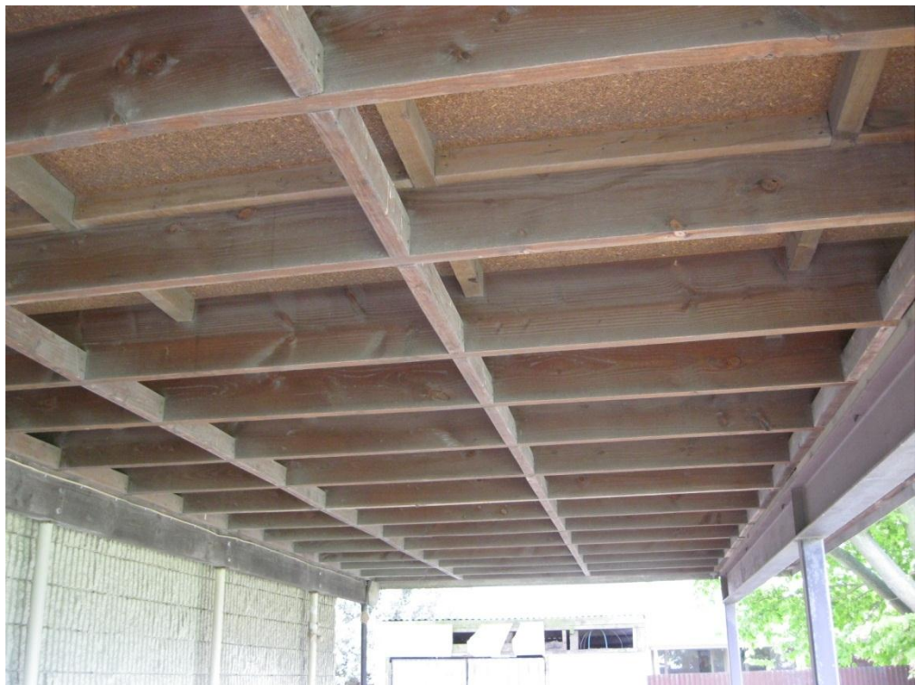
Photograph 4 Underside of the first floor framing supported by steel framing to the north and concrete masonry walls to the south.
