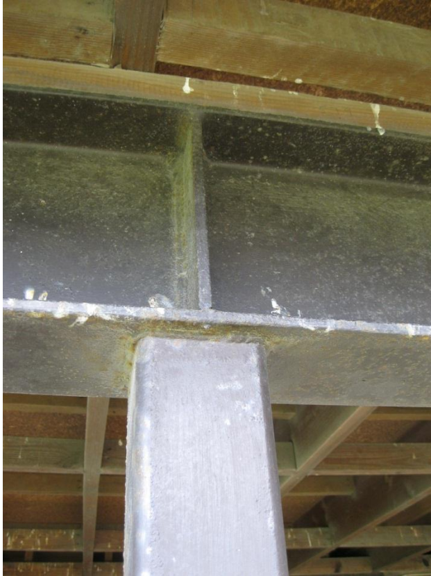
Photograph 5 Steel framing with web stiffener above SHS column.
