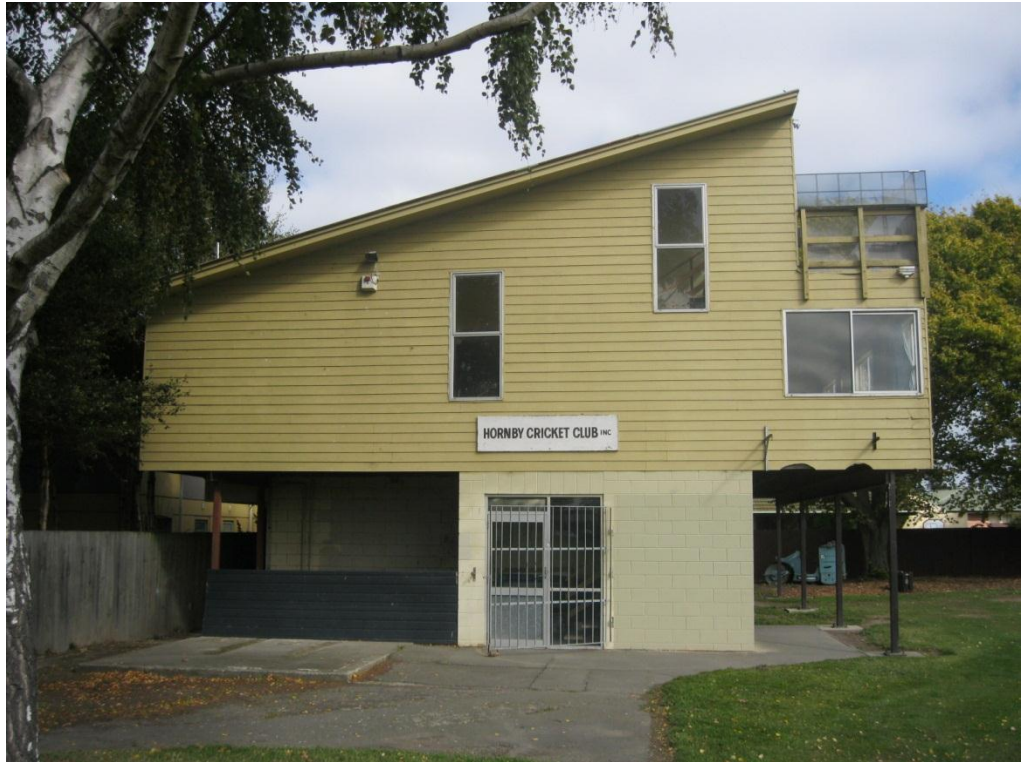
Photograph 3 East face of pavilion.
