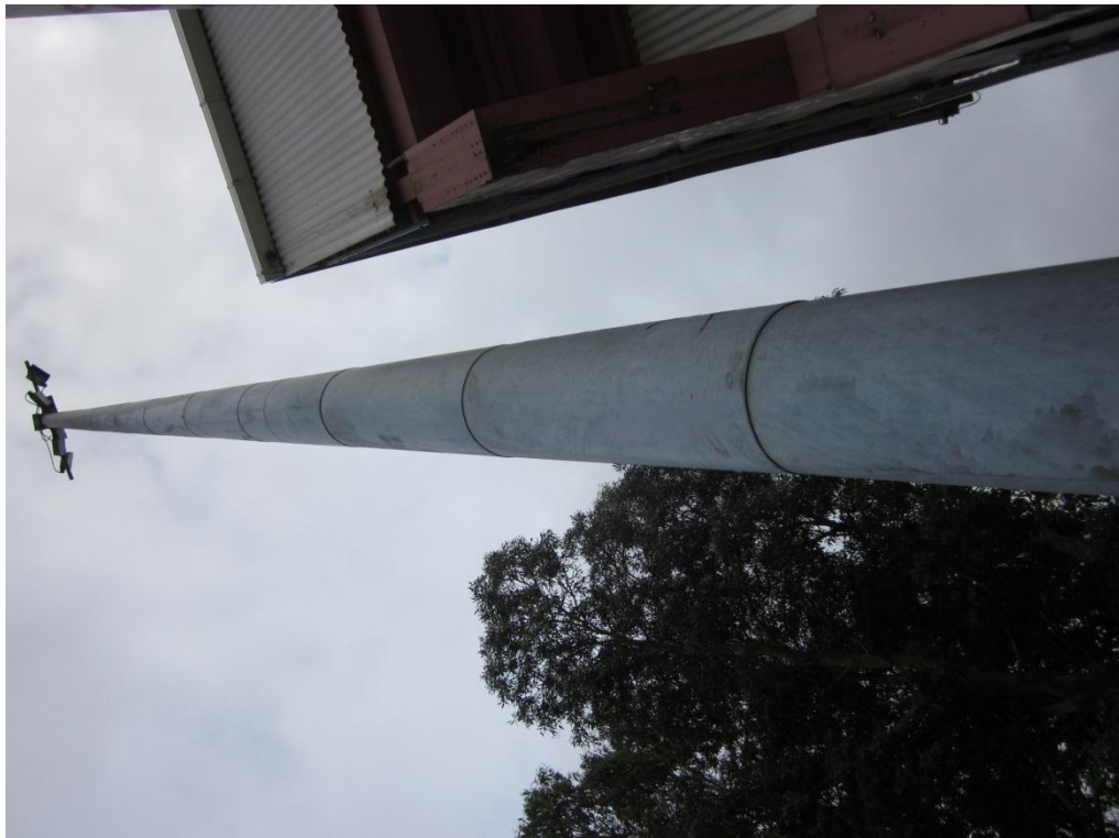
Photograph 2 Lighting tower elevation.
