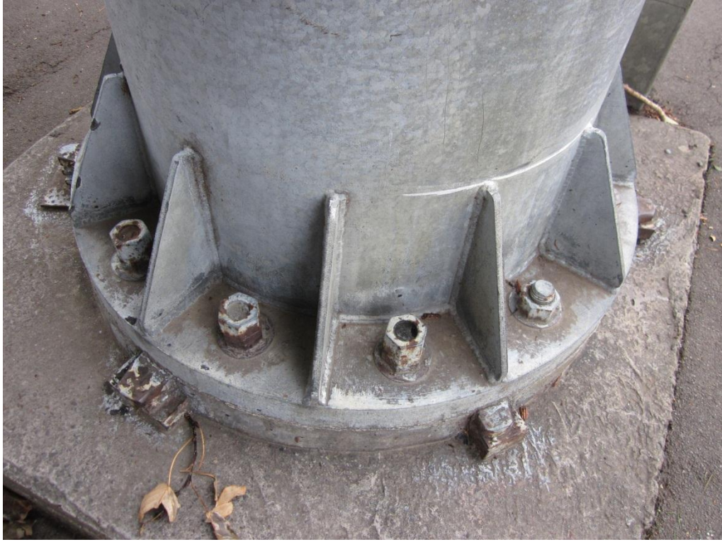
Photograph 3 Lighting tower base showing some rusting of tension bolts.
