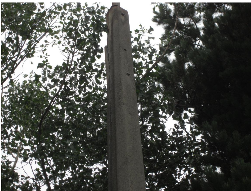
Photograph 11 Cracking to one of the smaller concrete lighting towers around Denton Oval.
