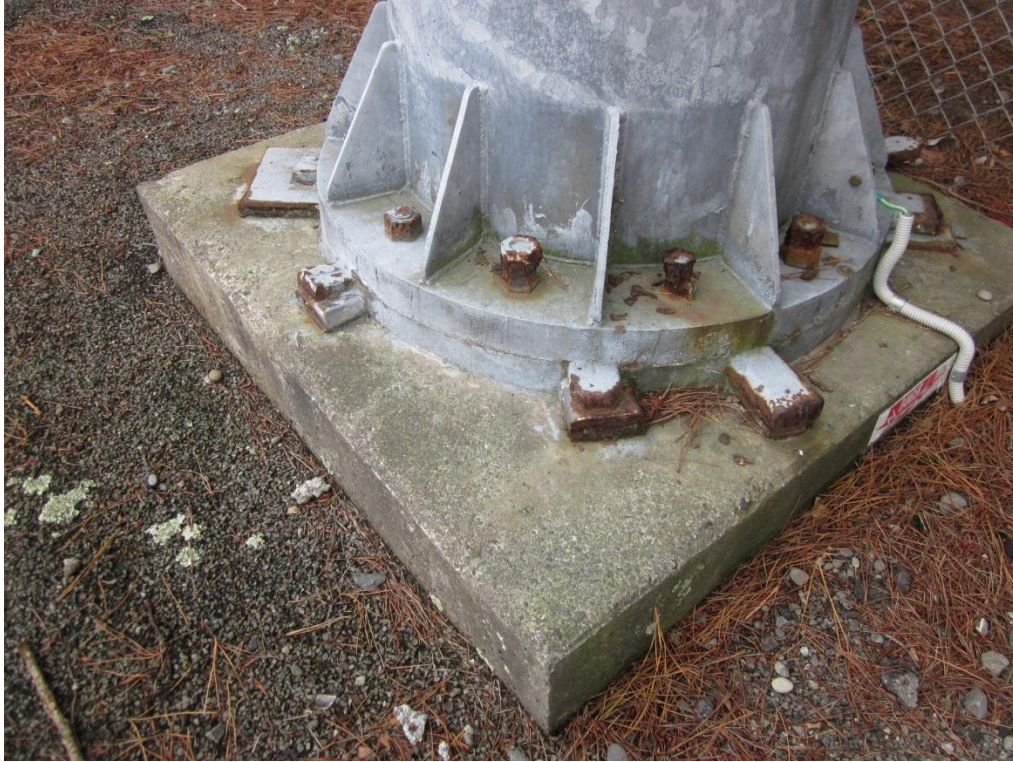
Photograph 9 Base of the North East lighting tower showing severe rusting to tension bolts and respective nuts.
