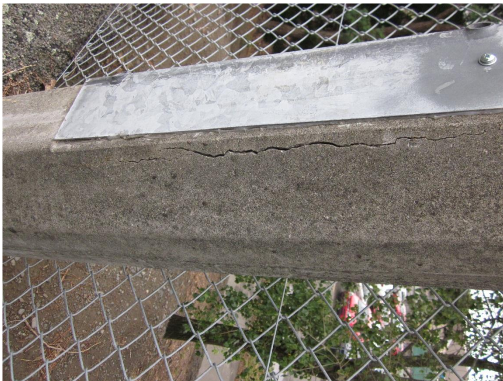
Photograph 11 Cracking to one of the smaller concrete lighting towers around Denton Oval.
