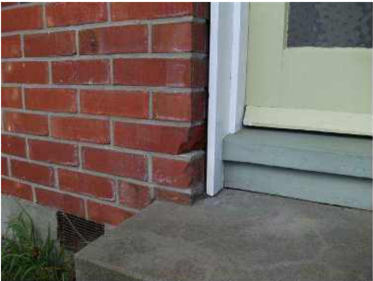
Photo 21: Shearing through Bricks of Exterior Veneer at Back of Flat 5 Looking Northwest
