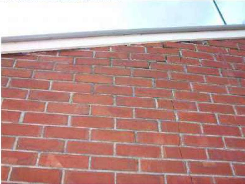
Photo 28: Moderate Vertical Cracking through Brick Veneer at Right Wall and Failing of Gable Bricks of Flat 7 (Photo 5 of 5) Looking East
