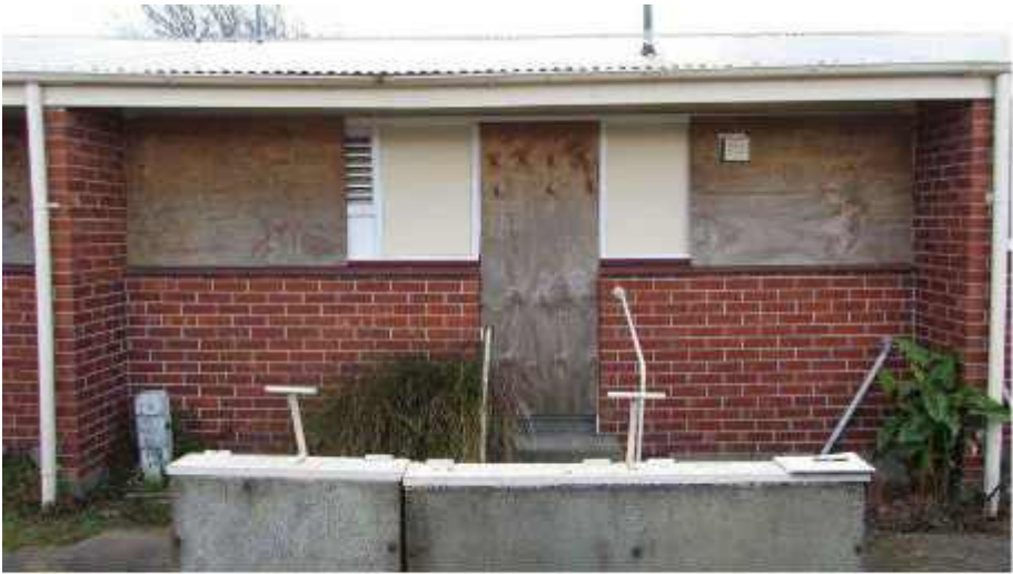
Photo 49: Differential Settlement at Back of Flat 21 Looking Northwest
