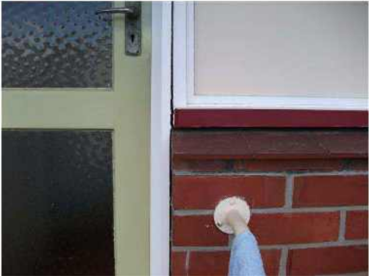
Photo 20: Separation of Doorjamb from Brick Veneer at Back of Flat 5 Looking North-Northwest
