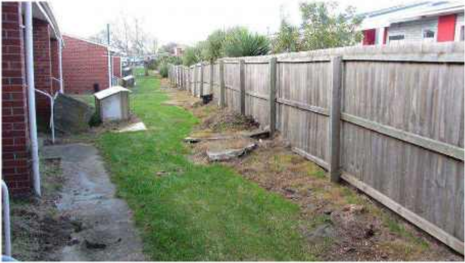
Photo 40: Distortion of Fence along Southern Property Boundary behind Flats Looking Northeast from behind Flat 31
