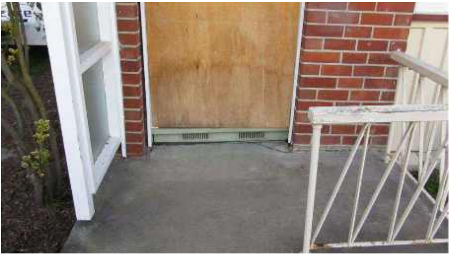
Photo 57: Cracking of Concrete Porch at Back of Flat 28 Looking Southeast
