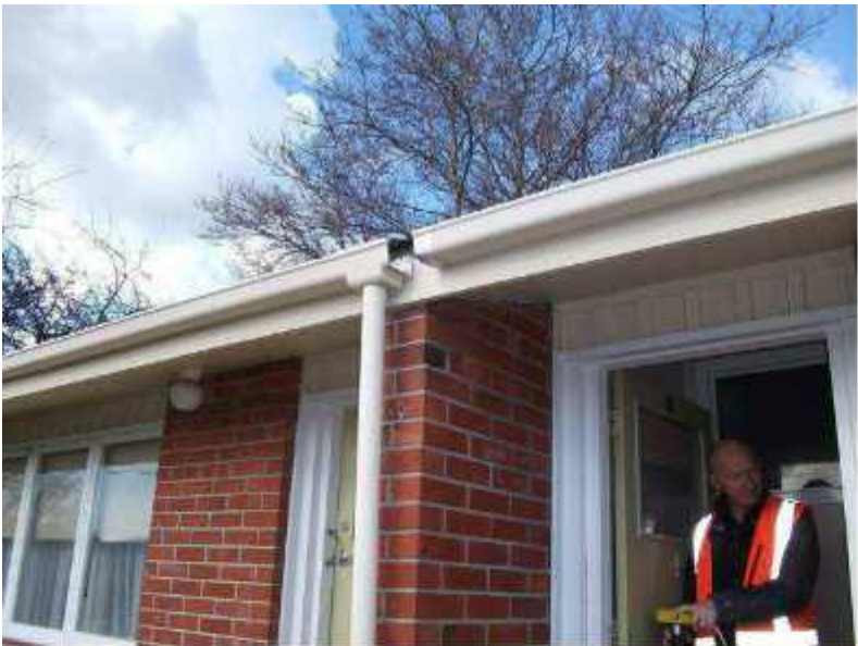
Photo 33: Separation of Downspout Connector from Pilaster and Separation of Gutter Sections at Front of Flats 1 and 3 Looking Southeast
