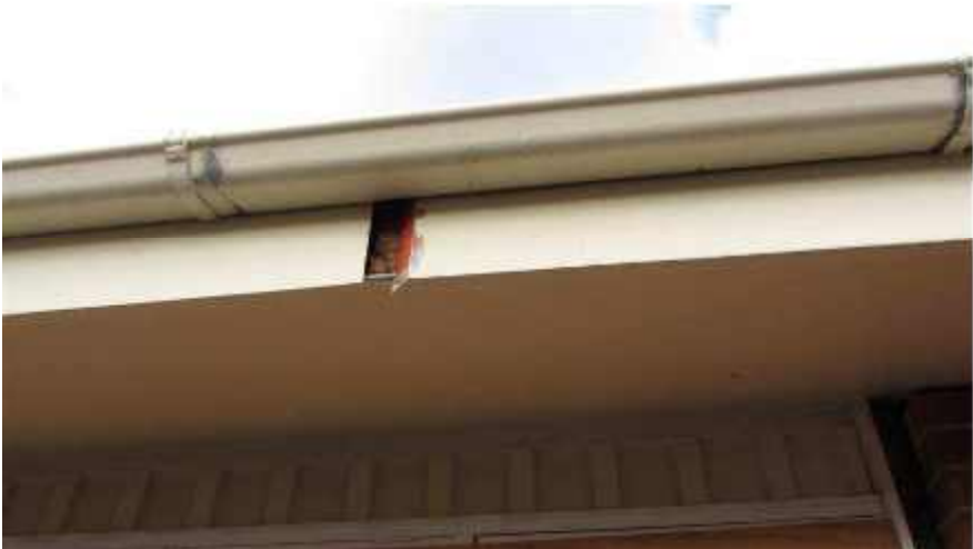
Photo 19: Stretching Separation of Fascia Boards and Movement of Gutter in its Hangar at Front of Flat 27 Looking South
