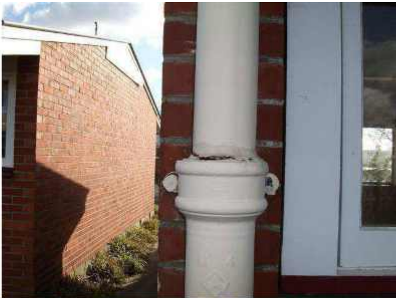
Photo 34: Shearing of Downspout at Rear of Flat 7 Looking Northwest
