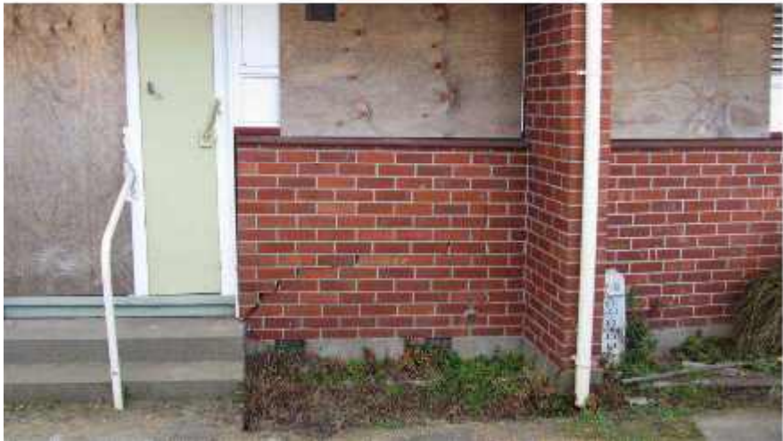
Photo 15: Severe Step Cracking in Brick Veneer at Back of Flat 21 Looking North
