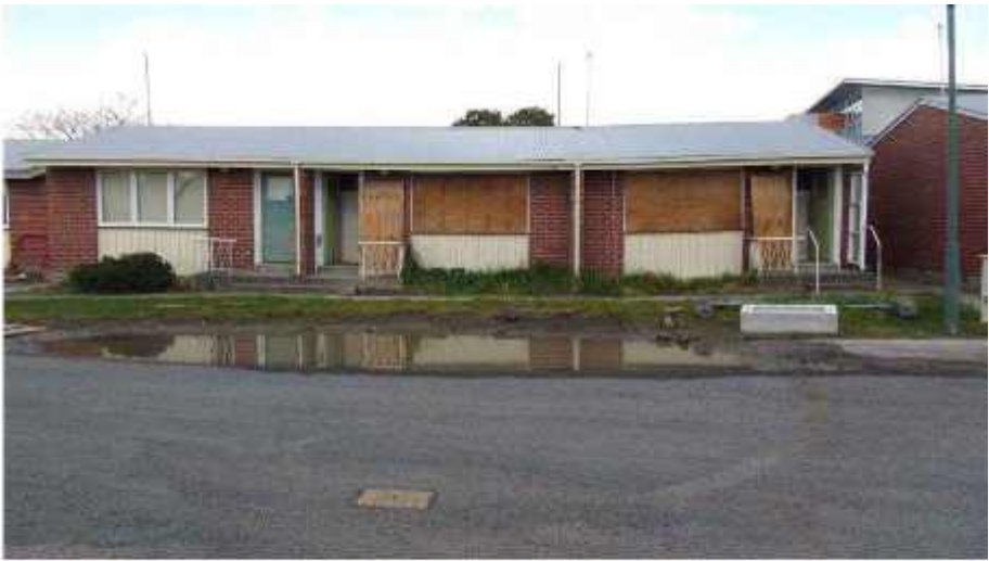
Photo 50: Depression and Differential Settlement at Front of Flats 21 and 23 Looking Southeast
