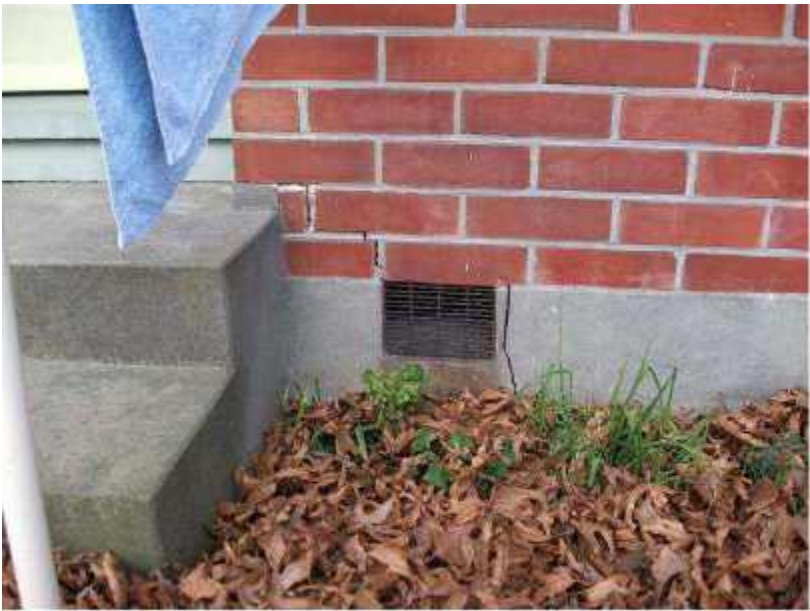
Photo 17: Moderate Crack in Foundation behind Flat 5 Looking North
