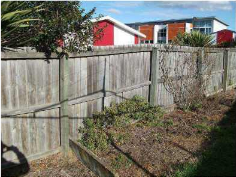
Photo 39: Distortion of Fence along Southern Property Boundary behind Flats 9 and 11 Looking Southwest
