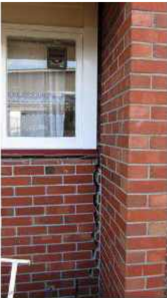
Photo 30: Severe Stretching of Walls at Rear of Flats 27 and 29 Looking North (Photo 1 of 2)
