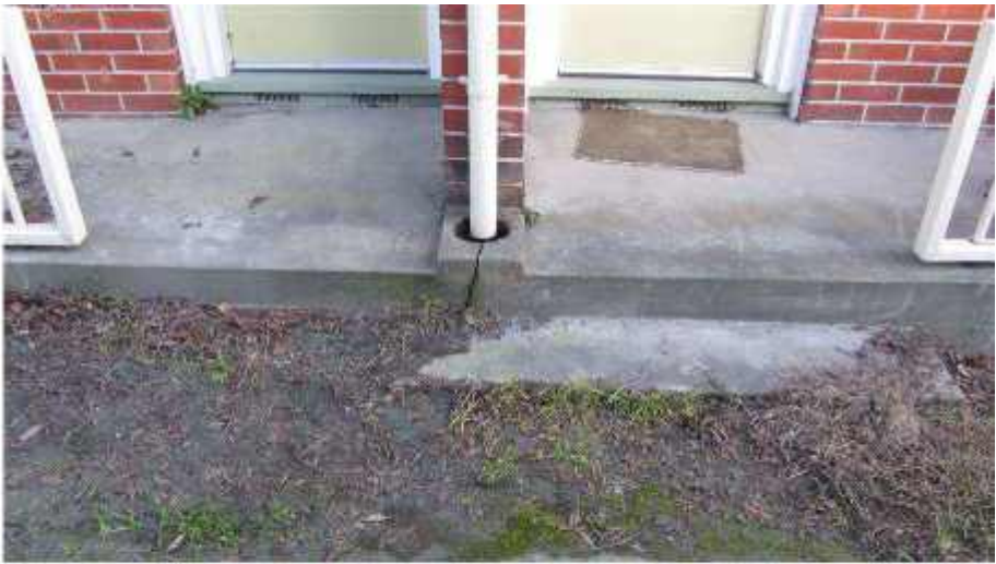
Photo 58: Cracking of Concrete Porch at Back of Flats 22 and 24 Looking Southeast
