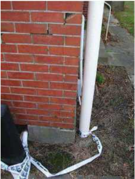
Photo 23: Shearing through Bricks of Exterior Veneer and Minor Vertical Cracking through Bricks in Corner Exterior Wall at Back of Right Wall of Flat 7 Looking East
