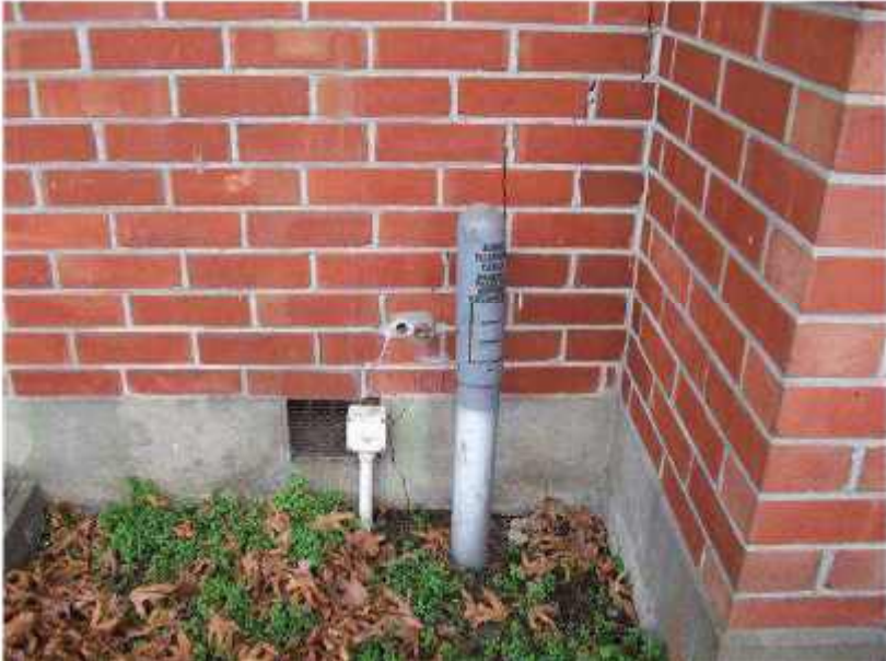
Photo 12: Bottom Portion of Medium Stepping Crack in Brick Veneer behind Flat 5 Looking North
