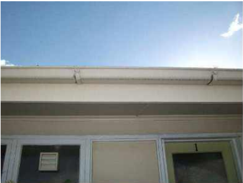
Photo 41: Movement of Gutter in its Hangar at Back of Flat 1 Looking Northwest
