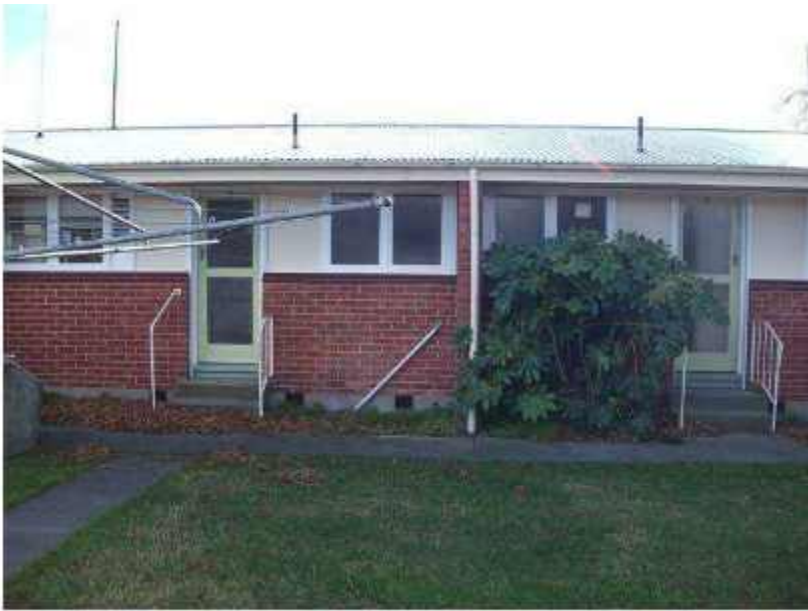
Photo 18: Stretching Separation of Fascia Boards at Back of Flats 1 and 3 Looking Northwest
