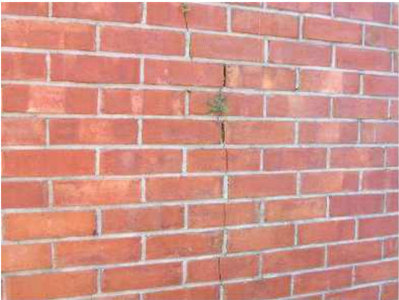
Photo 25: Moderate Vertical Cracking through Brick Veneer at Right Wall of Flat 7 (Photo 2 of 5) Looking Southeast
