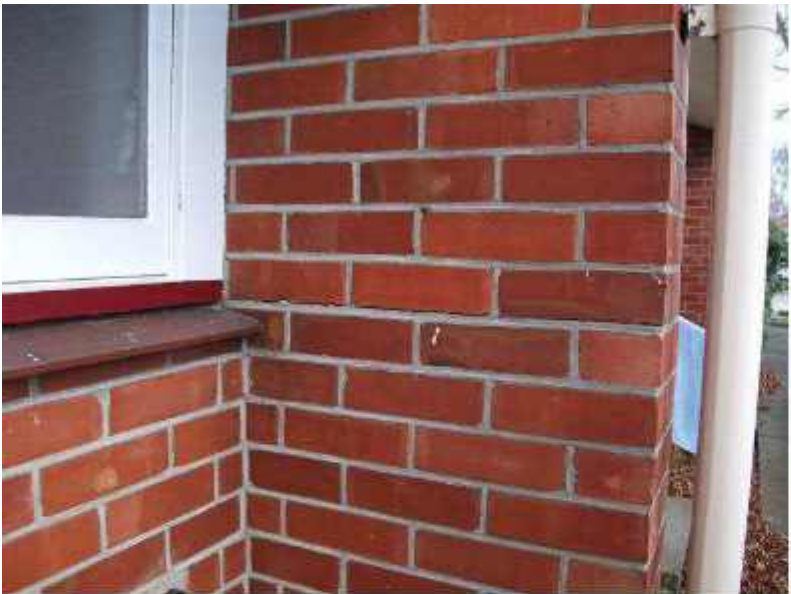
Photo 29: Tension Cracking of Pilaster between Rear of Flats 5 and 7 Looking East
