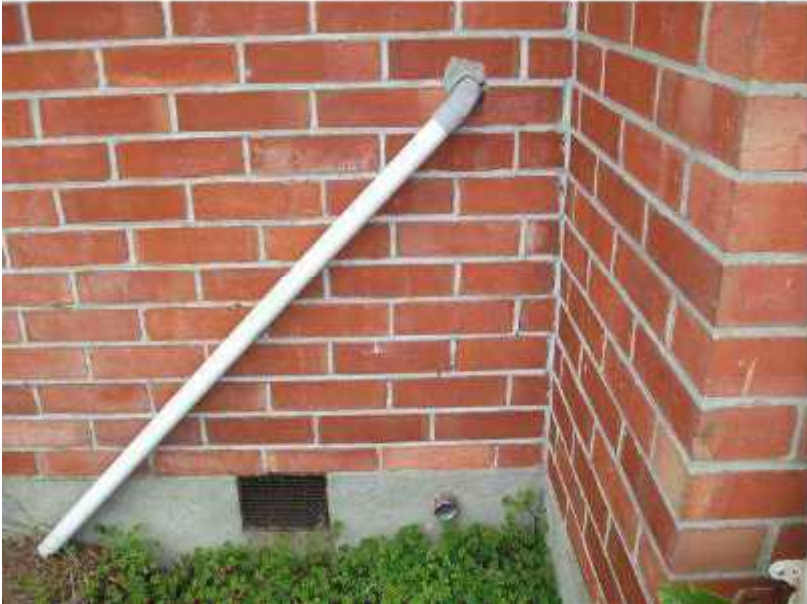
Photo 11: Small Stepping Crack in Brick Veneer behind Flat 3 Looking North
