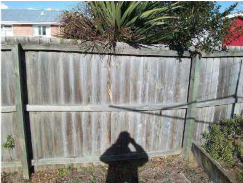
Photo 38: Distortion of Fence along Southern Property Boundary behind Flats 9 and 11 Looking Southeast
