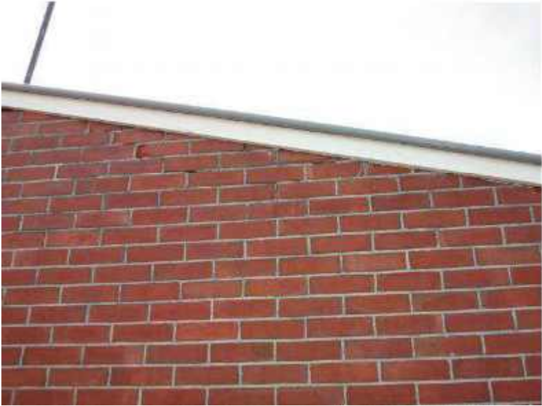
Photo 43: Cracking of Gable at Top of Right Wall of Flat 7 Looking Northeast
