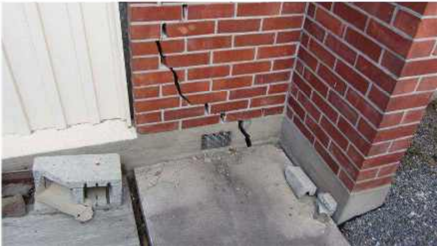
Photo 16: Severe Stepping Crack, Shearing Through Brick in Exterior Veneer and Cracking through Foundation at Front of Flat 27 Looking South
