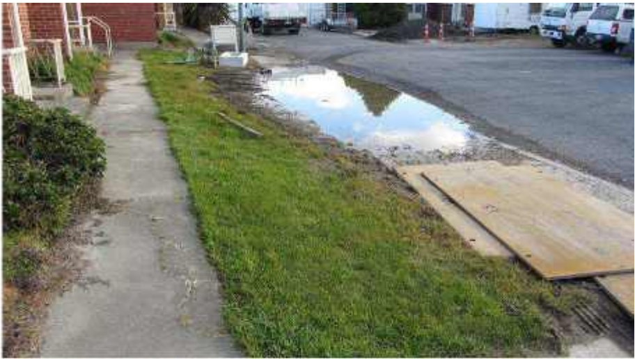
Photo 54: Depression, Differential Settlement and Distortion of Concrete Footpath and in Cresselly Place in Front of Flats 19, 21, 23 and 25 Looking Southwest
