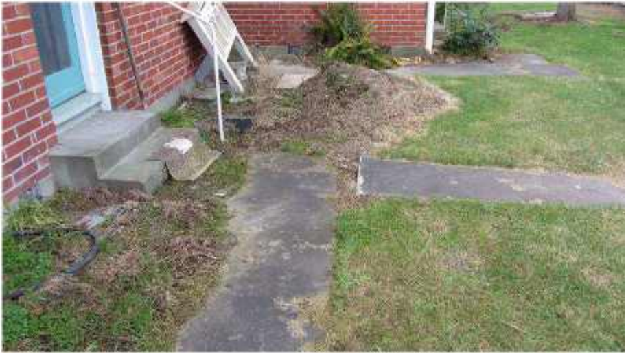
Photo 44: Differential Movement of Concrete Footpaths behind Flat 19 Looking Northeast
