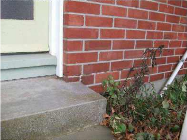
Photo 35: Shearing through Grout between Bricks of Exterior Veneer at Back of Flat 7 Looking North
