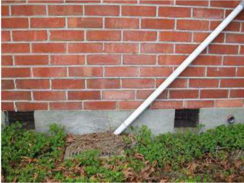
Photo 36: Shearing through Grout between Bricks of Exterior Veneer at Back of Flat 1 Looking Northeast
