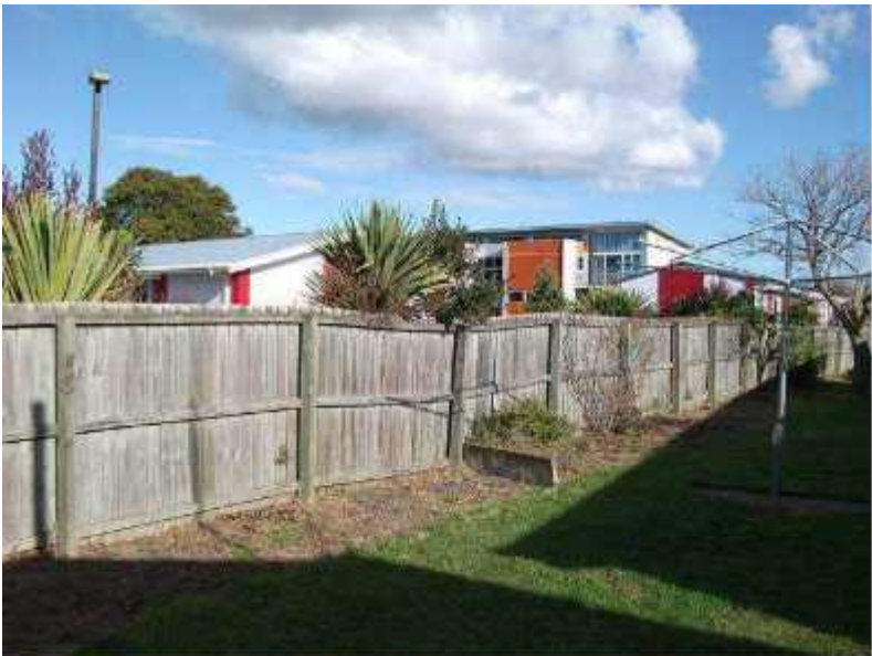
Photo 37: Distortion of Fence along Southern Property Boundary behind Flats 9 and 11 Looking Southwest
