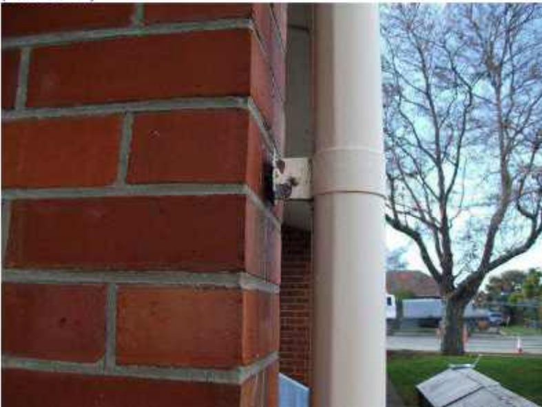
Photo 32: Separation of Downspout Connector from Pilaster at Rear of Flats 5 and 7 Looking East
