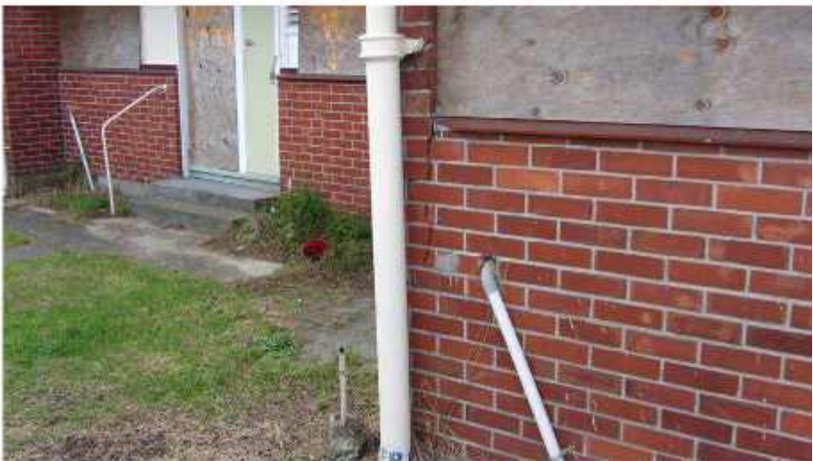
Photo 22: Shearing through Bricks of Exterior Veneer and Minor Vertical Cracking through Bricks in Corner Exterior Wall at Back of Flat 23 Looking West
