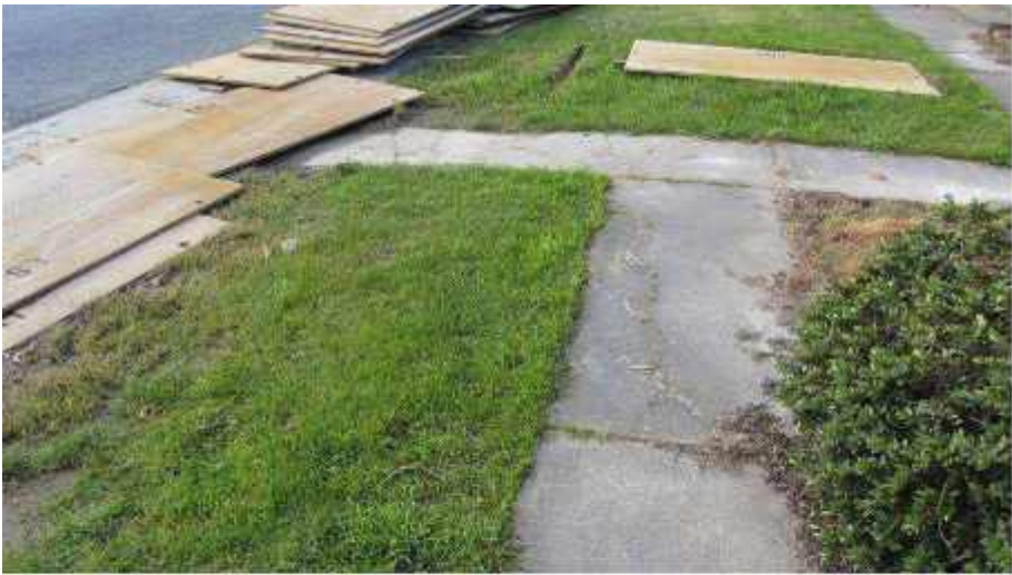
Photo 53: Depression, Differential Settlement and Distortion of Concrete Footpath in Front of Flats 23 and 25 Looking Northeast
