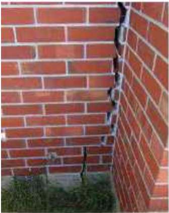
Photo 29: Tension Cracking of Pilaster between Rear of Flats 5 and 7 Looking East
