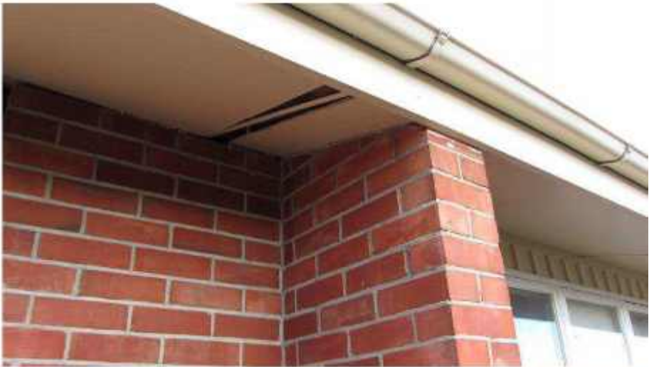
Photo 42: Movement of Gutter in its Hangar and Separation of Eave Joint at Front of Flat 29 Looking South-Southwest
