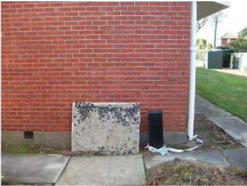
Photo 14: Major Stepping Crack in Brick Veneer in the Back Portion of the Right Wall of Flat 7 Looking East
