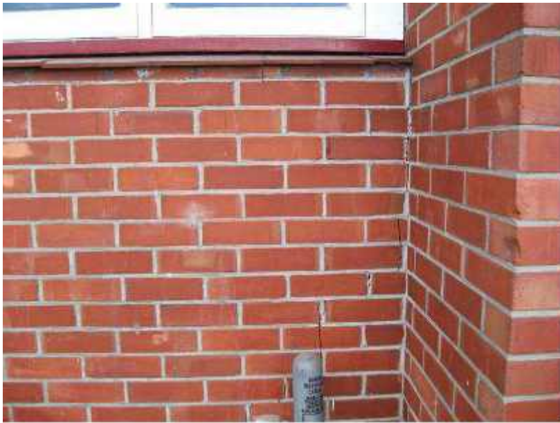
Photo 13: Top Portion of Medium Stepping Crack in Brick Veneer behind Flat 5
