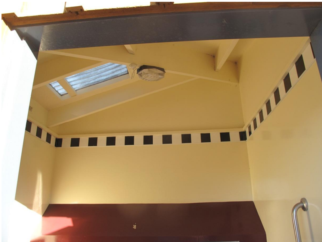
Photograph 6 Roof structure with purlins and timber beam visible.
