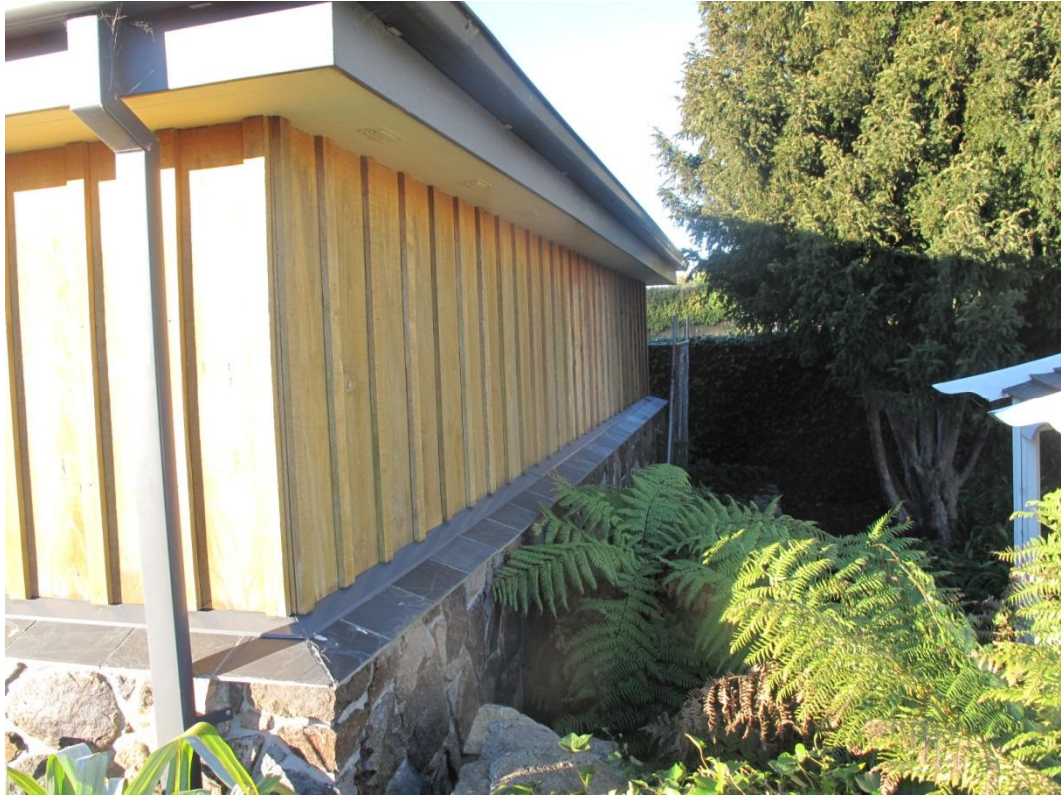
Photograph 9 The south wall shows the timber panelling above the stone and mortar veneer.
