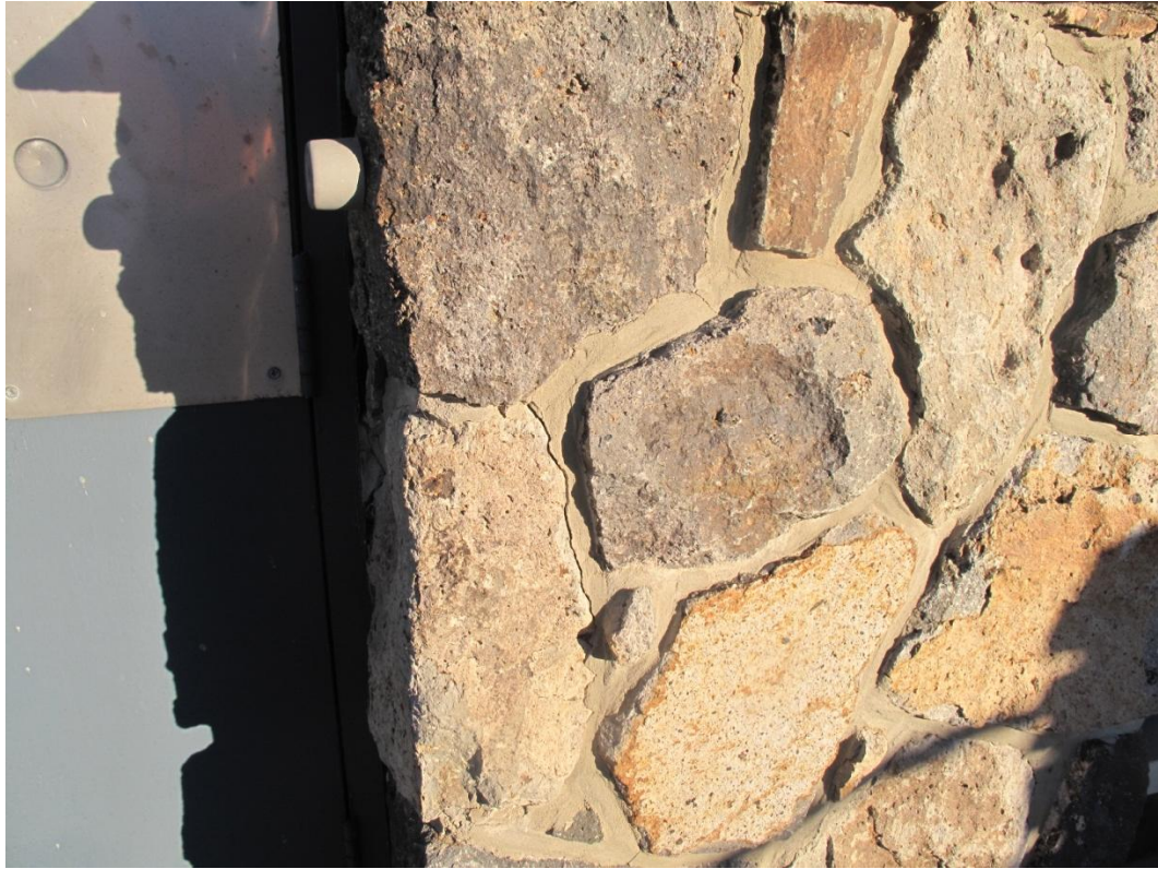
Photograph 5 Minor cracks in the mortar on the north side of the toilet block.
