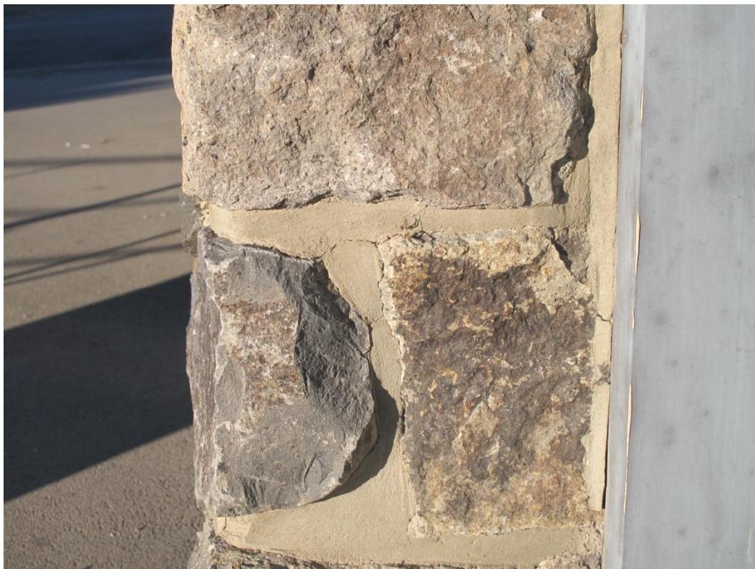
Photograph 4 Minor cracks in the mortar on the north side of the toilet block.
