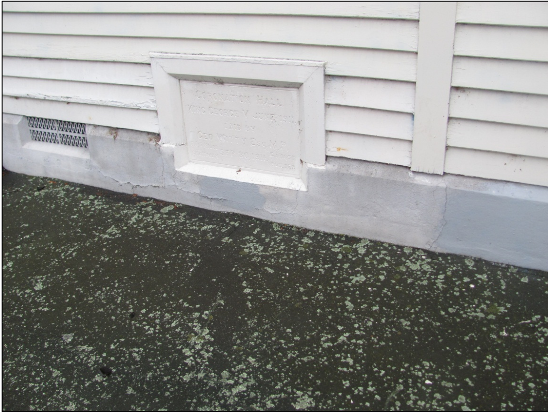
Photograph 7: View of the hairline cracks in the concrete footings on the northeast corner of the hall.
