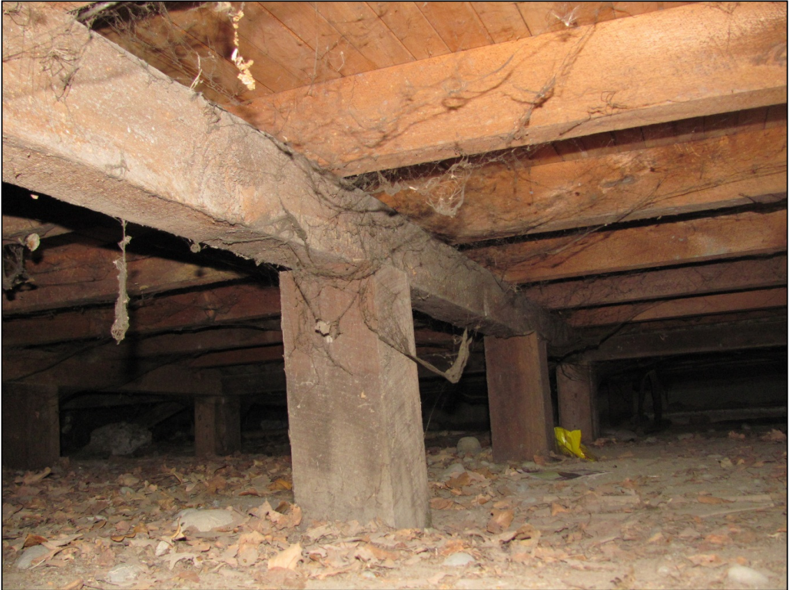
Photograph 4: View of the 200mm square timber piles where the southern half of the structure stands on the gentle slope.
