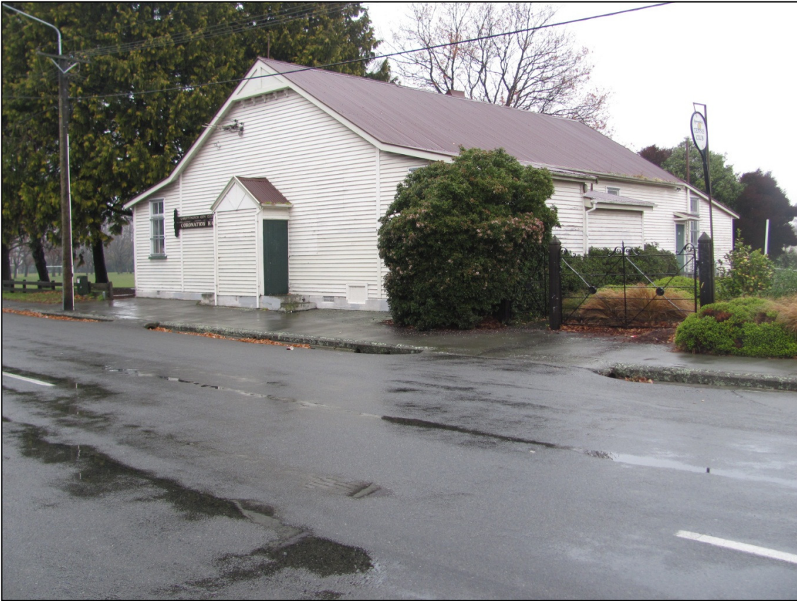
Photograph 1: View of north facing side of Coronation Hall.
