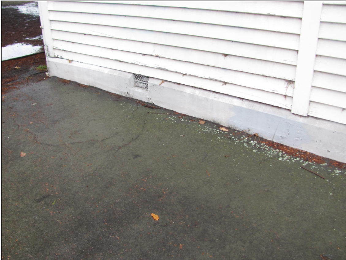
Photograph 6: View of the hairline cracks on the concrete footings on the northeast facing side of the hall.
