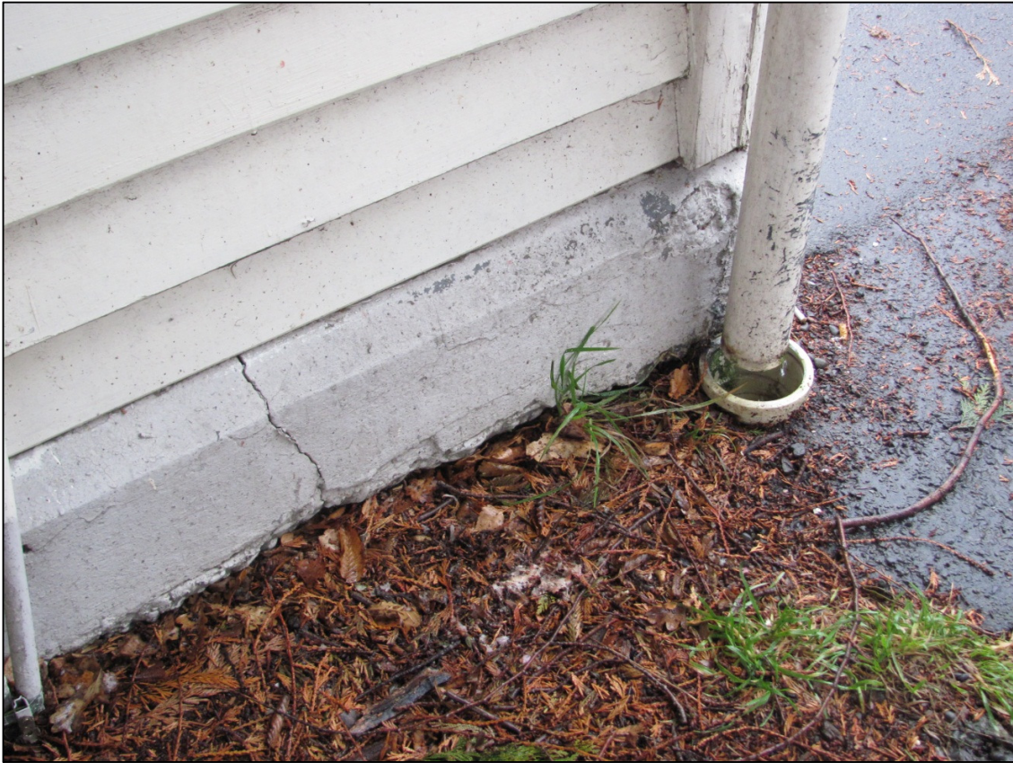
Photograph 5: View of the 3mm wide crack in the concrete footings on the eastern corner of the hall.
