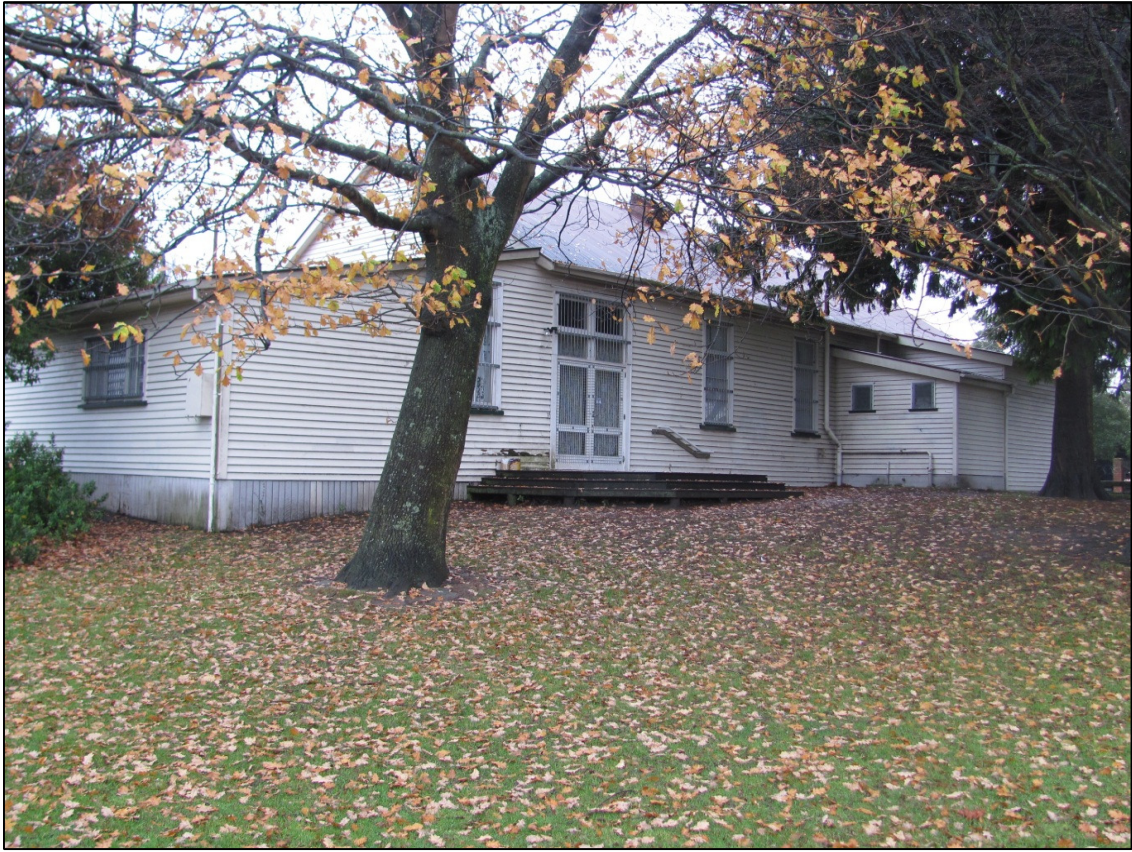
Photograph 3: View of south facing side of Coronation Hall.
