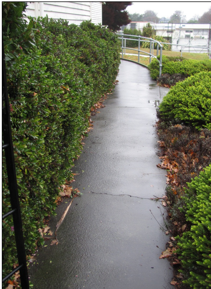
Photograph 8: View of the two 5mm wide cracks in the asphalt pavement located by the northwest side of the hall.
