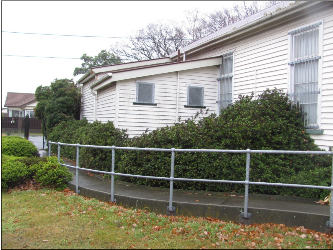
Photograph 9: View of the dense growth of shrubbery along west facing side of the hall obscures the concrete strip footings.
