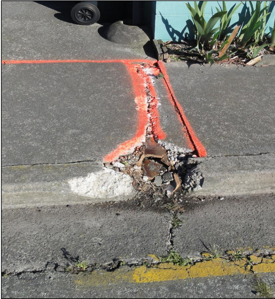
Photo 9 Broken 100 mm diameter clay drainage pipe east of Unit No. 39
