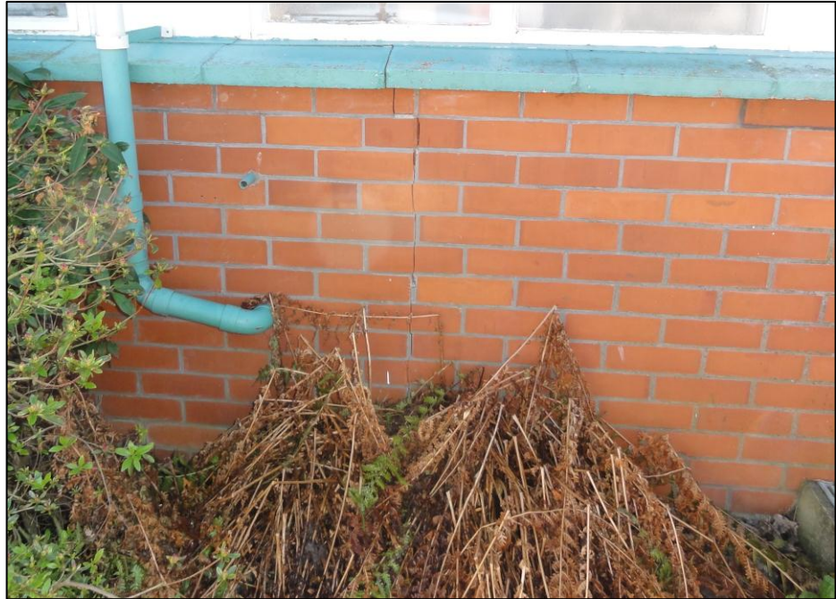
Photo 11 Crack through mortar and bricks from floor slab to window. No cracking observed in floor slab. (South wall of No. 42).
