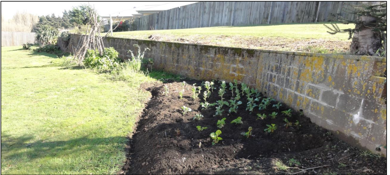
Photo 14 Retaining wall at north of site. No obvious visual indication of movement
