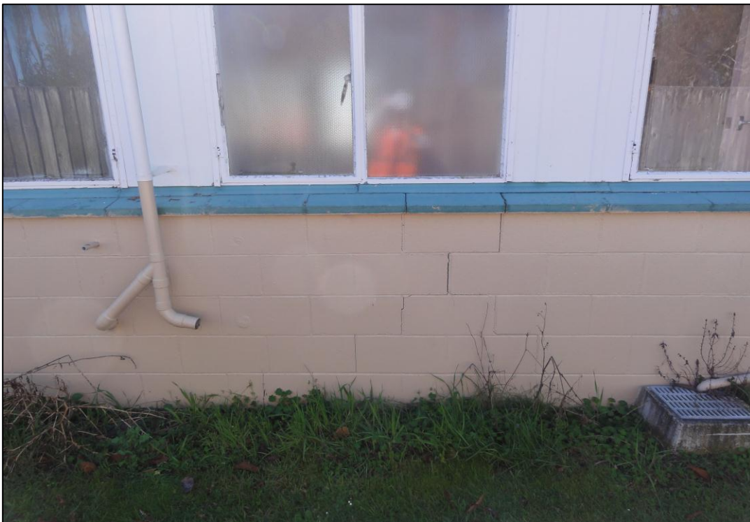
Photo 4 Step crack in the mortar of concrete masonry wall between Unit No. 15 (left) and Unit No. 14 (right)
