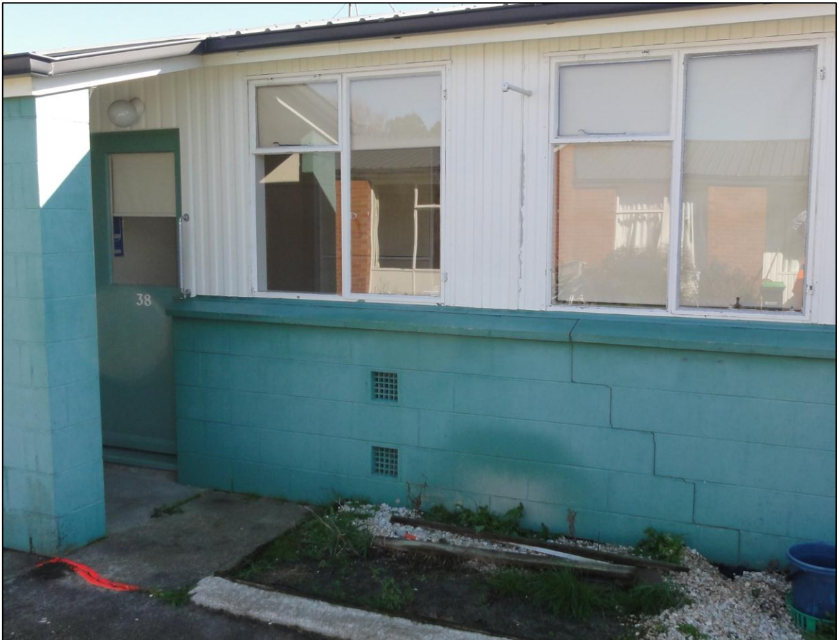
Photo 7 Step crack in mortar, south side of No. 38
