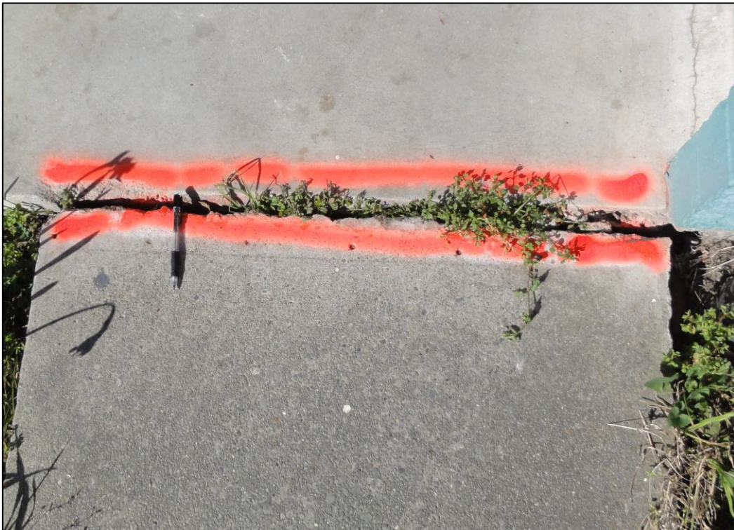
Photo 5 Footpath displacement of approx. 40 mm to the south of No. 11
