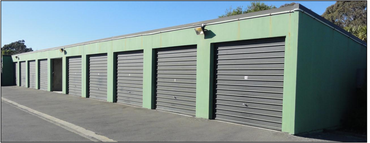
Photo 13 Garage Block No obvious visible indication of movement
