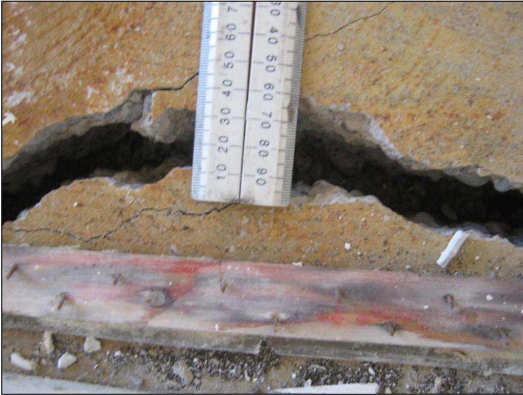
Photo 3 Cracked floor slab inside Unit No. 12 (20 mm wide)
