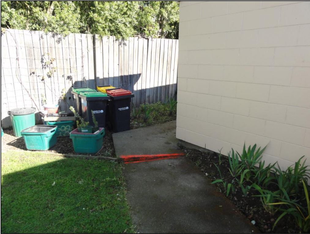
Photo 1 – Footpath displacement at SE corner of Unit No. 5
