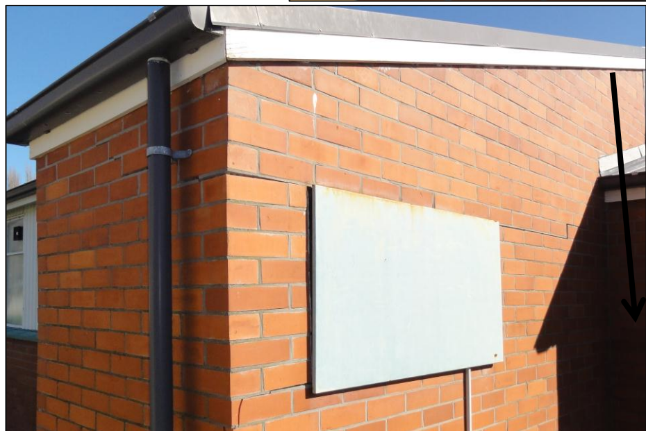
Photo 12 and 12a Cracking in mortar from downpipe to doorway on the right. Unit No. 41 porch (Unit No 42 door on right).
