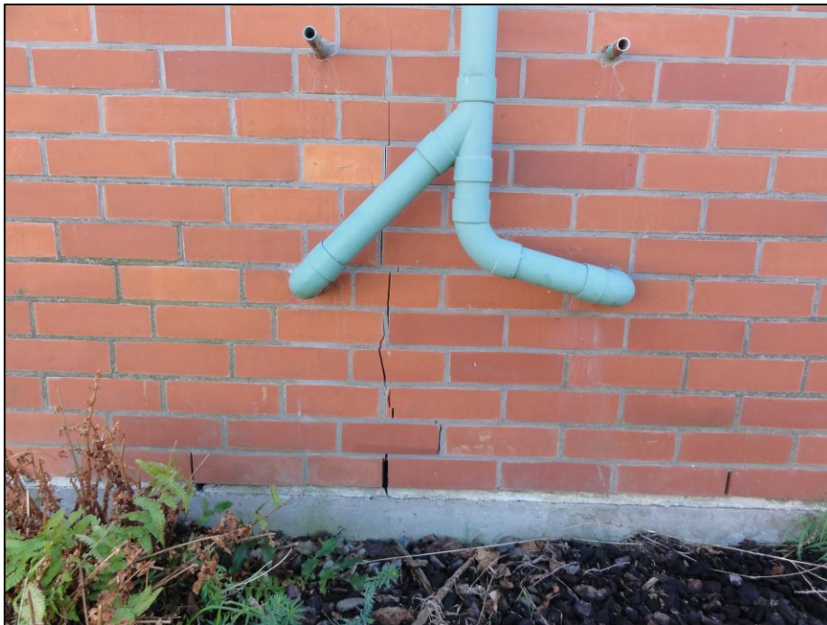
Photo 10 Crack through mortar and bricks. Note intact floor slab. Unit No. 40 Left, Unit No. 41 Right.
