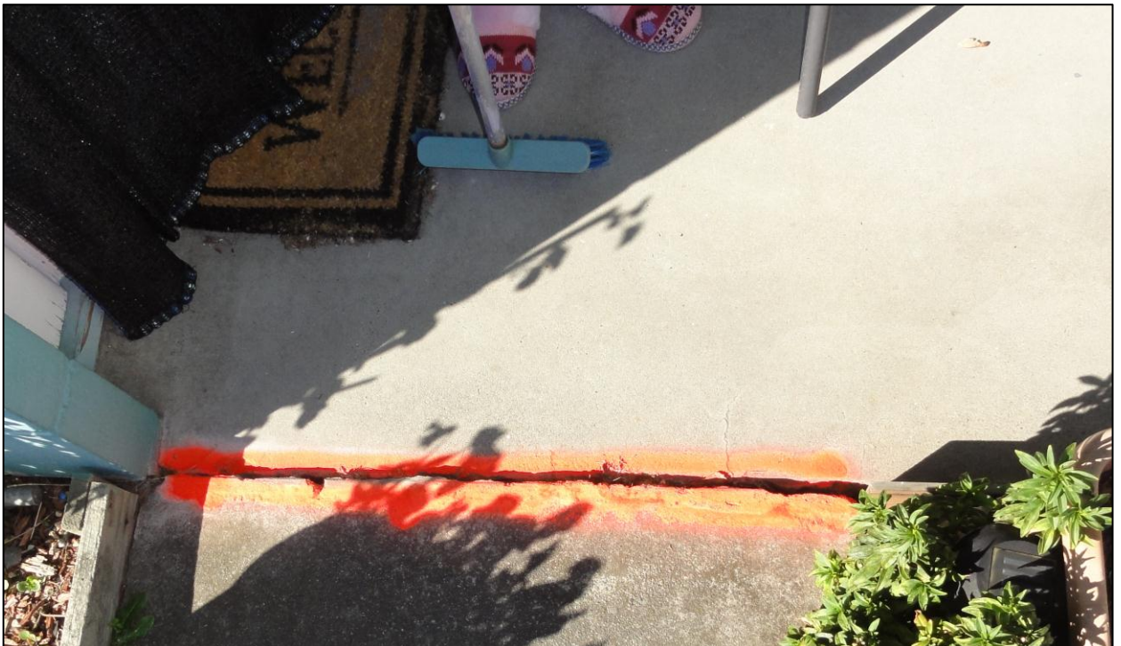
Photo 7 Step crack in mortar, south side of No. 38
