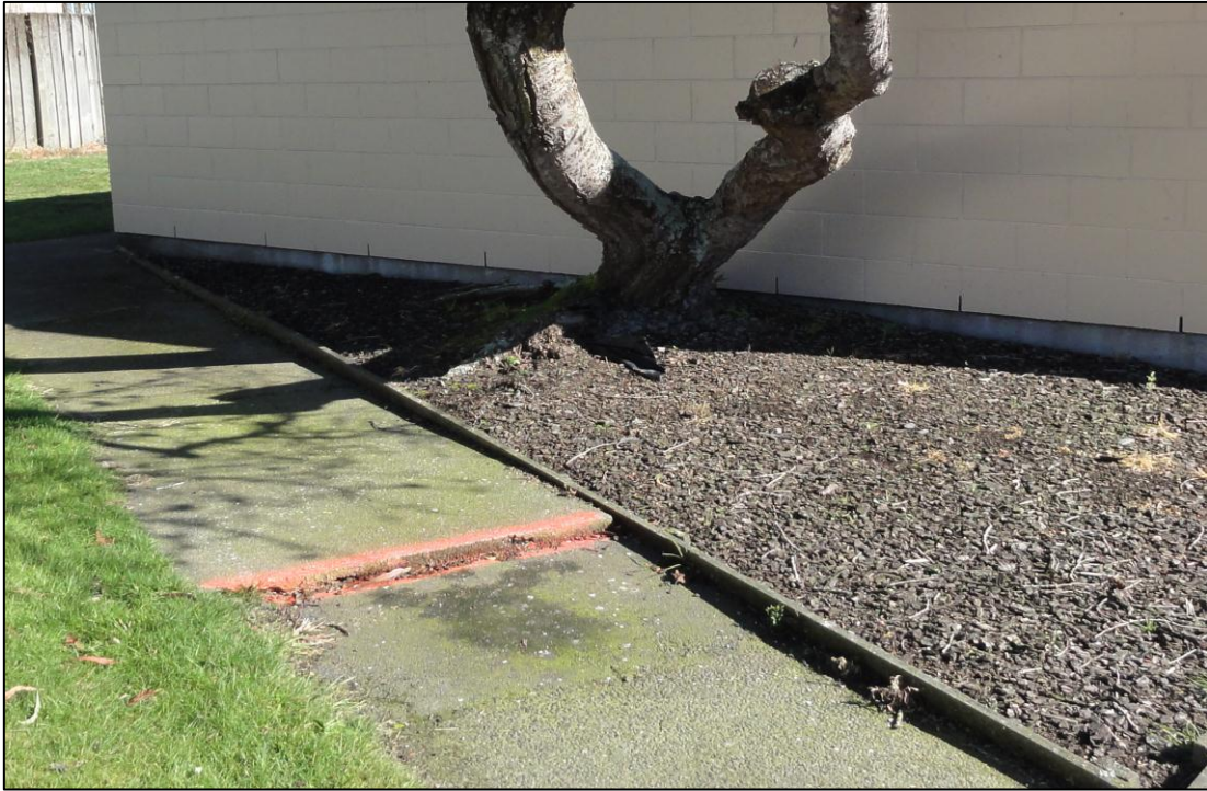
Photo 5 Footpath displacement of approx. 40 mm to the south of No. 11
