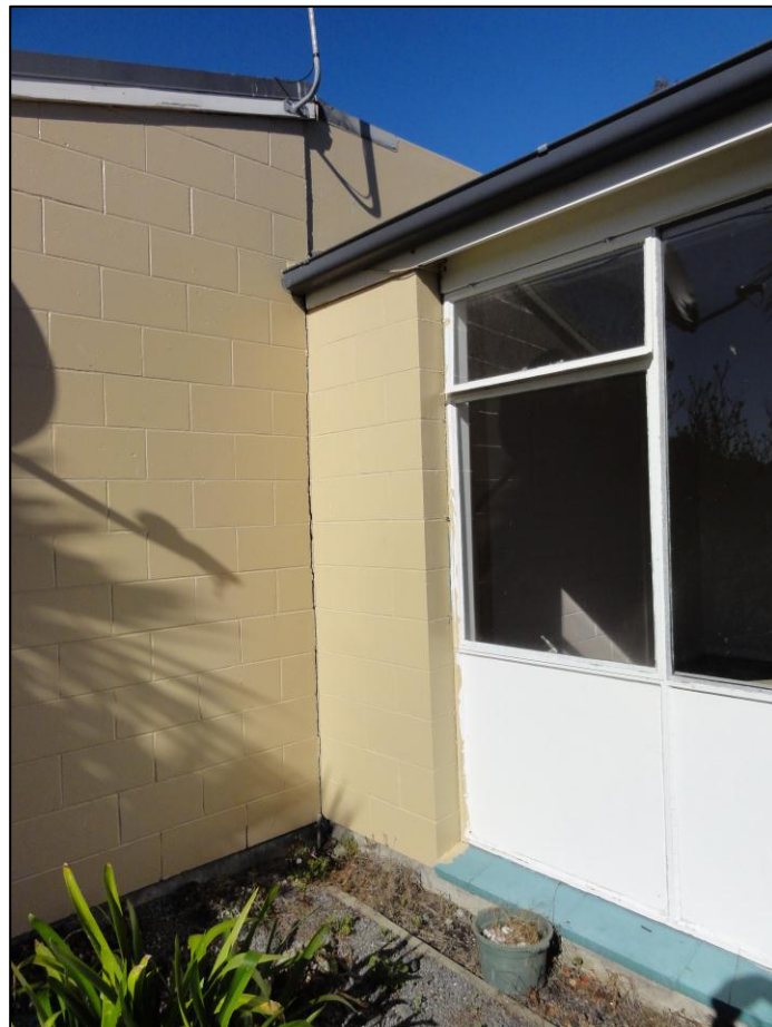
Photo 2 Vertical crack between No. 12 on left and No. 14 on right
