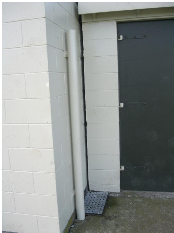
Photograph 8 Separation between the pavilion building and adjacent garage
