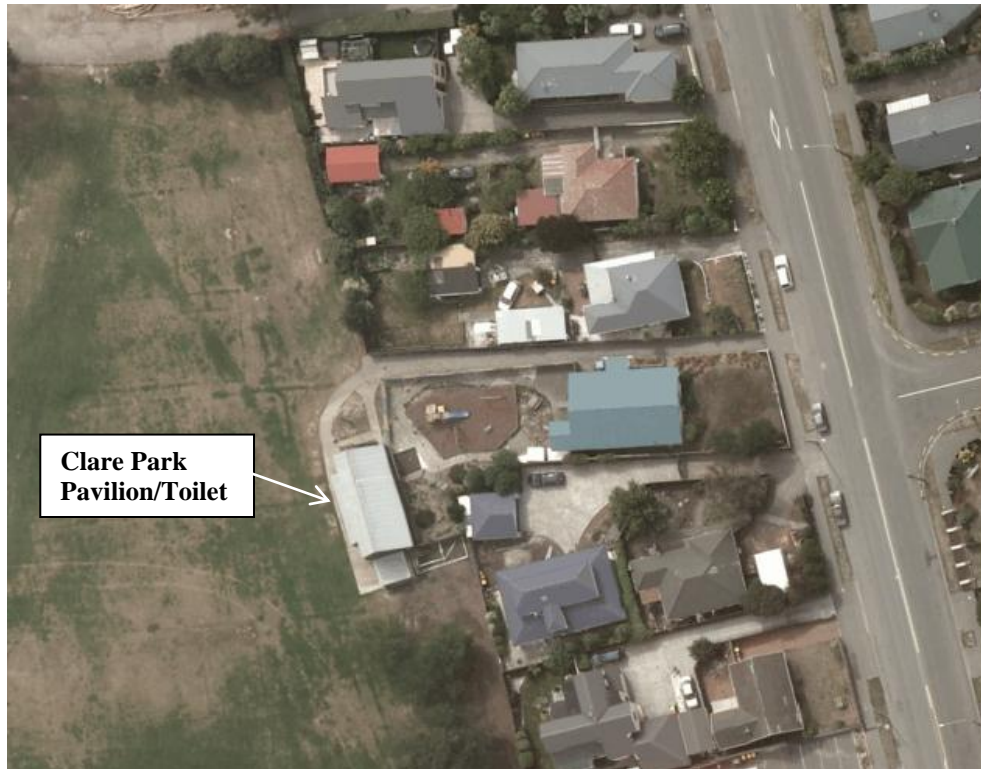
Figure 4 Post February 2011 Earthquake Aerial Photography 3
