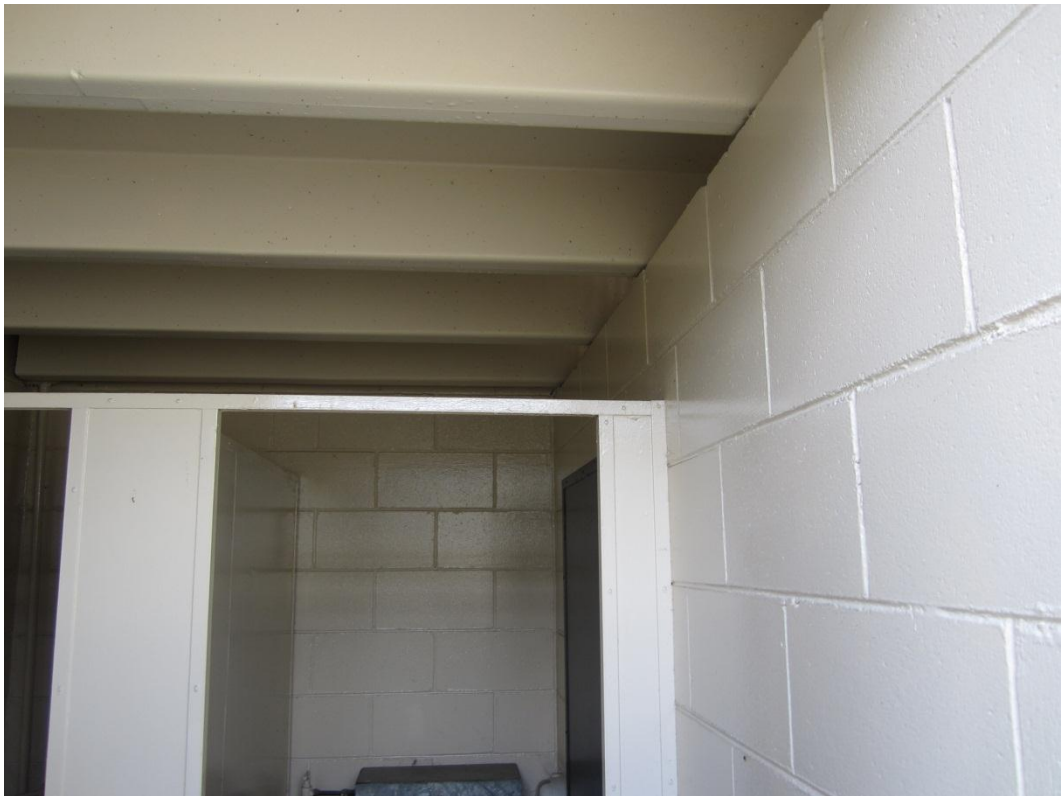
Photograph 5 Overhanging double tee units
