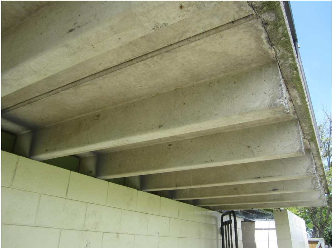
Photograph 5 Overhanging double tee units
