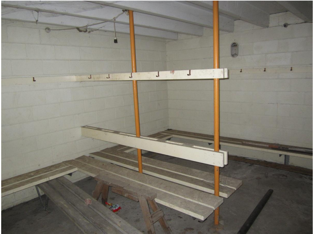
Photograph 7 View of internal masonry walls and double tee units
