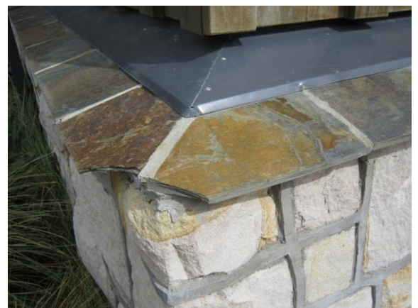
Photo 8: Suspected impact damage to stonework veneer on the southwest corner of the building
