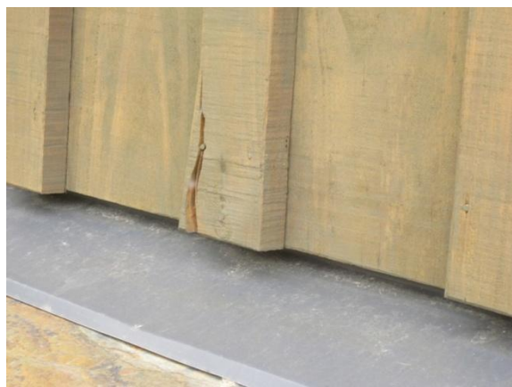
Photo 7: Cracking along the grain of external timber wall cladding elements
