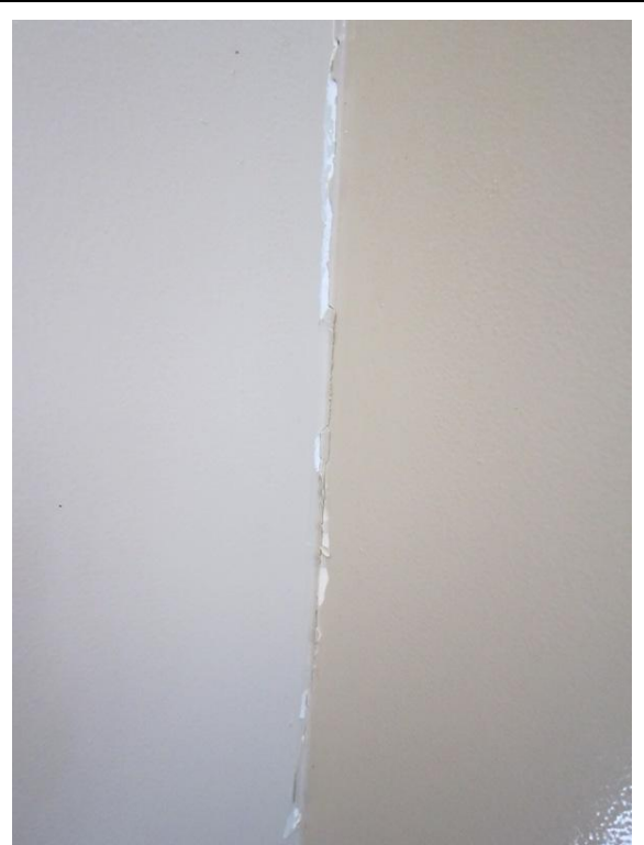
Photo 10: Tearing of internal wall layout at joints (typical)
