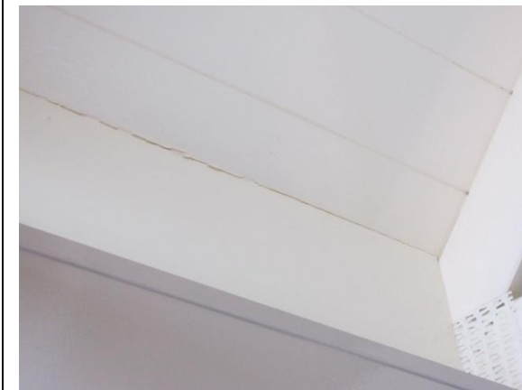
Photo 11: Gap opening up between internal timber cladding elements on the southern side of the building
