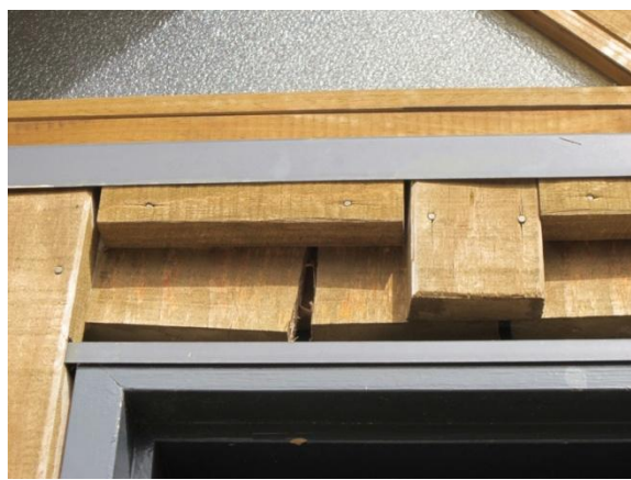
Photo 5: Cracking along the grain of external timber wall cladding elements
