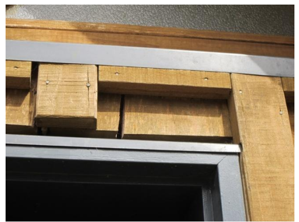
Photo 6: Cracking along the grain of external timber wall cladding elements
