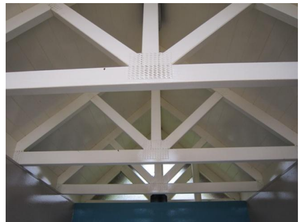
Photo 12: Timber roof trusses
