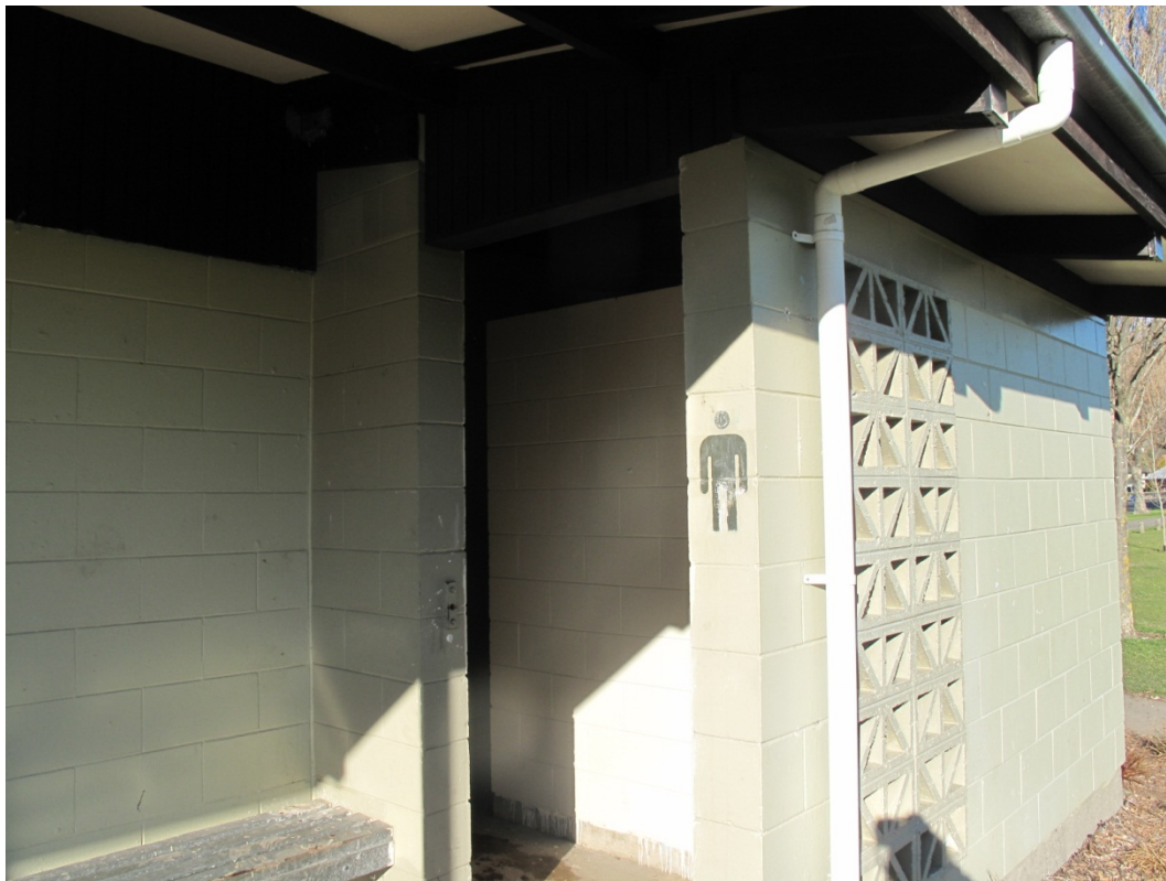
Photograph 10 Toilet area on the southern end of the building.
