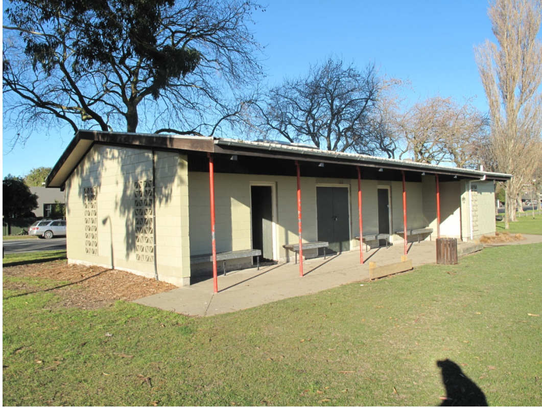
Photograph 3 View of the canopy and pavilion from the north west.
