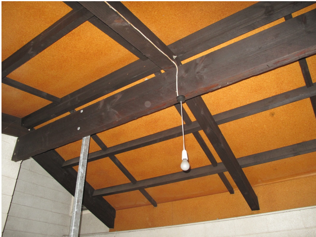
Photograph 4 Purlins, rafters and beams supporting the roof.
