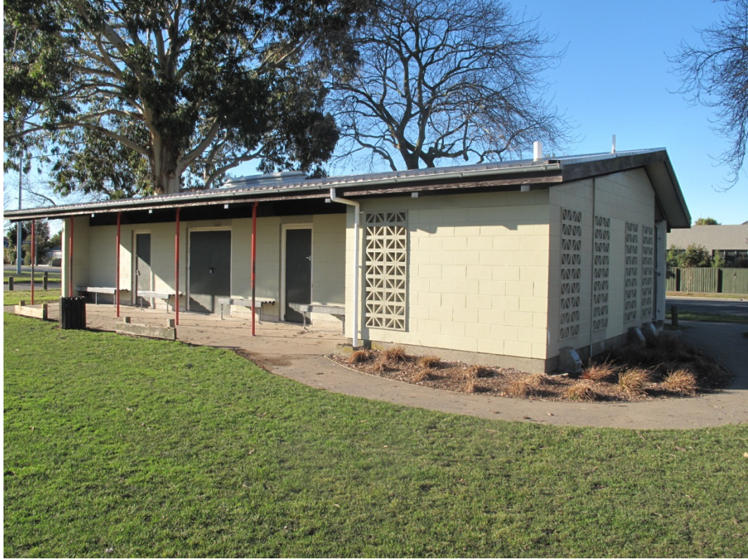
Photograph 1 South west elevation.
