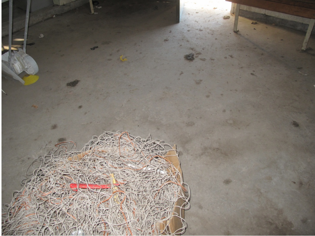
Photograph 9 No visible damage to the slab on grade flooring.
