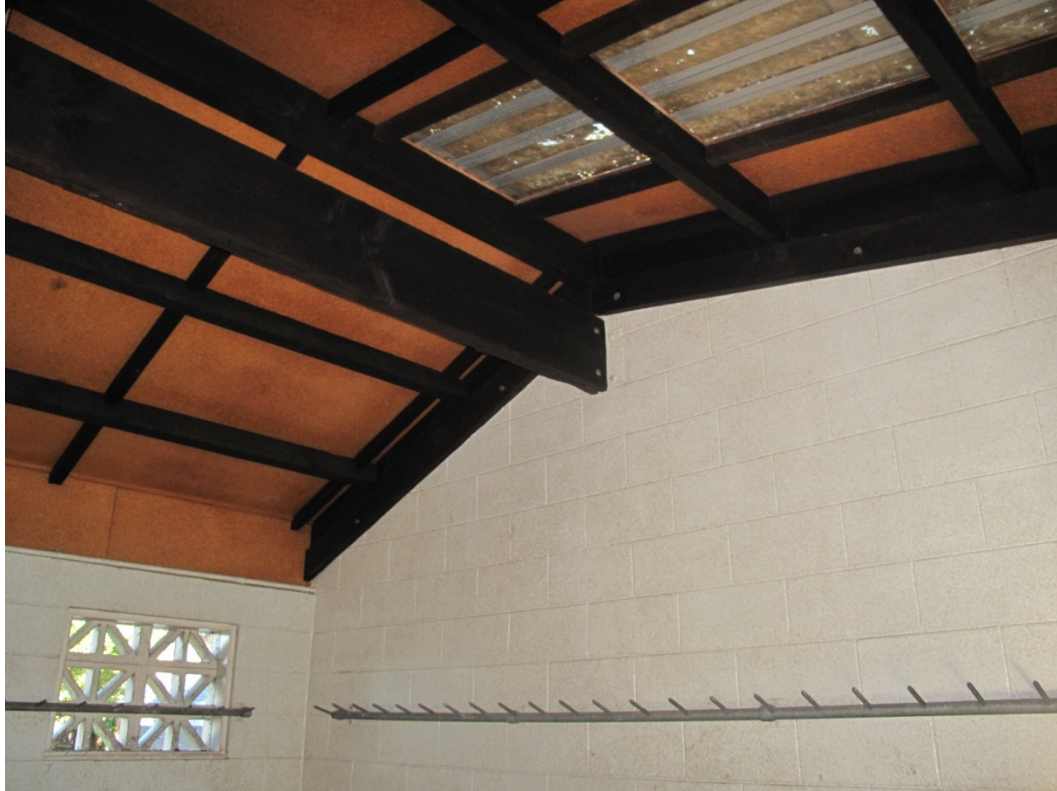
Photograph 5 Eaves beam and central beam bolted to the southern end of the block.
