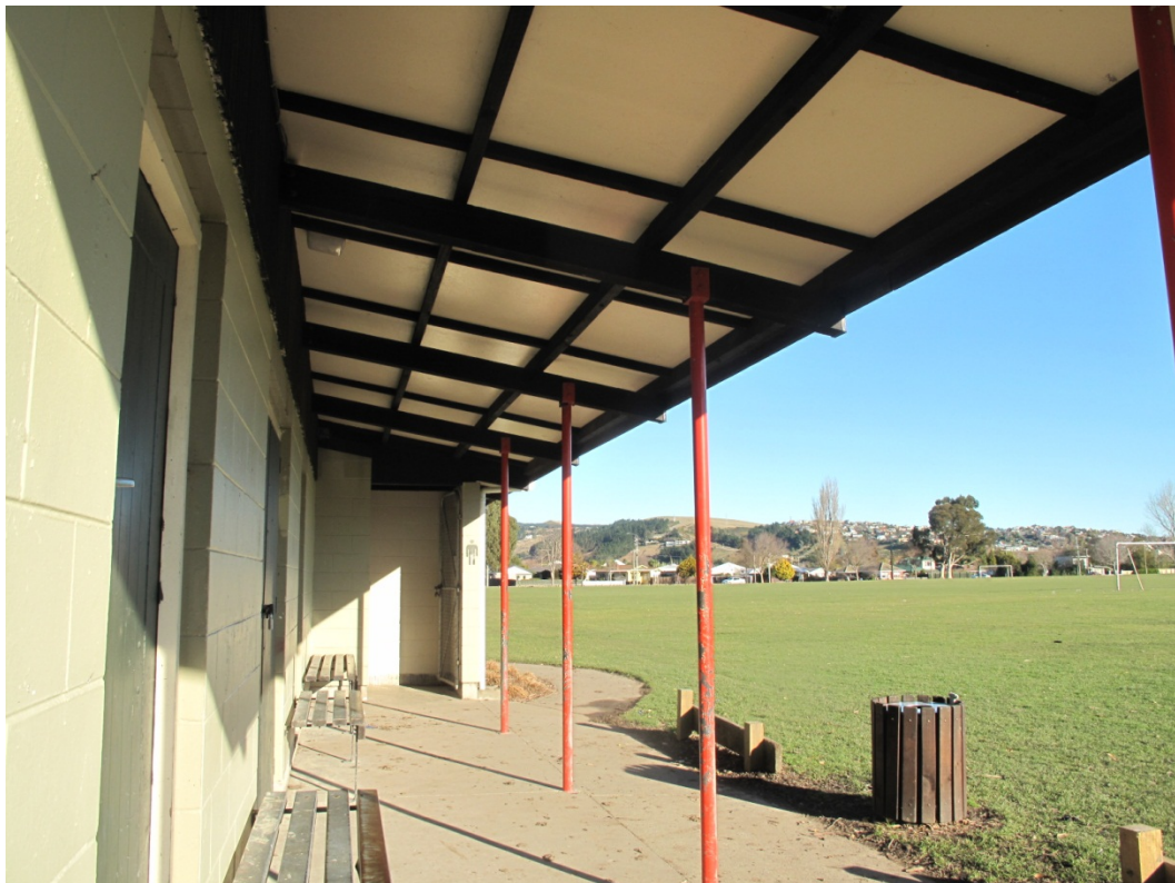
Photograph 6 Steel support posts holding up the canopy rafters.
