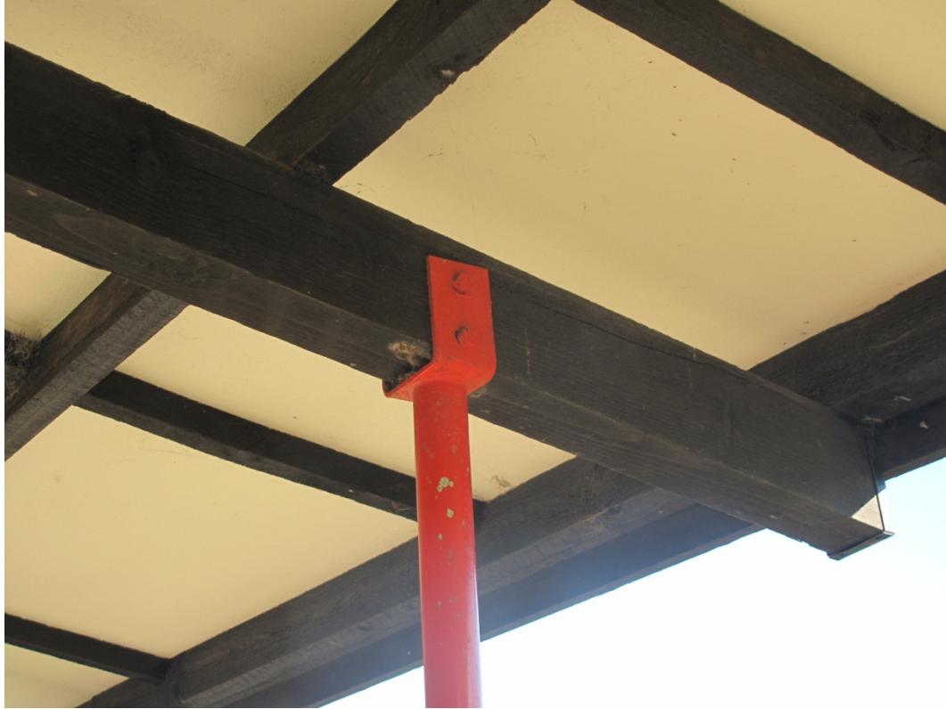
Photograph 7 Connection between the steel support posts and canopy rafter.
