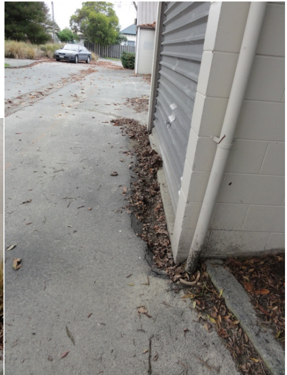
Subsidence in front of Garage Block J
