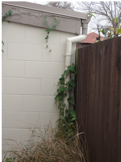
Garage leaning on fence
