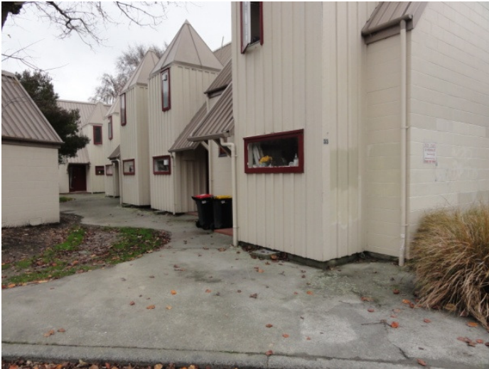
Possible ground heave of asphalt
