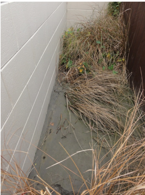
Liquefaction behind garage
