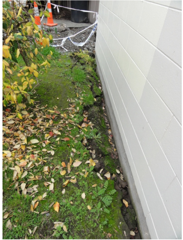
Ground Damage on eastern elevation of Unit 9 33 Vienna
