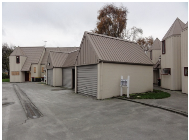
Garage Block H suspected subsidence on north side
