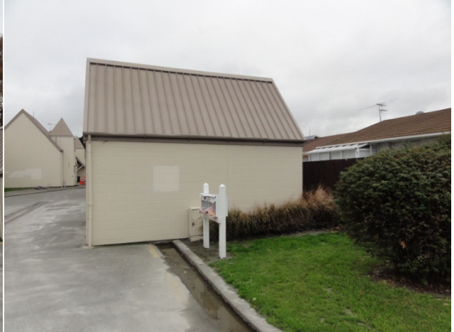
Garage Block G tilting south, up to 150mm settlement.
