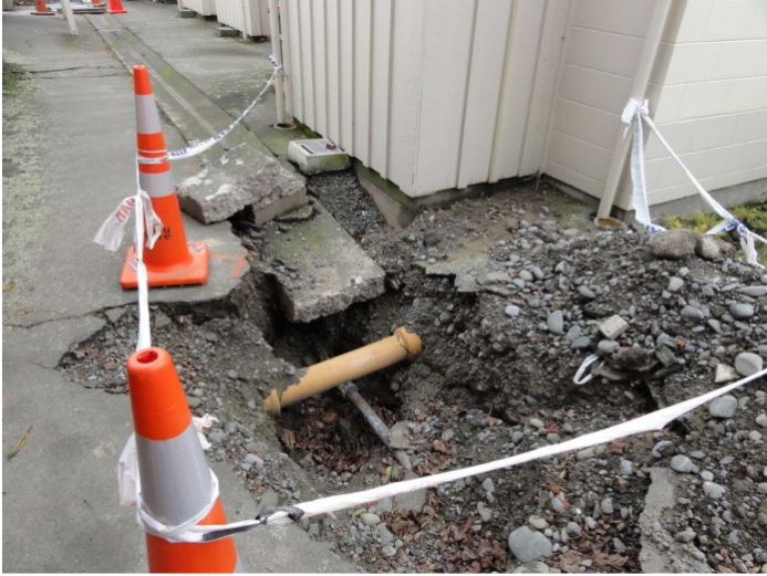
Ground Damage eastern corner of Unit 9 33 Vienna Courts
