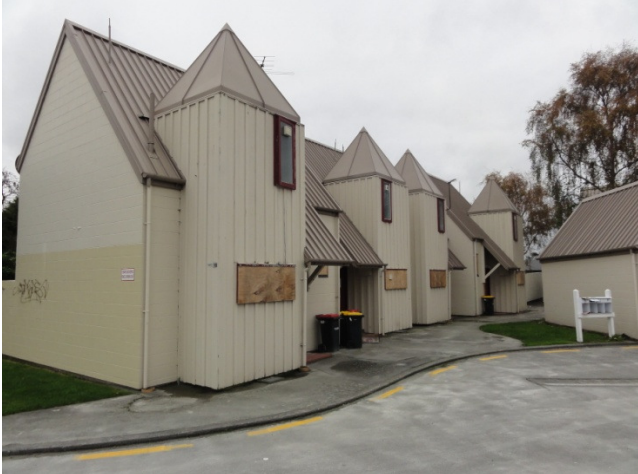
Units 1 – 4 16 Cecil Courts
