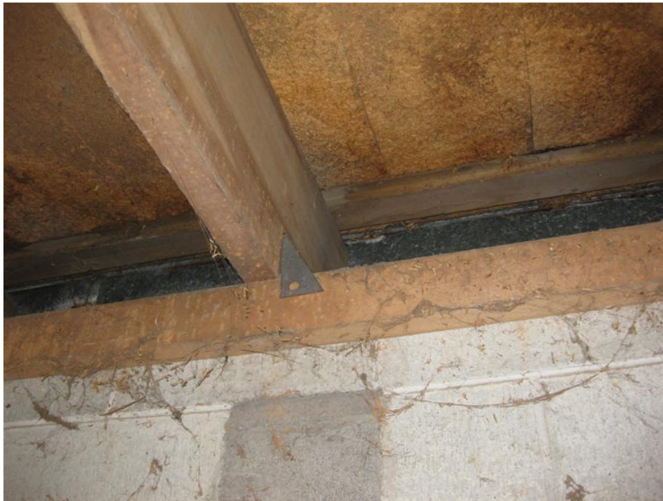
Typical rafter connection with particle board lining over
