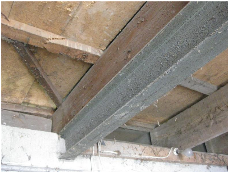
Typical RSJ beam connection to rear wall
