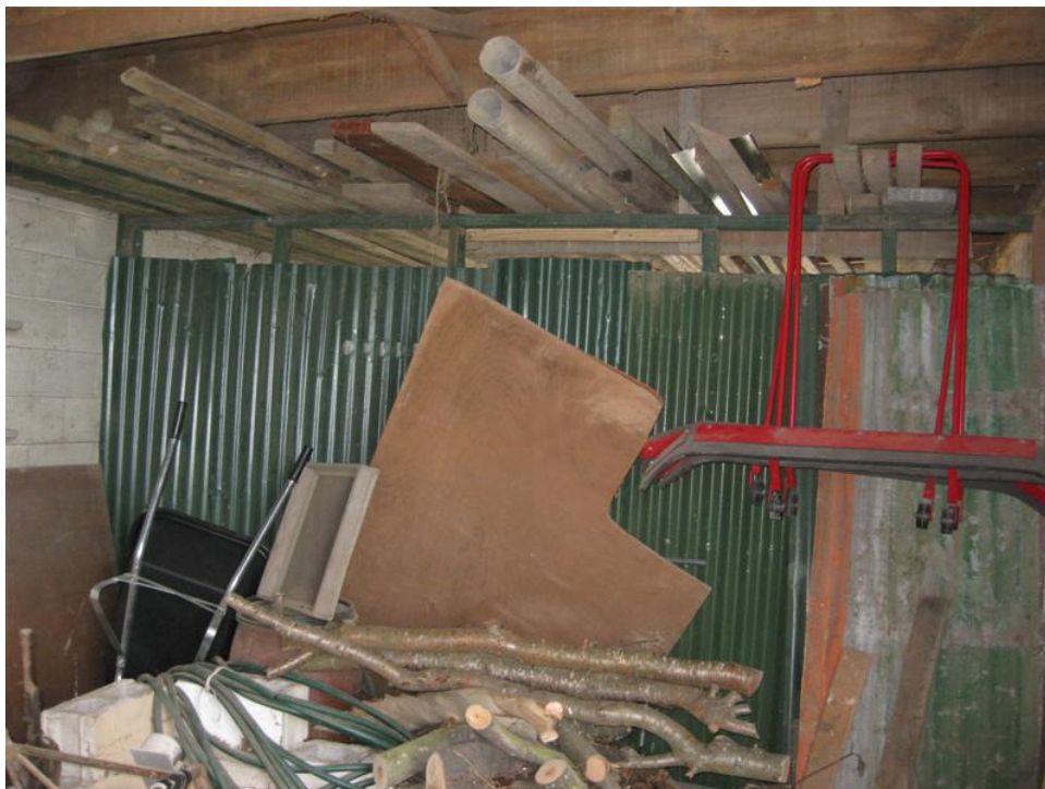
Internal partition wall
