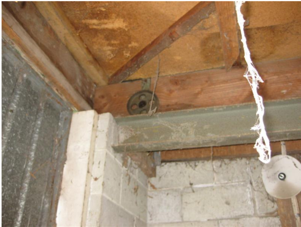
RSJ beams each side of front wall door
