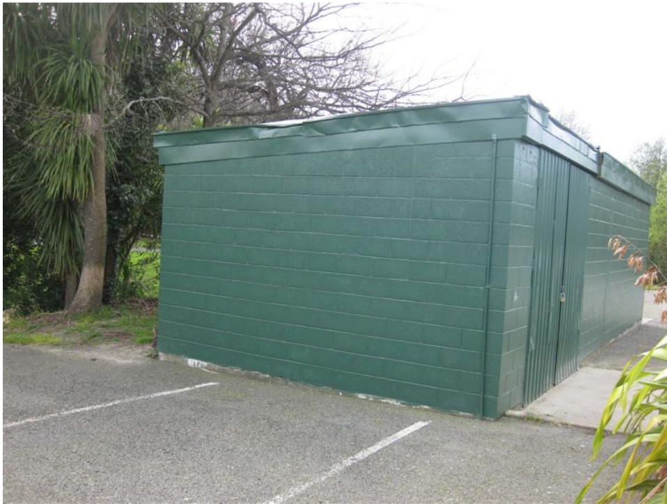
West end (The original door in this wall, has been filled with masonry)
