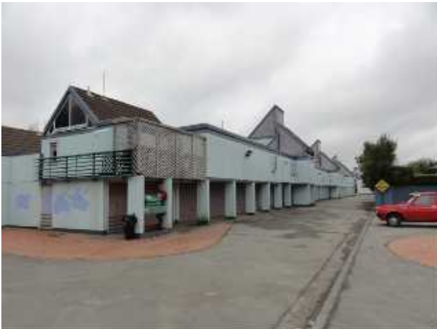
South Elevation of Units 356 – 372
