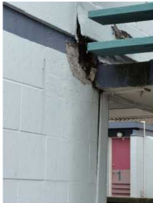
Typical Structural Damage
