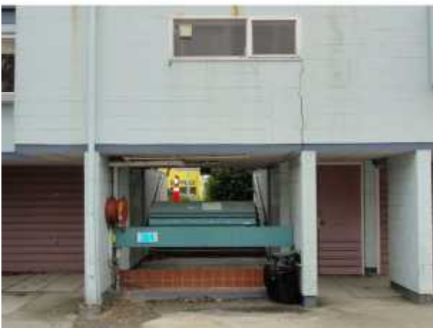
Structural Damage to 2 nd and 3 rd Storey at Unit 364
