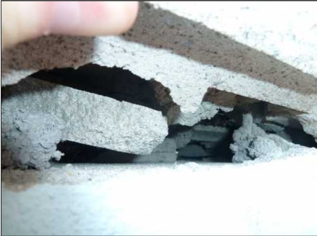
Photo 7: Unfilled concrete masonry void
