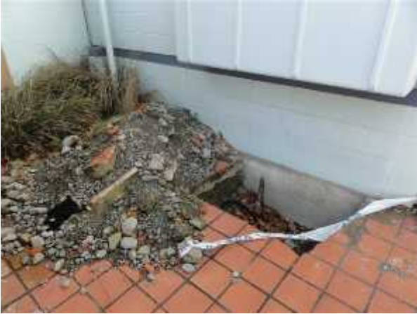
Open excavation showing rounded pit run.
