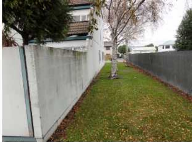
Western limit, no damage visible
