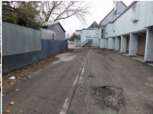
Heave and damage to driveway.
