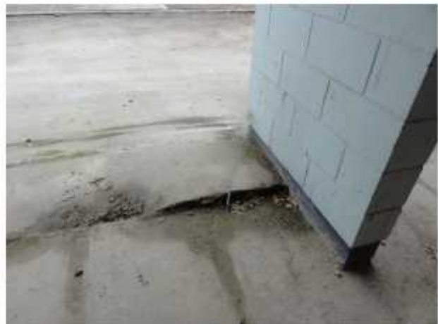
Ground Heave at footing adjacent to Unit 364
