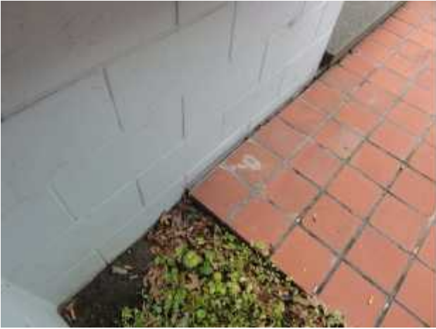
10mm crack, movement towards Brougham Street at Unit 368
