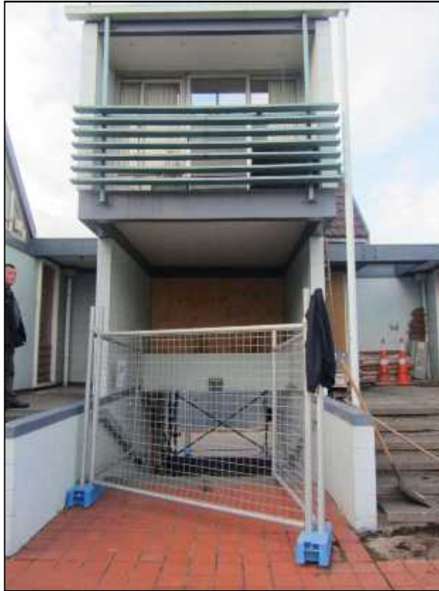
Photo 3: View of a typical 3 storey section of building
