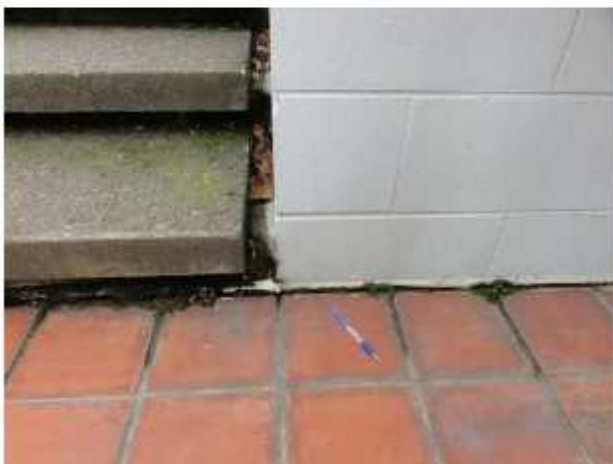
10mm settlement of patio tiles
