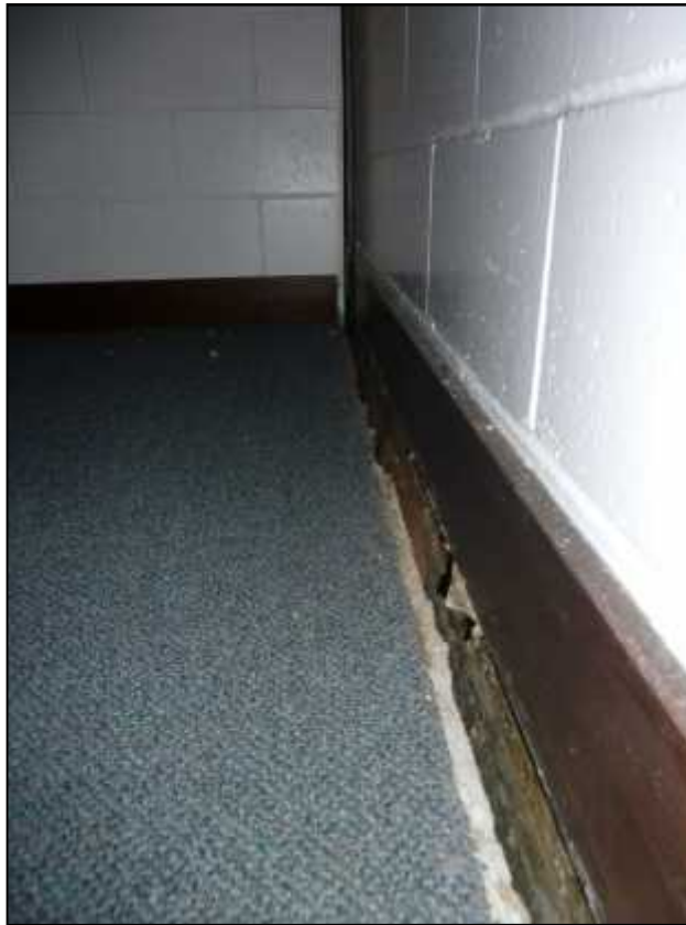
Photo 5: 60mm settlement with 40mm lateral displacement of slab and wall at the interface with adjacent unit
