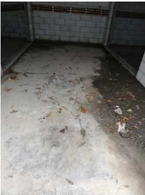
Garage 33 near Unit 388 crack in floor slab and liquefaction
