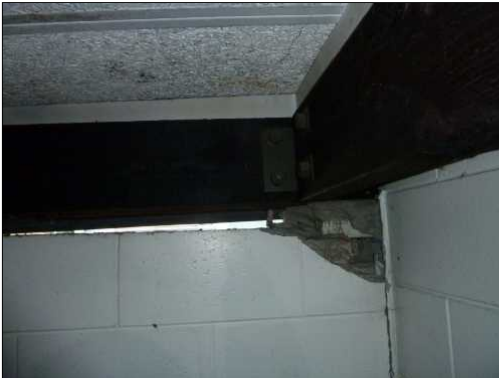
Photo 4: 50mm settlement of a masonry wall 4 at the interface with adjacent unit
