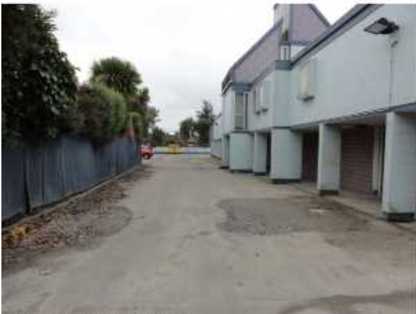
View East, damage to Asphalt
