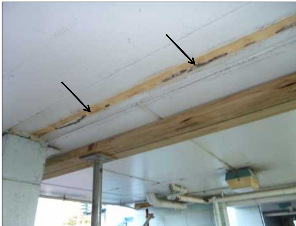
Photo 6: Cracking of suspended slab
