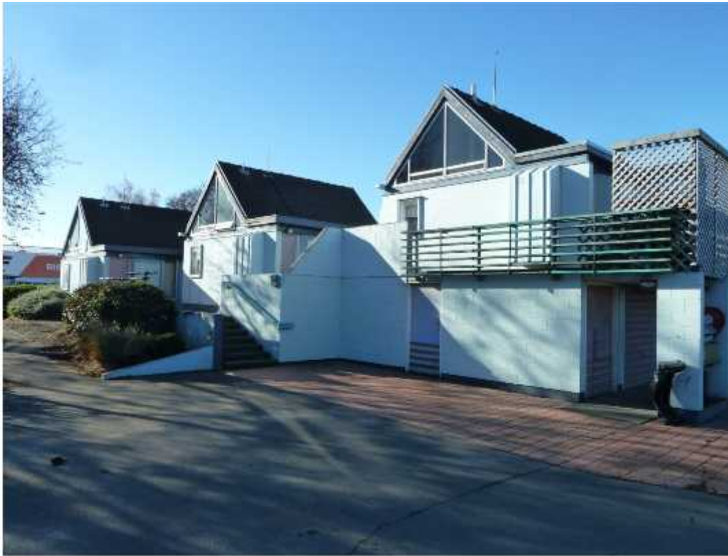
Photo 1: West elevation of block A
