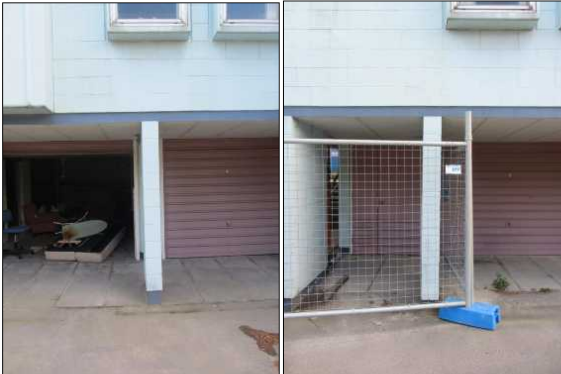
Photo 8 and 9: Masonry piers out of plumb due to differential settlement and lateral spread
