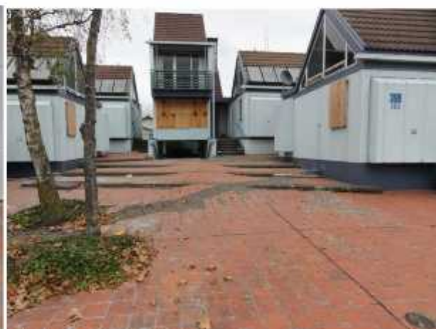
Typical damage to buried services
