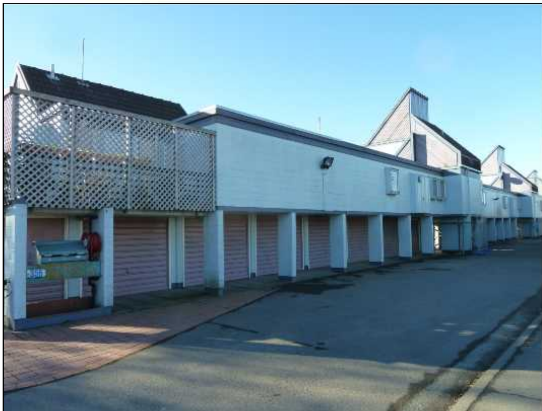
Photo 2: South elevation of block A
