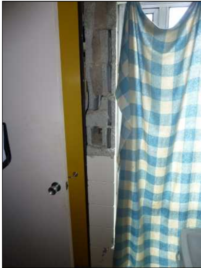
Photo 10: Failure of wall cover concrete due to excess loading
