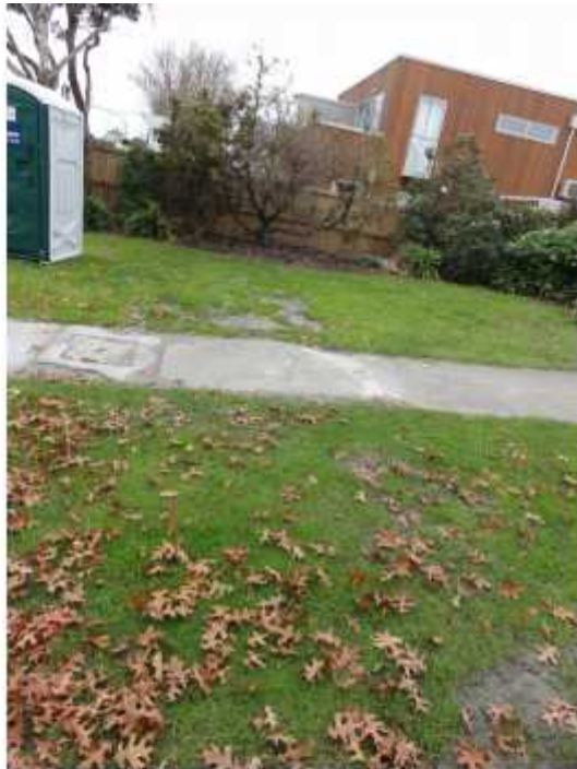
Ground Heave above service trench
