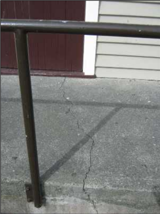
Photograph 5: Cracks in the concrete access ramp
