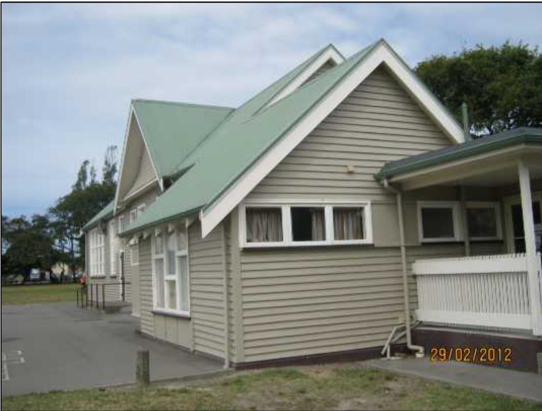
Photograph 1: North west facing corner
