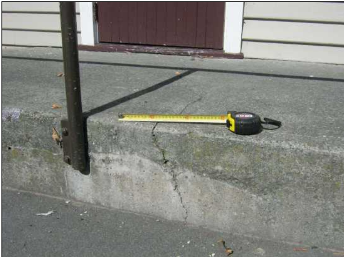
Photograph 12: 2mm wide cracking in rear access ramp (north face).
