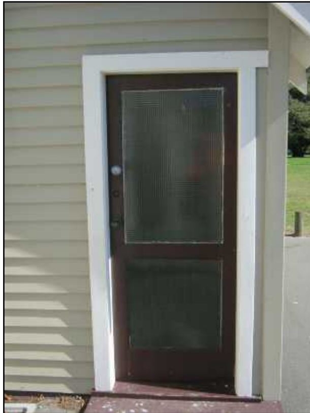
Photograph 9: Rear door way, northwest corner. Minor distortion to door frame.
