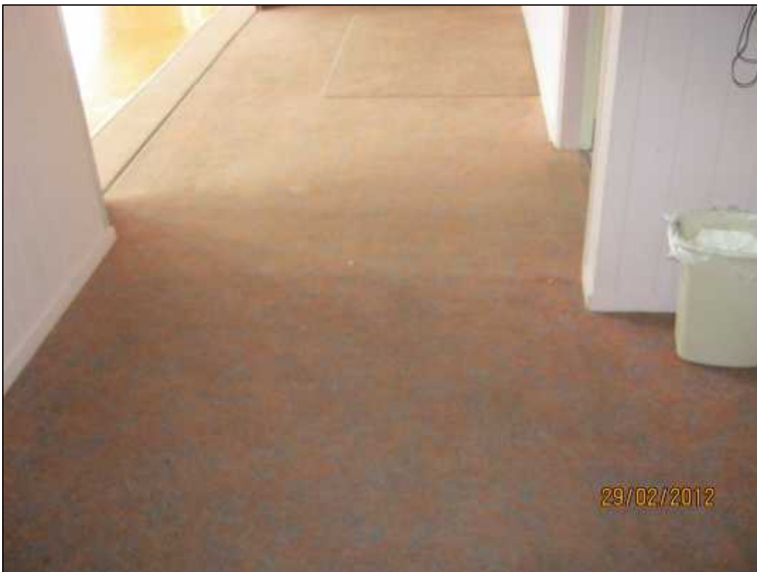
Photograph 4: Floor heaving outside the kitchen
