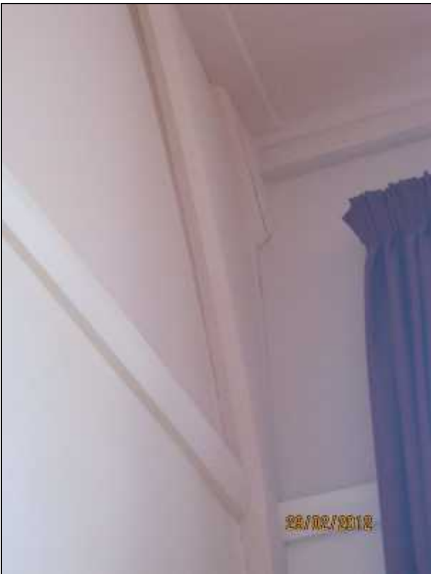
Photograph 6: Cracks in the timber rafter support
