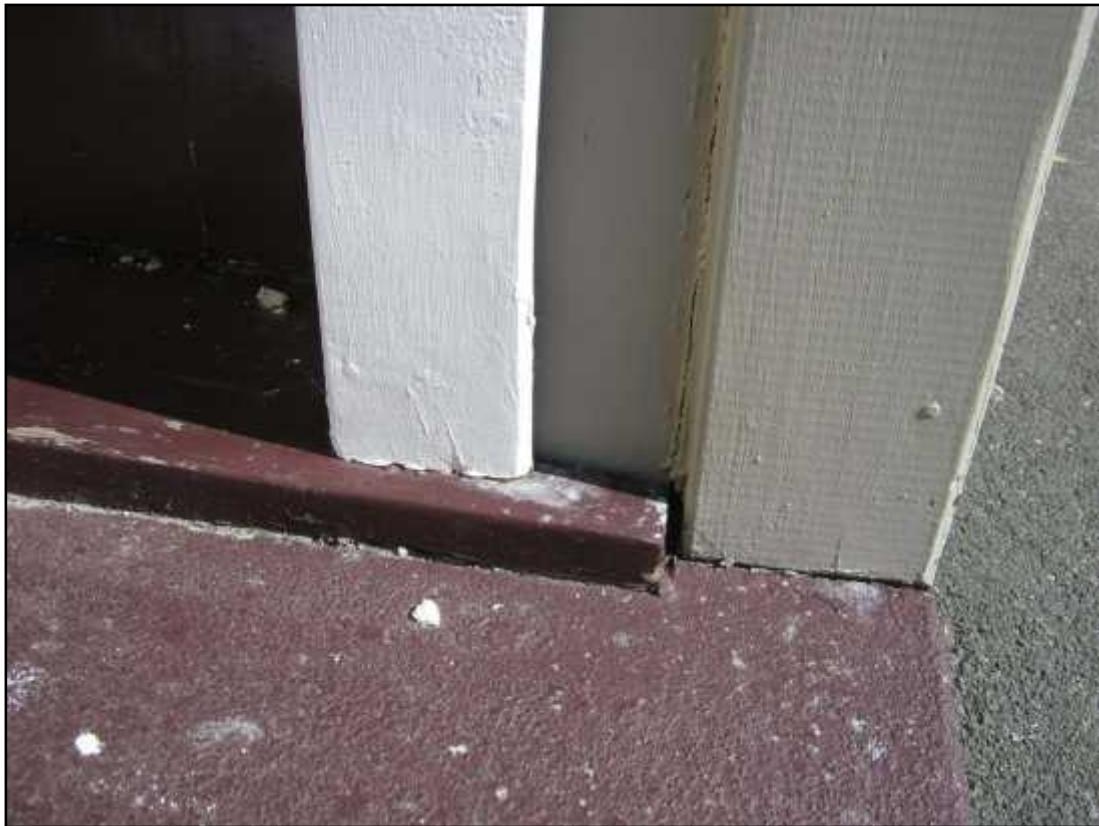
Photograph 10: Separation between rear door step and building frame/facing.
