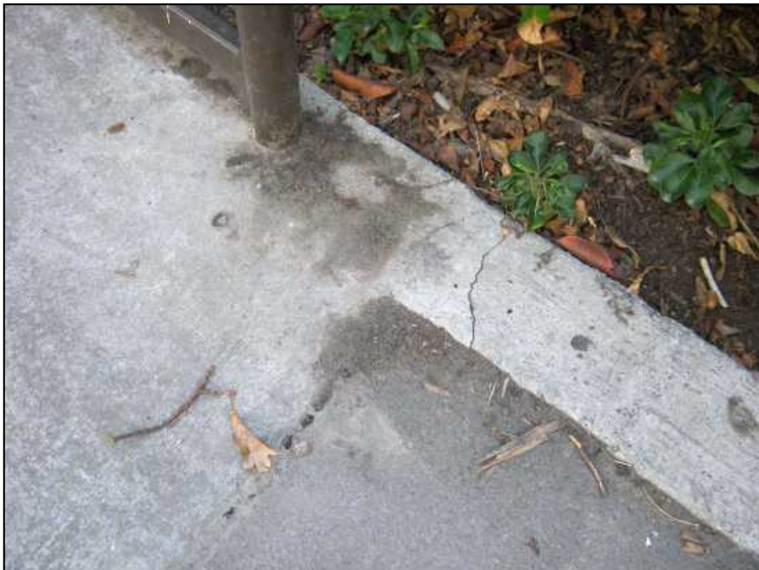
Photograph 16: Cracking in access ramp (south face).
