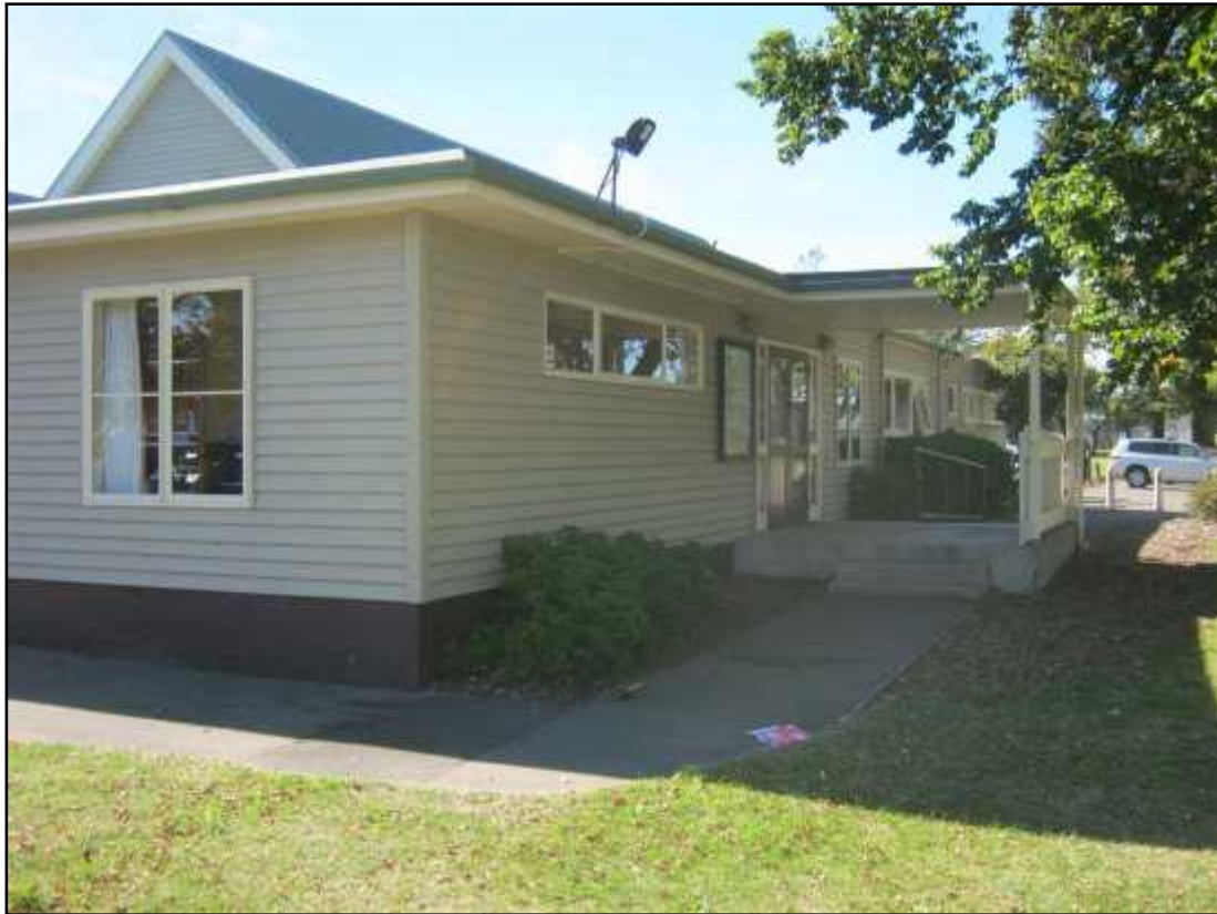
Photograph 1: View of south west corner of Community Centre
