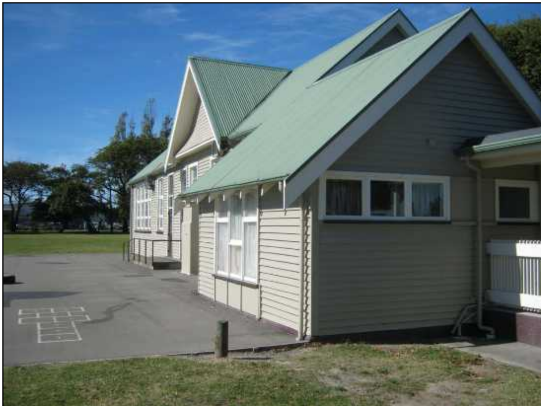
Photograph 2: View of north west corner of Community Centre
