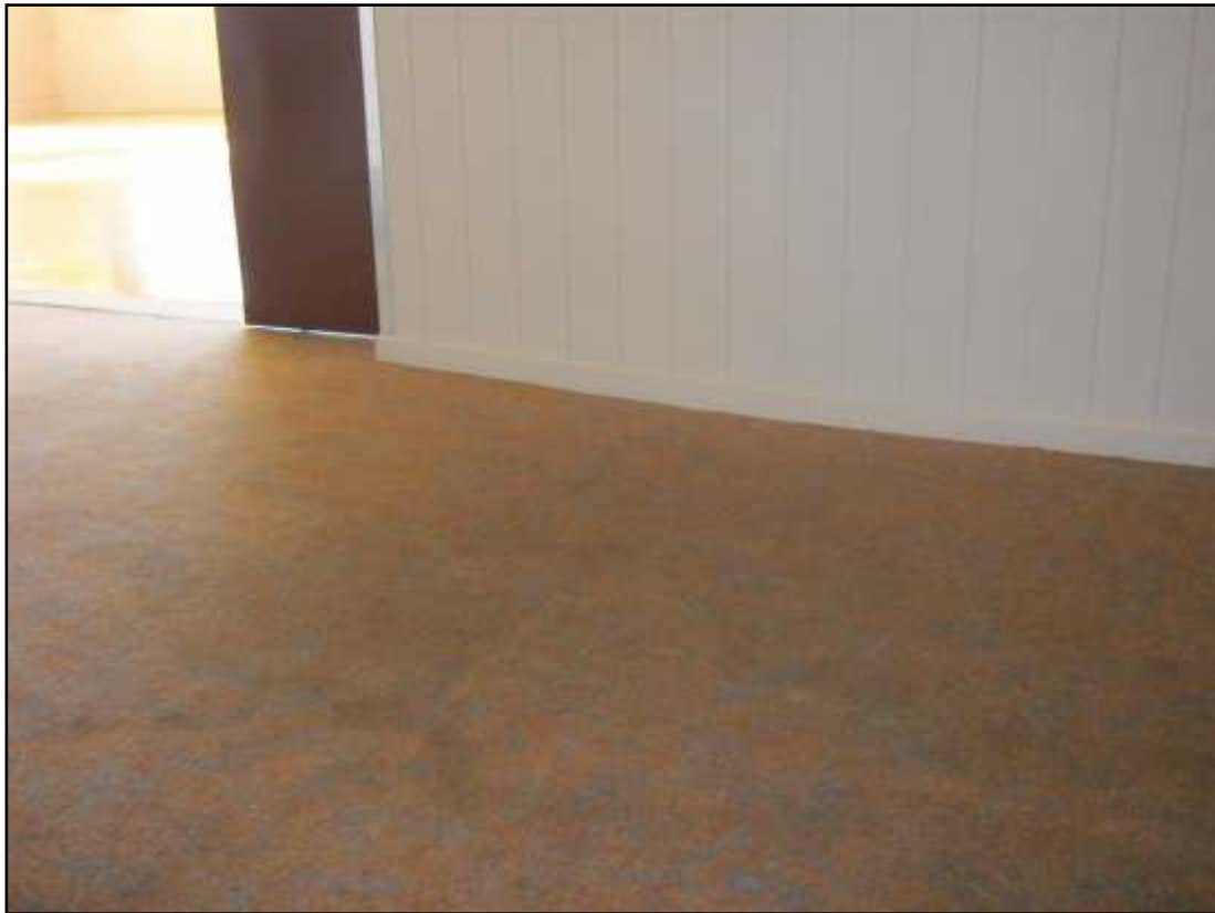
Photograph 6: View of bulging in floor to the front of the kitchen area.
