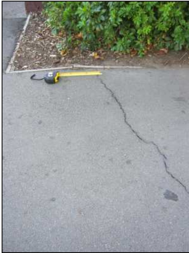
Photograph 7: cracking in footpath, south west corner.
