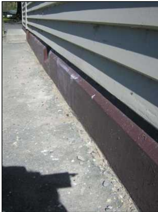
Photograph 14: Up to 50mm separation of asphalt seal away from footings (east face).
