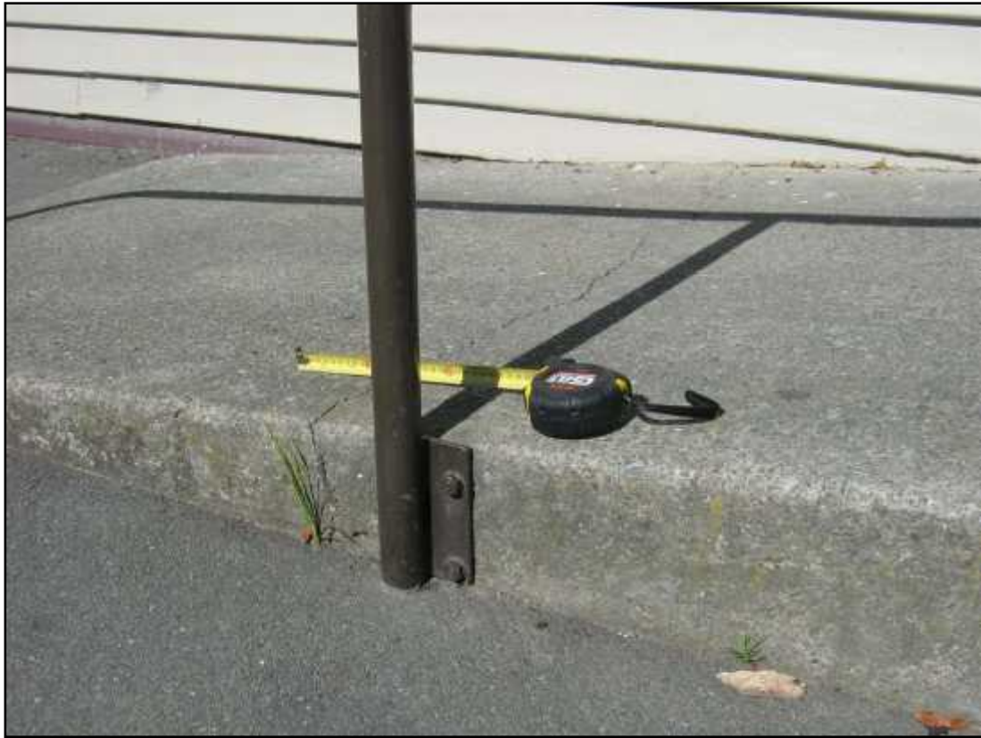
Photograph 13: 2mm wide cracking in rear access ramp (north face).
