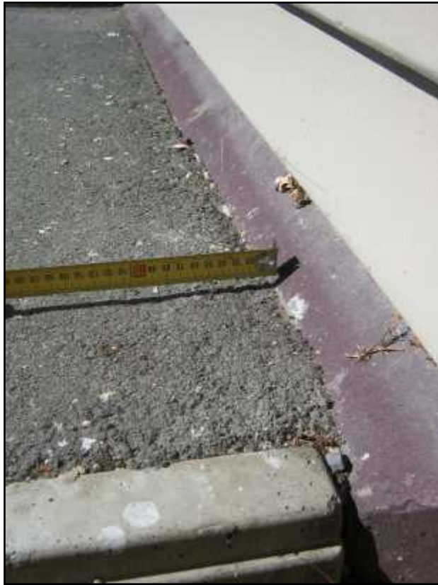
Photograph 11: Possible separation of asphalt seal away from footings (north face).
