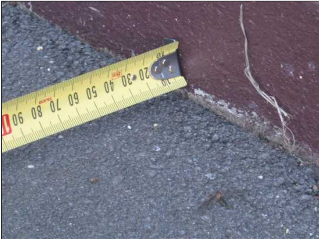
Photograph 15: Possible separation of asphalt seal away from footings (south face).
