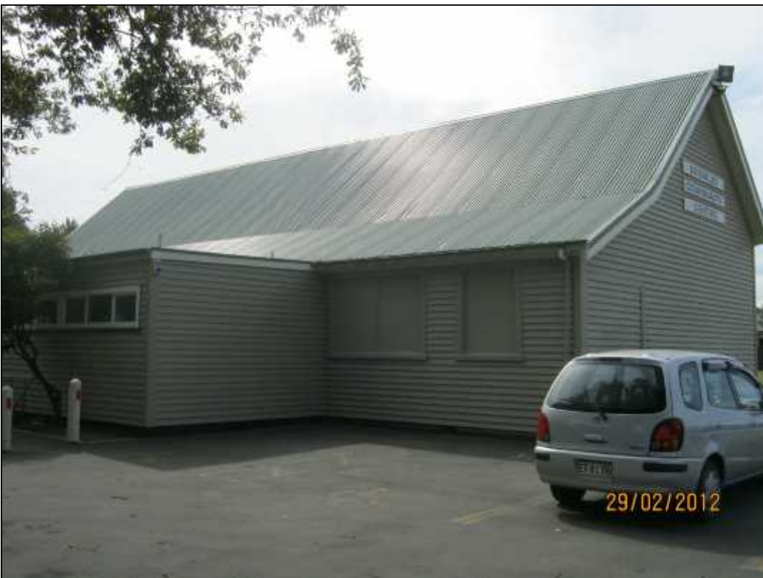
Photograph 2: South east facing corner
