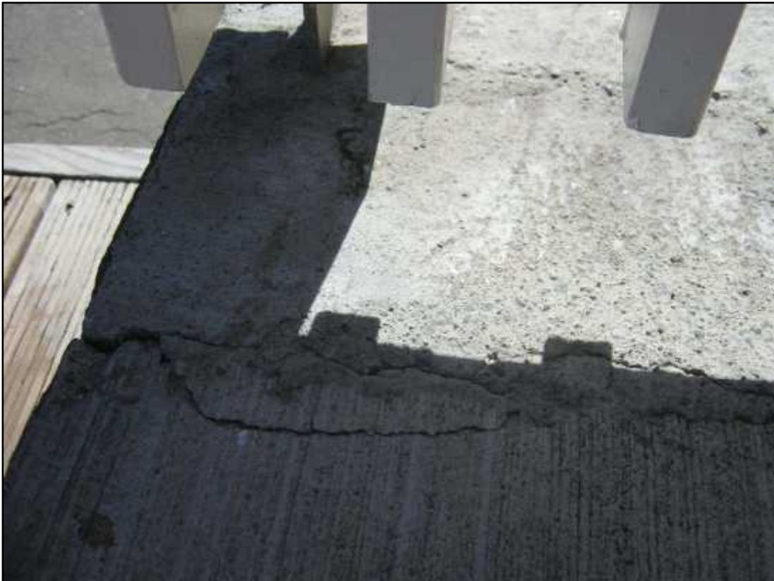
Photograph 8: cracking around support column to porch, northwest corner.
