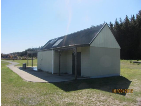
Photo 1: View of Broadhaven Park toilets
