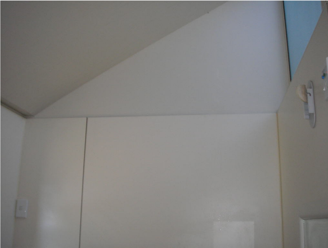
Photo 5: Typical ceiling detail
