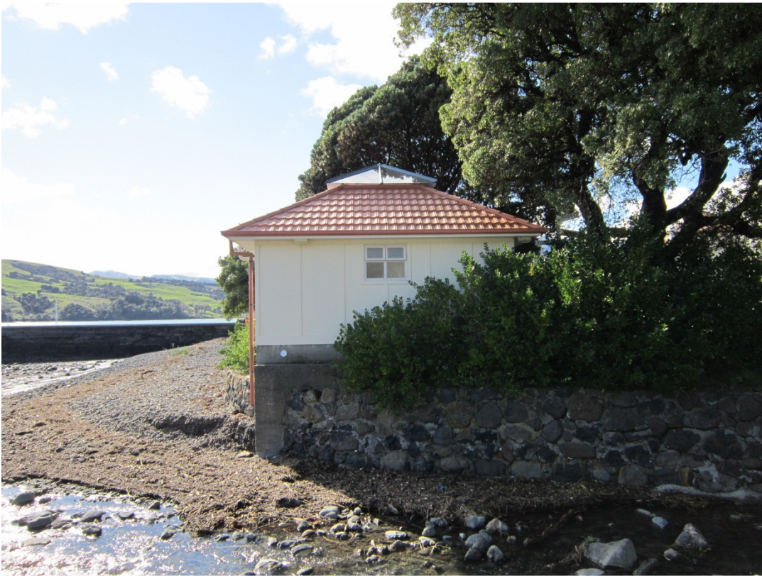
Photo 3: Building side wall
