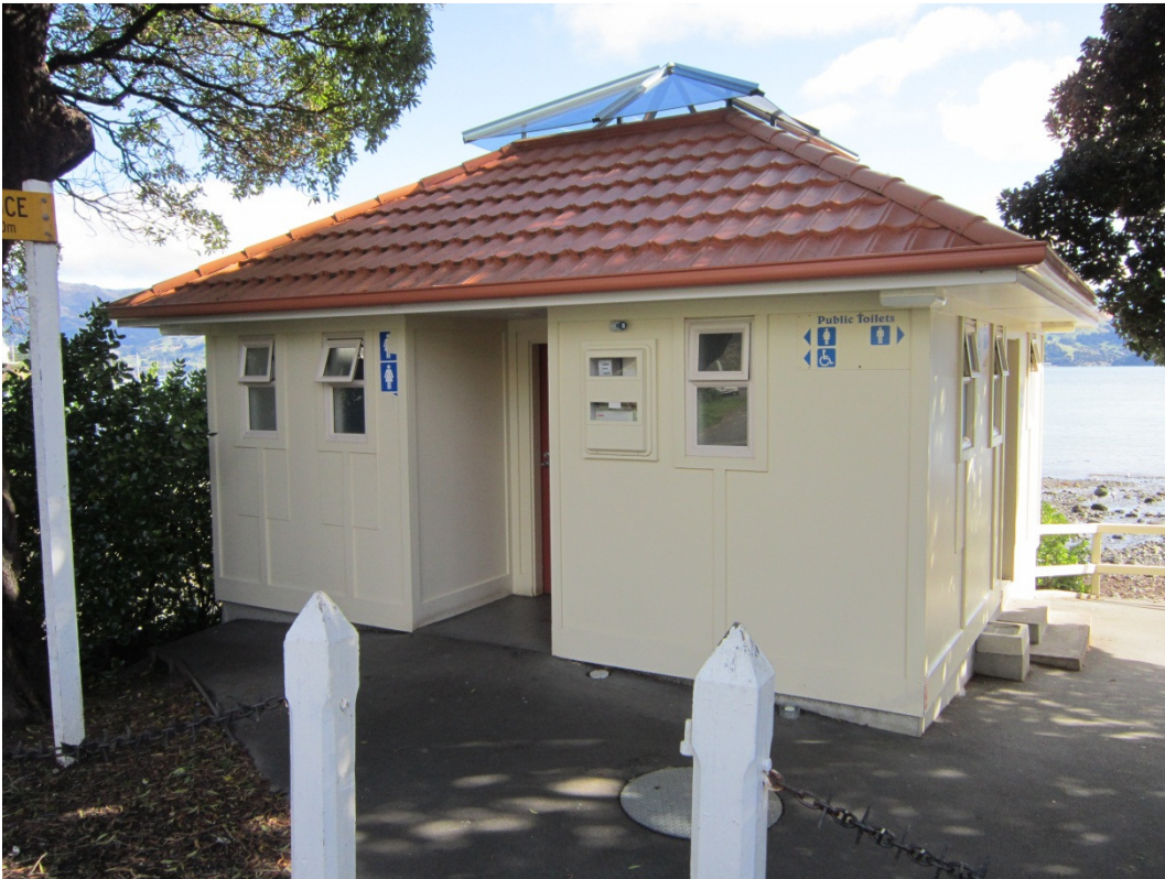
Photo 1: Building frontage and side wall
