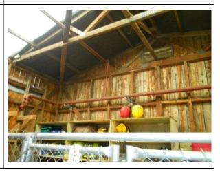
Lateral braces for the timber framed wall and roof trusses
