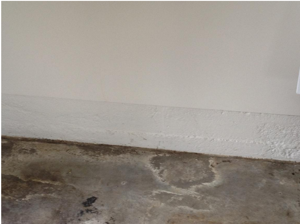
Photograph 4: Perimeter strip footing supporting timber framed wall
