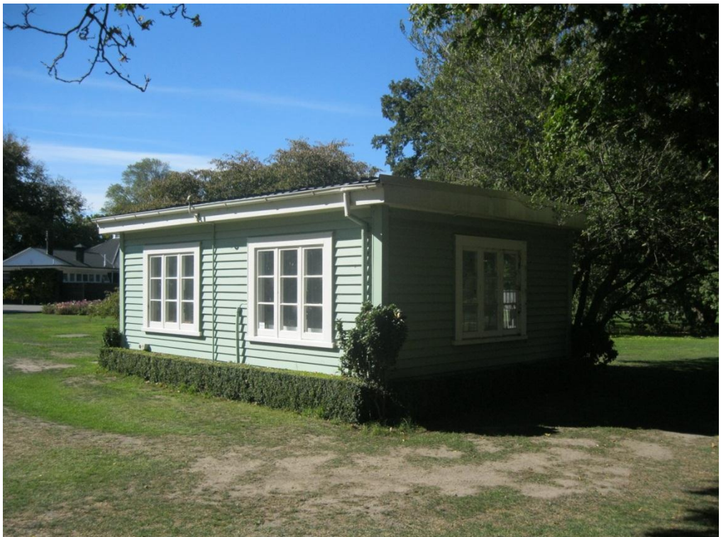
Photograph 2: West and south facing elevation
