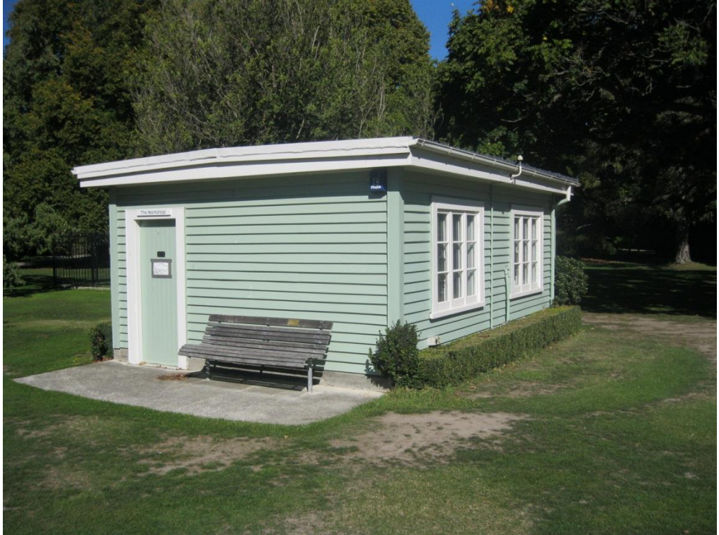
Photograph 1: North and west facing elevation
