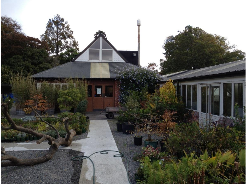
Photograph 1: East facing elevation with link corridor extension on right
