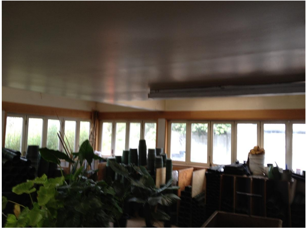
Photograph 5: Boxed out post and beam with windows to south east side of building
