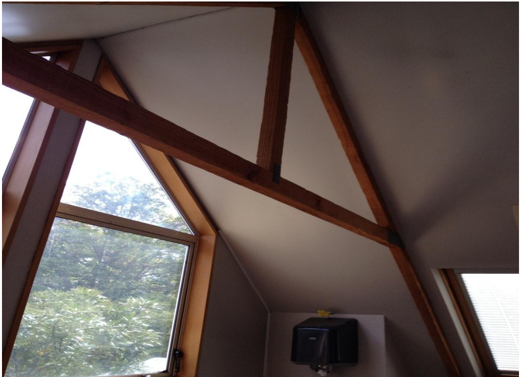
Photograph 8: Timber roof truss to first floor
