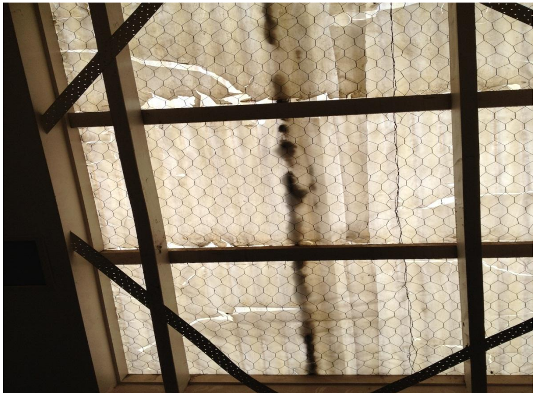
Photograph 6: Extent of roof diagonal strap bracing through skylights
