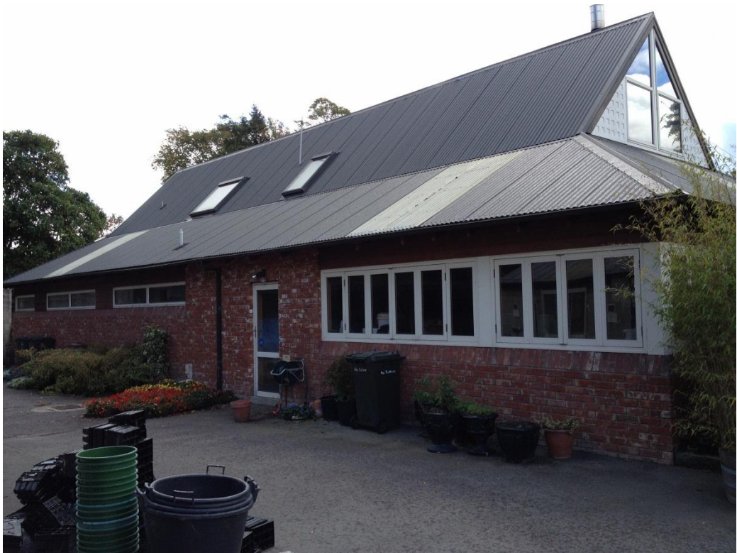
Photograph 2: South elevation showing Dutch hip roof
