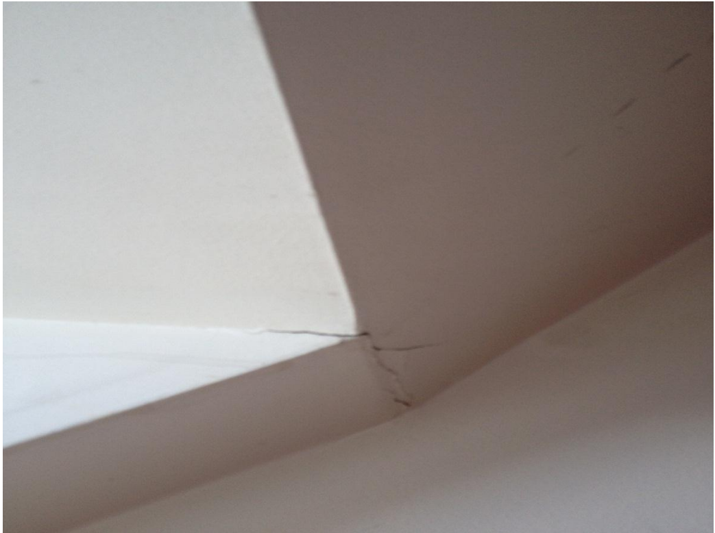
Photograph 7: Minor cracking to plasterboard
