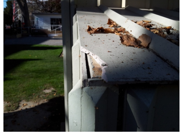
Photo 2: Damage to the external cladding in the north west corner of the pump house lean-to
