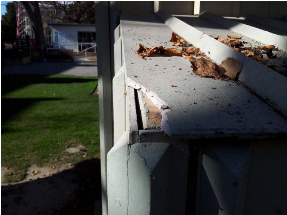
■ Figure 8 - Damage to the roof of the lean-to
