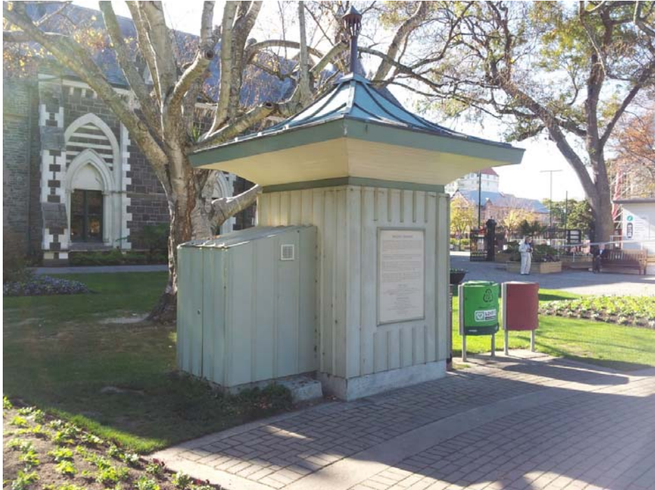
■ Figure 7 - Overview of the pump house
