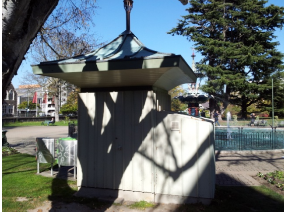
Photo 1: The north elevation of the pump house
